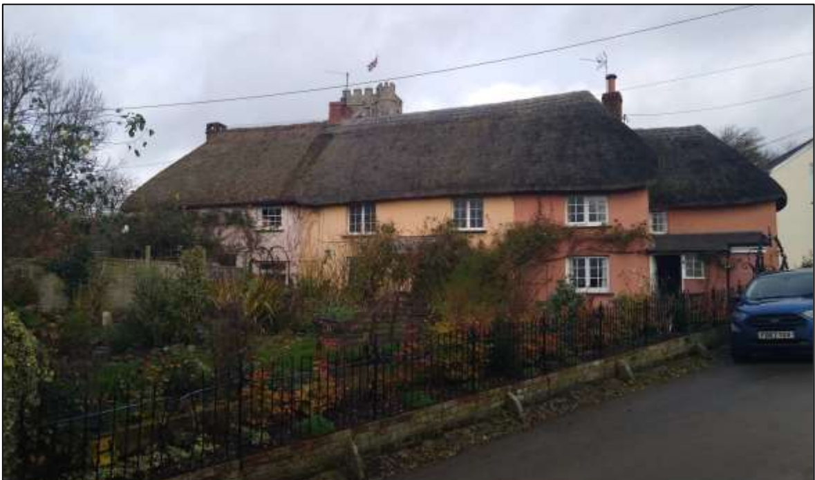
FIGURE 6: THE SOUTH ELEVATION OF THE THREE COTTAGES; VIEWED FROM THE SOUTH.
