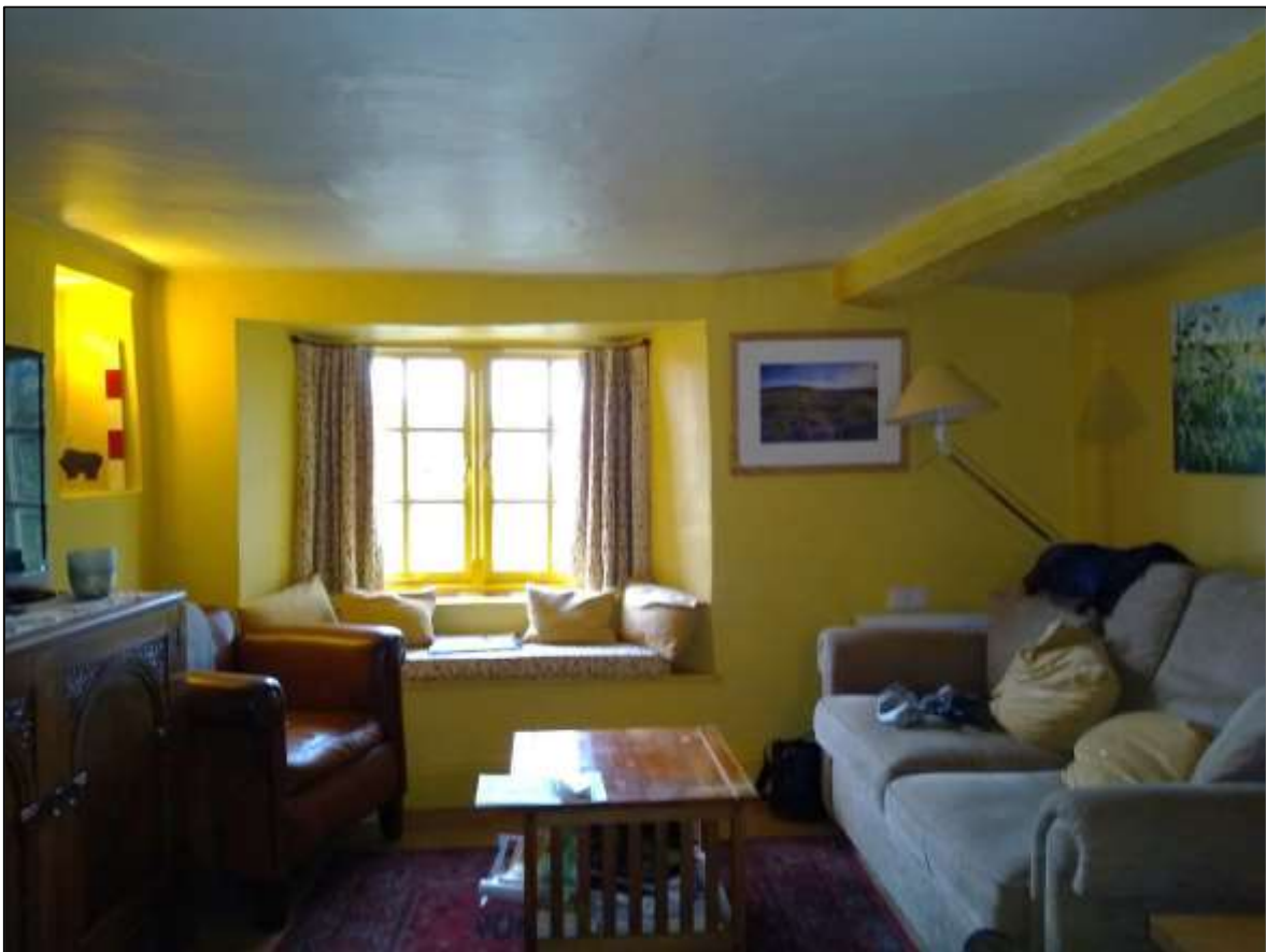
FIGURE 9: CHALLICE GATE COTTAGE: GROUND FLOOR R5 FROM NORTH, WITH C17 CHAMFERED BEAM TO RIGHT AND POSSIBLE C17 SQUINT WINDOW TO LEFT (WITH 50CM SCALE). FRONT WINDOW IS MODERN, IN C17 OPENING.
