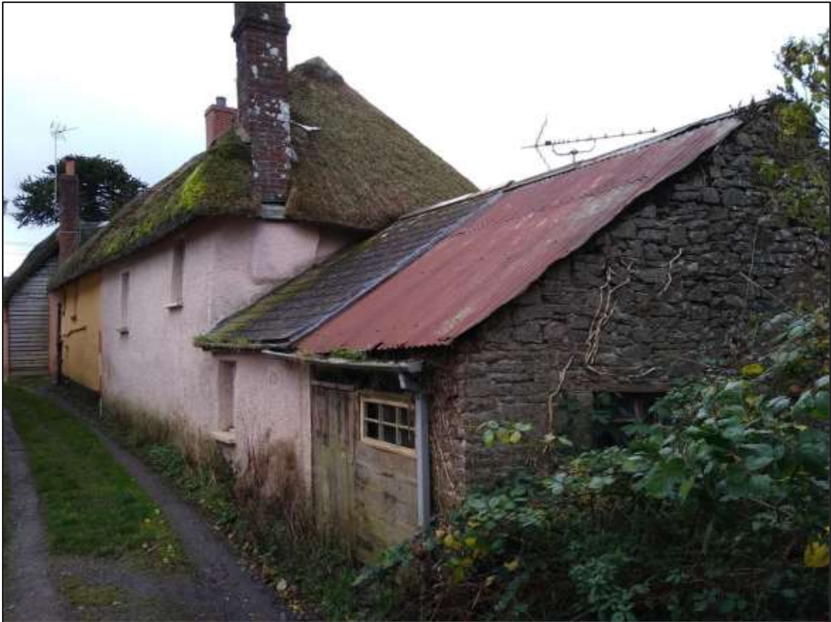
FIGURE 8: THE NORTH ELEVATION OF THE COTTAGES; VIEWED FROM ALONG POORHOUSE LANE TO THE NORTH-WEST.
