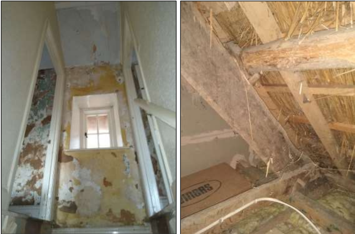
RIGHT: FIGURE 13: HONEY COTTAGE: FIRST FLOOR LANDING R4 LOOKING UP LATER C19 STAIRS FROM SOUTH WITH INSERTED WINDOW OF SAME DATE, CUTTING ACROSS TRACES OF OLDER PARTITION.
