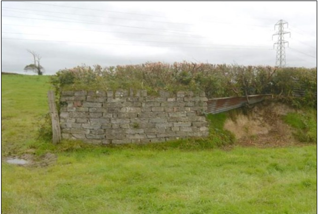
Figure 9: Gateway between Fields 57 and 58 constructed of reused concrete block quoins.
