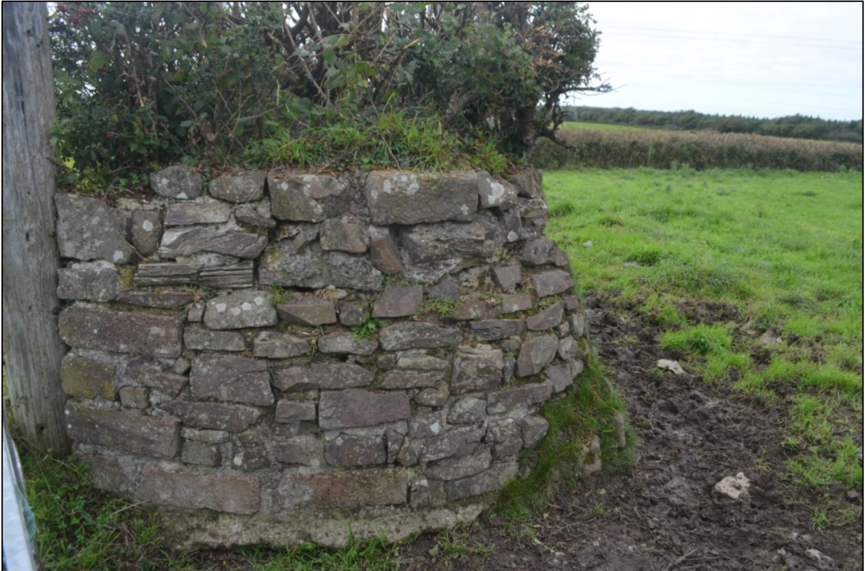
Figure 10: Stone quoin gateway at entrance to Field 59.
