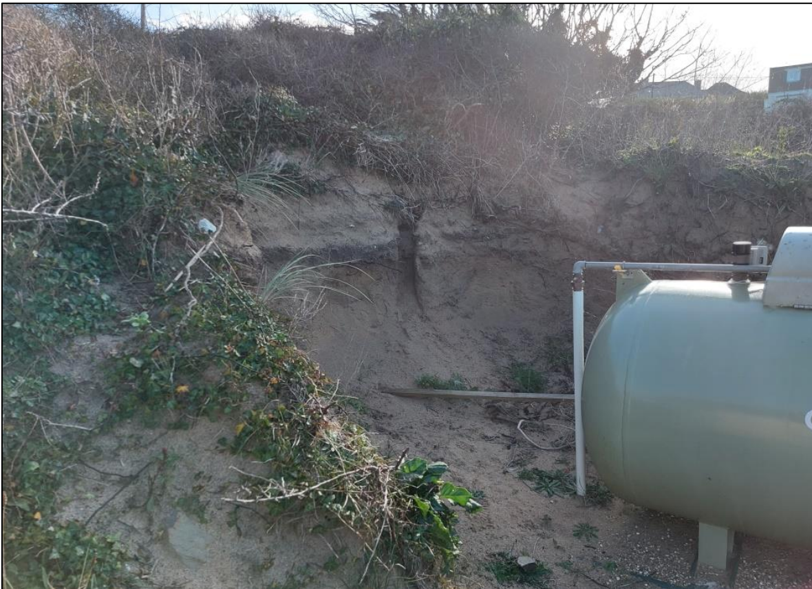
FIGURE 9: ADJACENT OIL TANK, TERRACED INTO THE SAND BANK AT THE BACK (EAST) OF THE EXISTING GARAGE. VIEWED FROM THE NORTH WEST.
