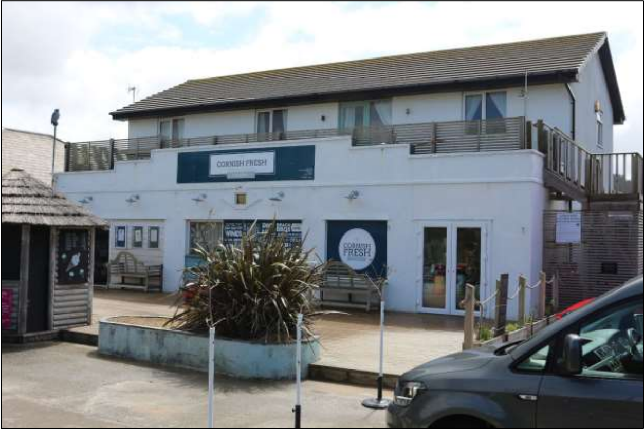
14. BUILDING 1, VIEWED FROM THE WEST.
