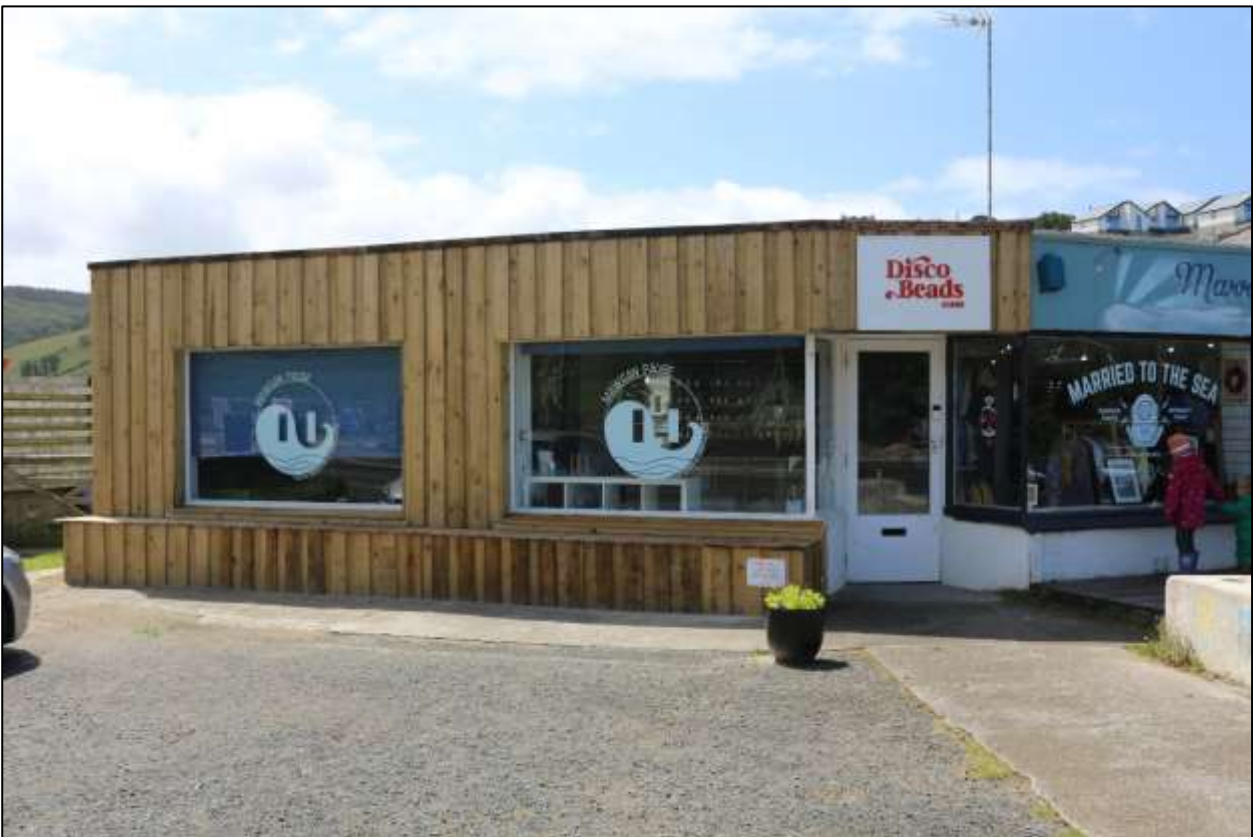
8. BUILDING 3, FROM THE NORTH.
