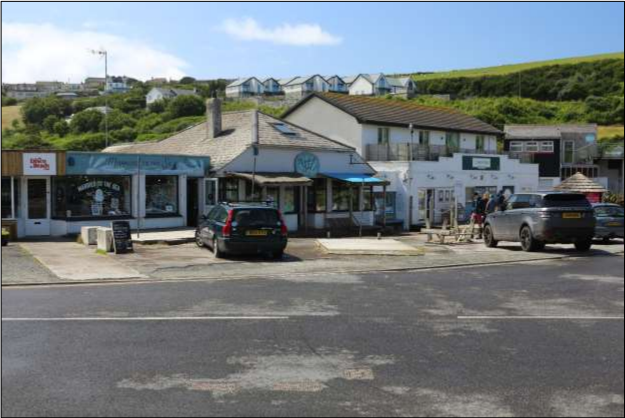
5. THE SITE VIEWED FROM THE NORTH.
