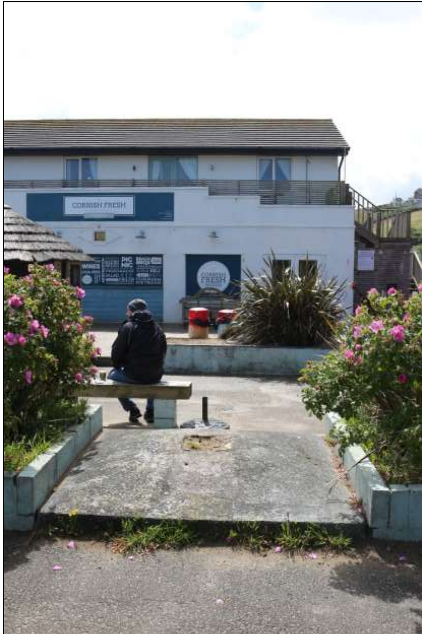
13. BUILDING 1, VIEWED FROM THE NORTH-WEST.
