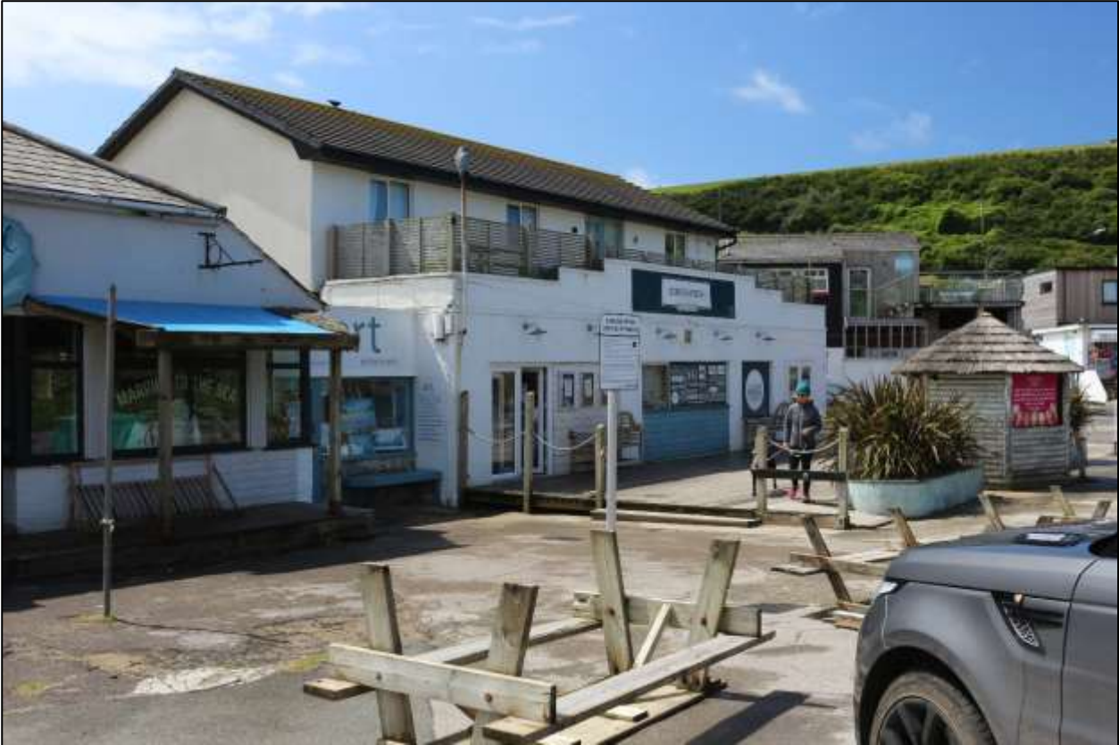
11. BUILDING 1, VIEWED FROM THE NORTH.
