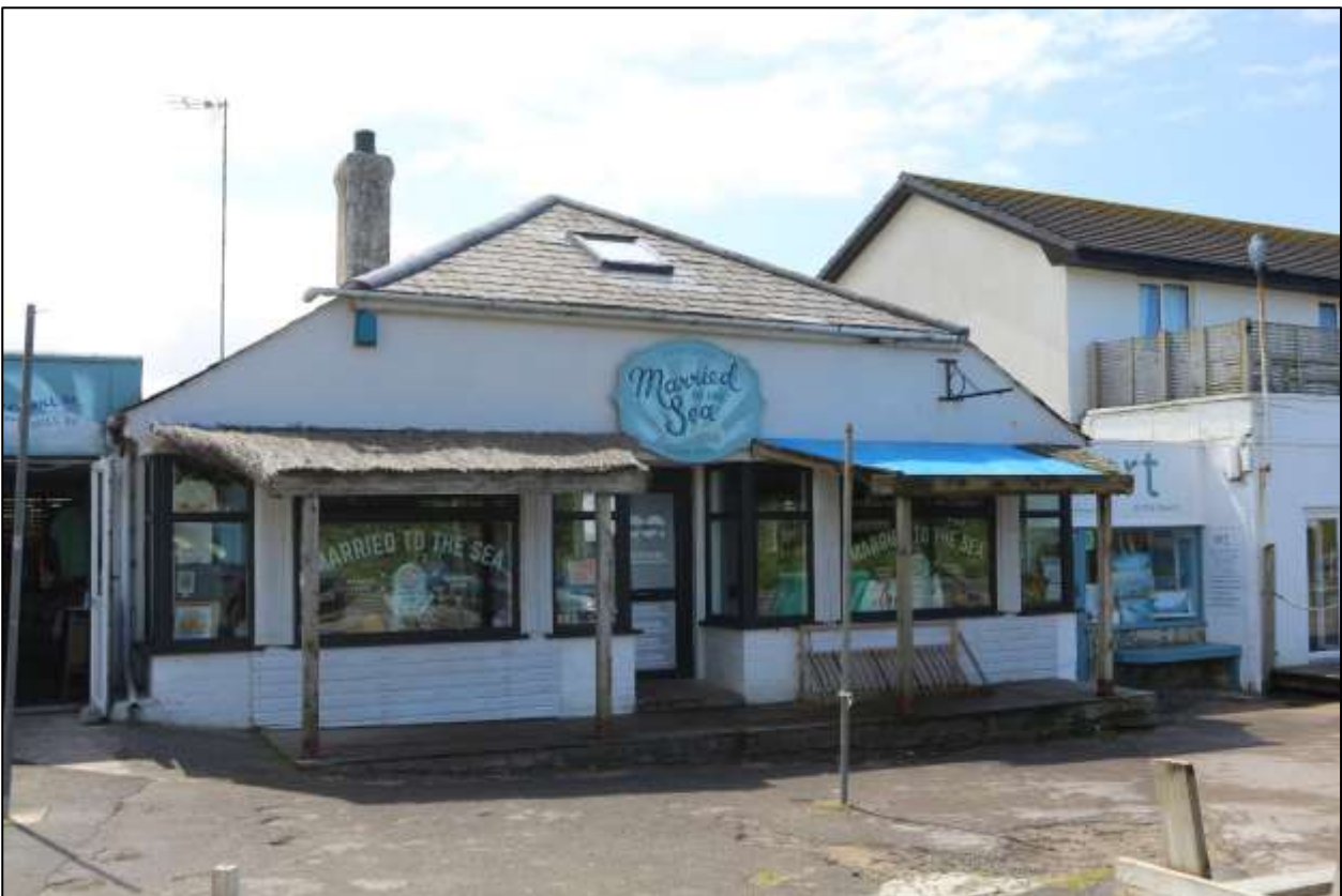
10. BUILDING 2, VIEWED FROM THE WEST.
