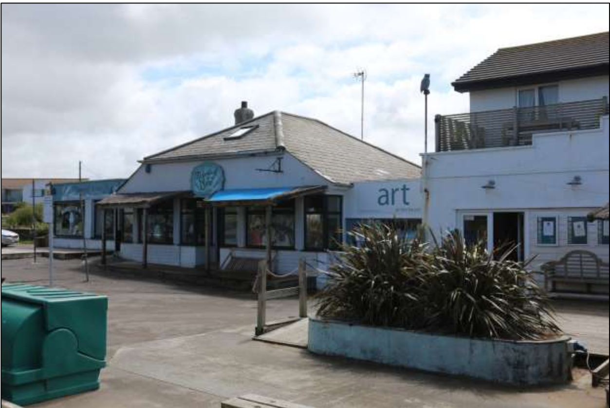
12. BUILDING 2, VIEWED FROM THE WEST.
