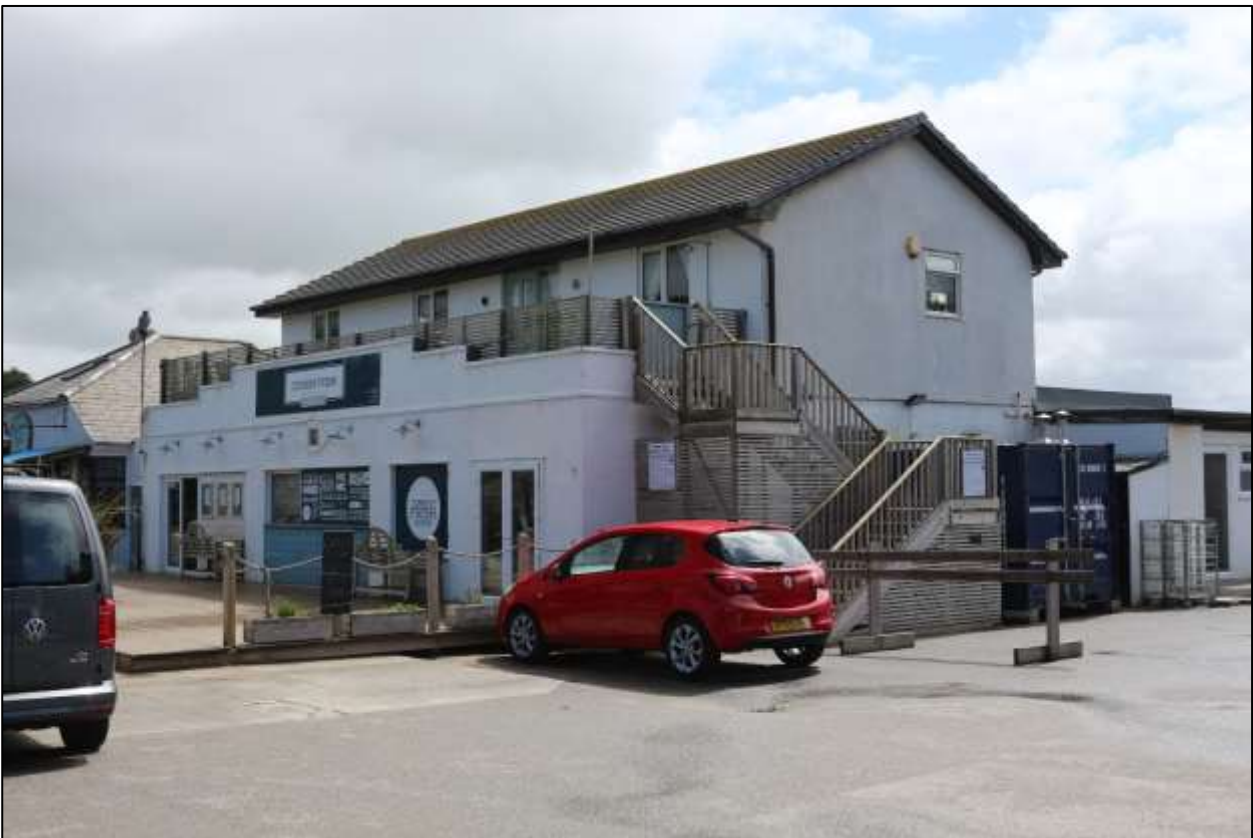
15. BUILDING 1, VIEWED FROM THE WEST.
