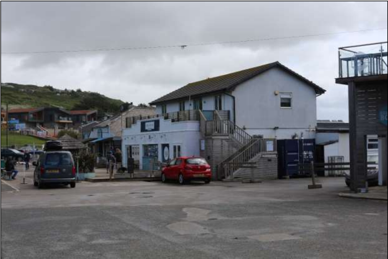
16. BUILDING 1, VIEWED FROM THE WEST, WITH MARVER CHALETs IN THE BACKGROUND.
