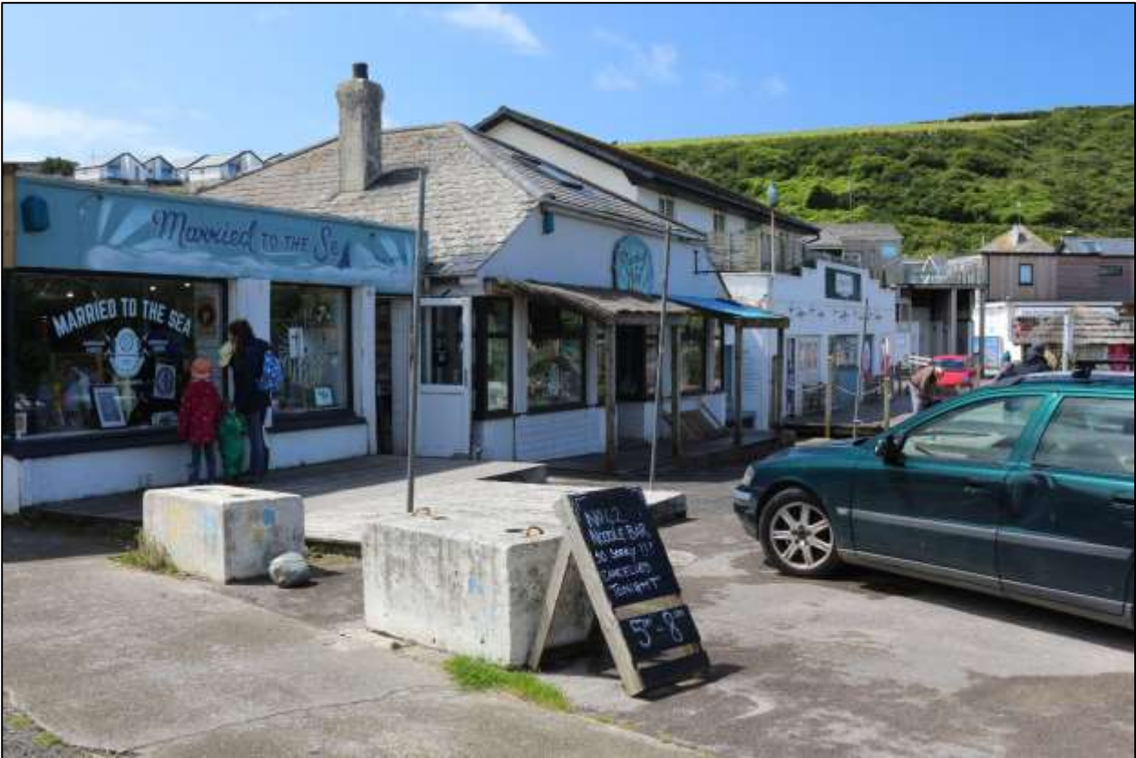
9. BUILDINGS 3-2, VIEWED FROM THE NORTH.
