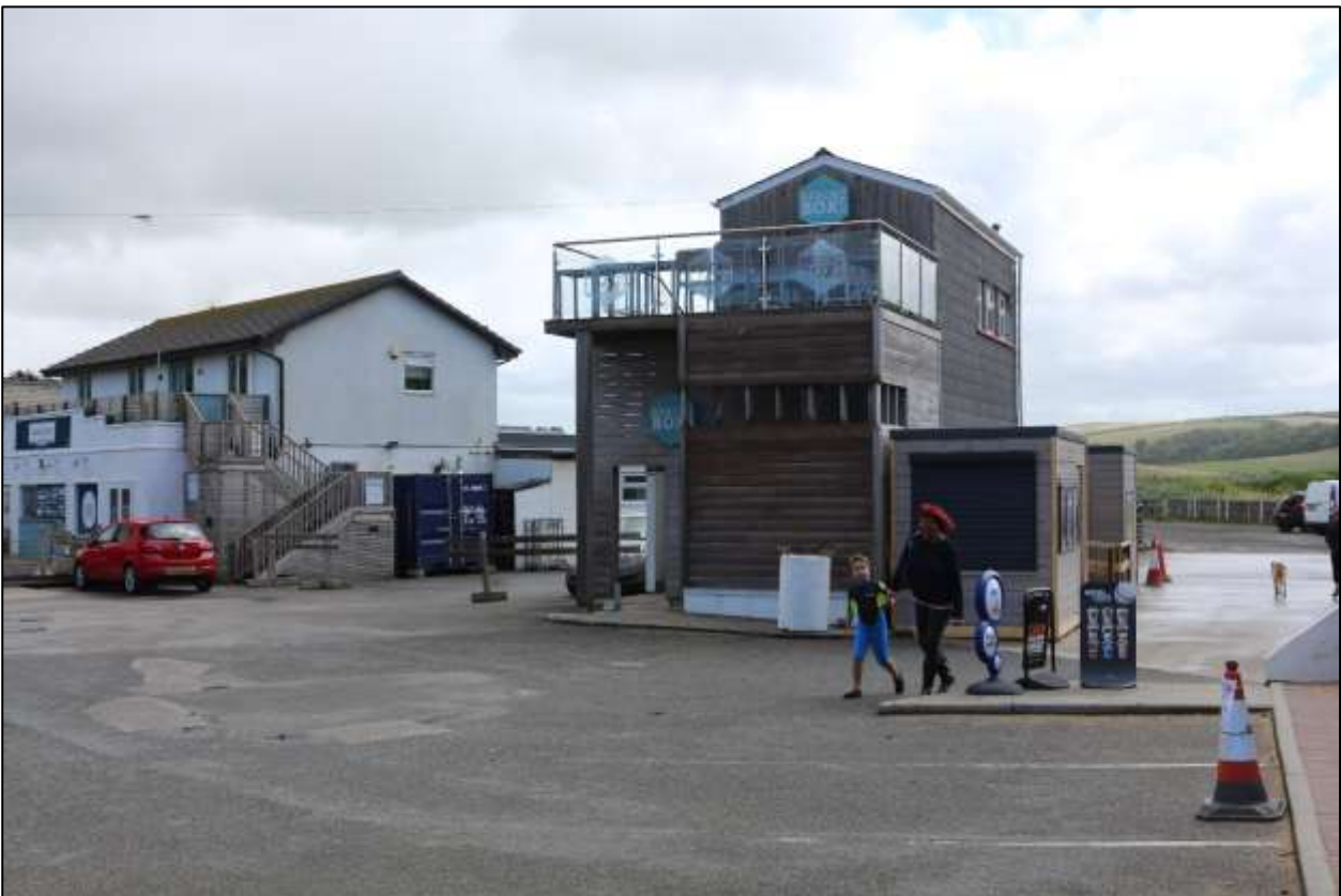
17. BUILDING 4, VIEWED FROM THE WEST.
