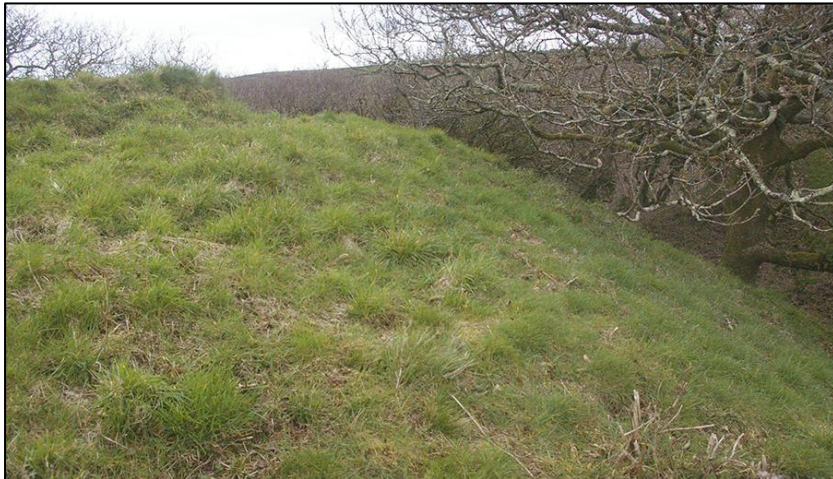
5. THE SLOPE ON THE EAST SIDE OF THE MOTTE; VIEWED FROM THE SOUTH (NO SCALE).
