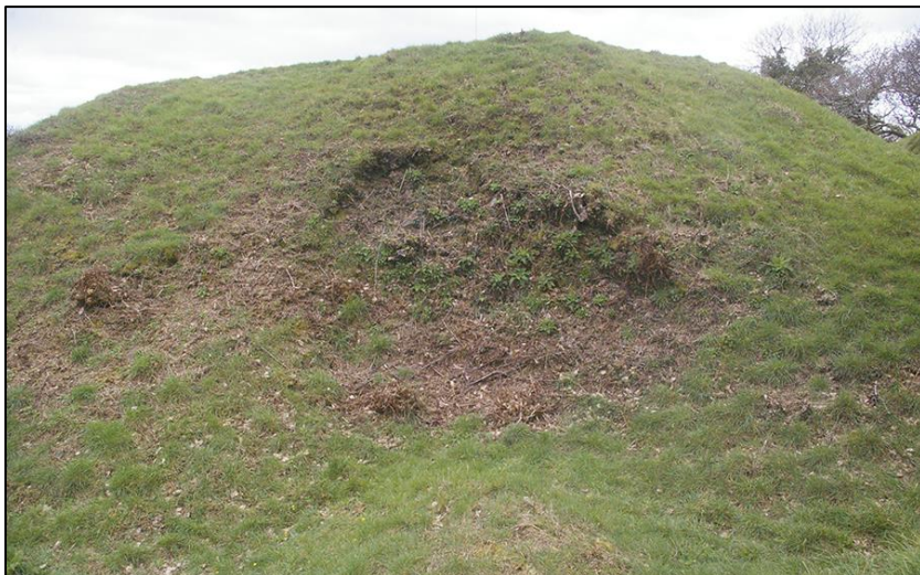
24. EROSION/COLLAPSE IN THE EAST BANK TO THE INNER BAILEY; VIEWED FROM THE EAST (NO SCALE).
