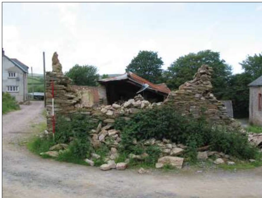
Plate 6 View of exterior of south wall.
