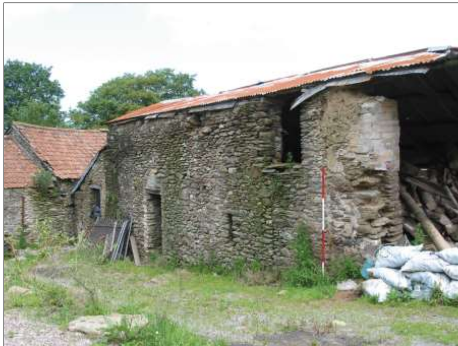
Plate 8 View of west wall of barn.
