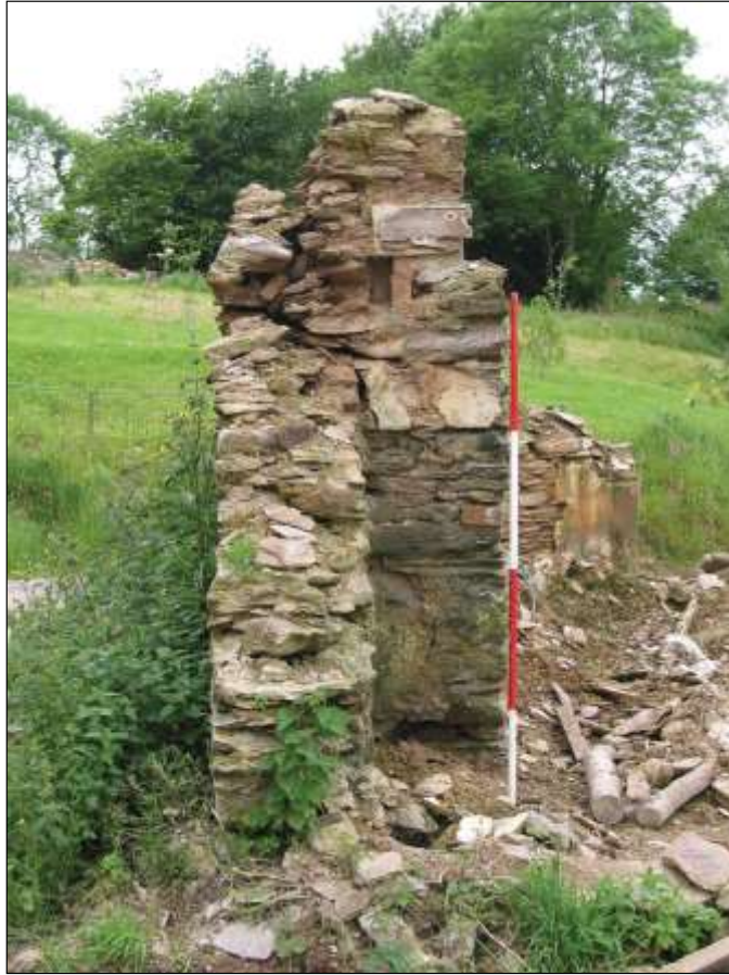
Plate 5 View of chimney stack in south wall. Note skirting board at first floor level.
