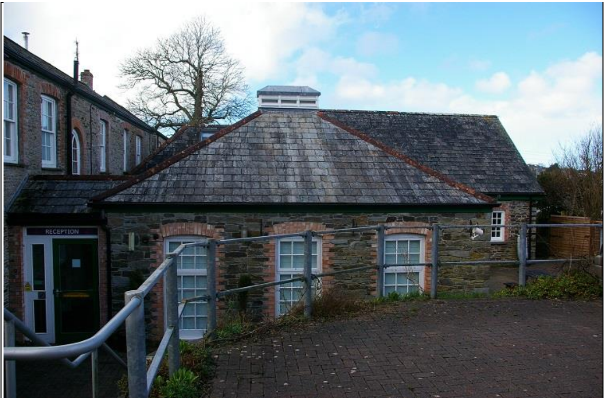
4. MODERN BLOCK 2, BEHIND THE MAIN HOUSE, A PURPOSE-BUILT DINING ROOM; FROM THE EAST.
