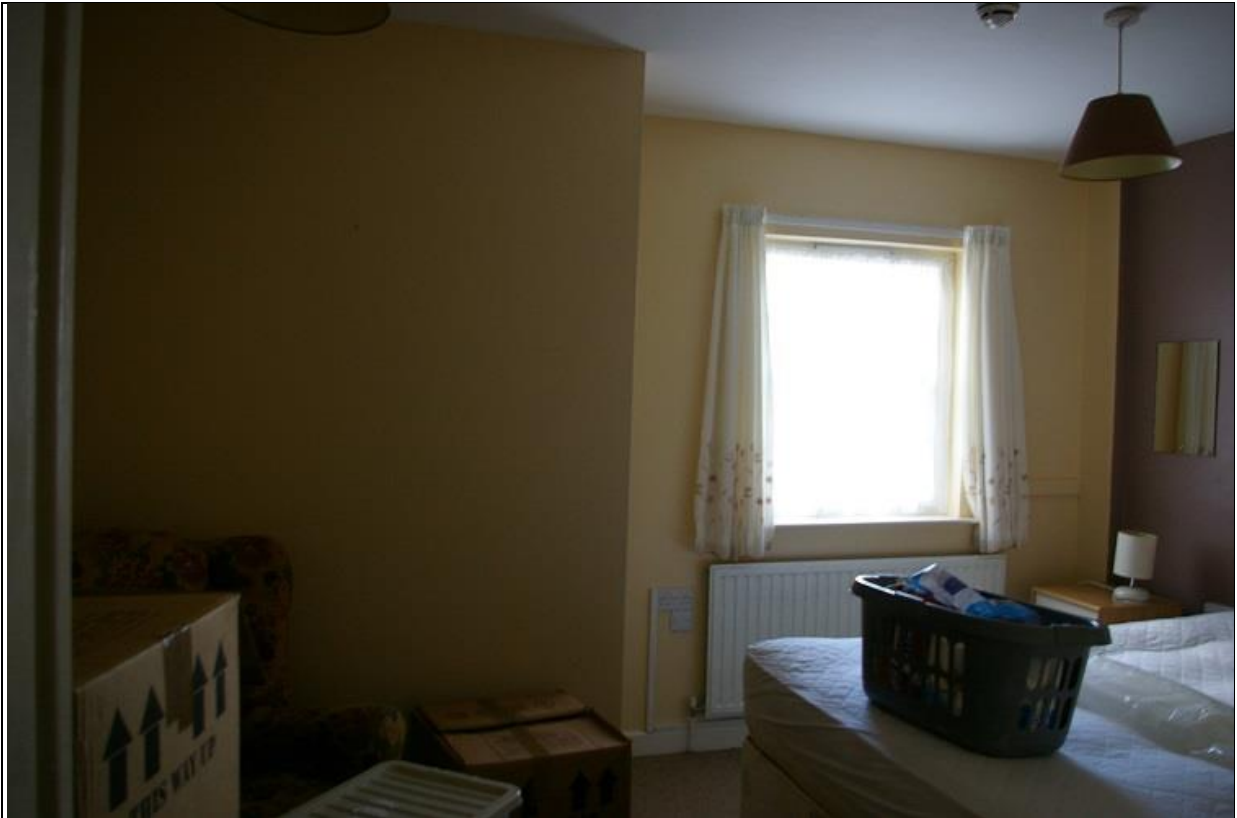
14. R17A, SHOWING WHERE THE THICK WALL OF THE SERVICE WING ENDS AND THE MODERN BLOCK EXTENDS THE RANGE; FROM THE EAST-SOUTH-EAST.
