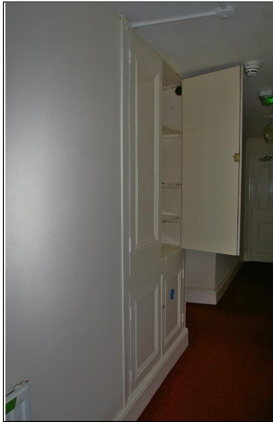
FIGURE 9: THE PANELLED CUPBOARD WITHIN THE REAR CORRIDOR IN THE PARALLEL RANGE; FROM THE EAST-NORTH-EAST.
