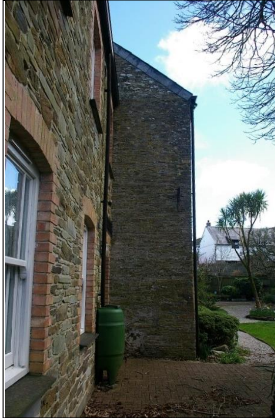
5. THE WEST GABLE OF THE MAIN RANGE, PARTIALLY OBSCURED BY THE MODERN BLOCK; FROM THE WEST.
