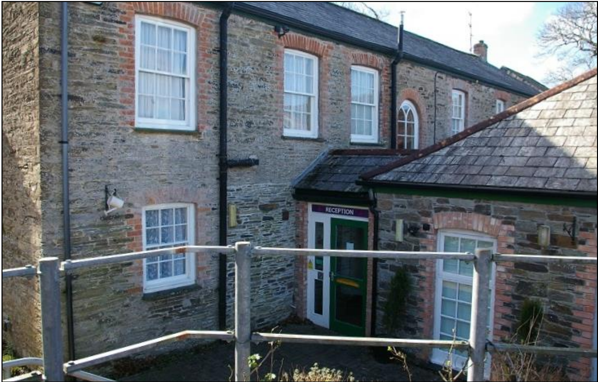
FIGURE 6: THE REAR ELEVATION OF THE PARALLEL RANGE, ABUTTED BY A NUMBER OF EXTENSIONS; FROM THE NORTH-EAST.
