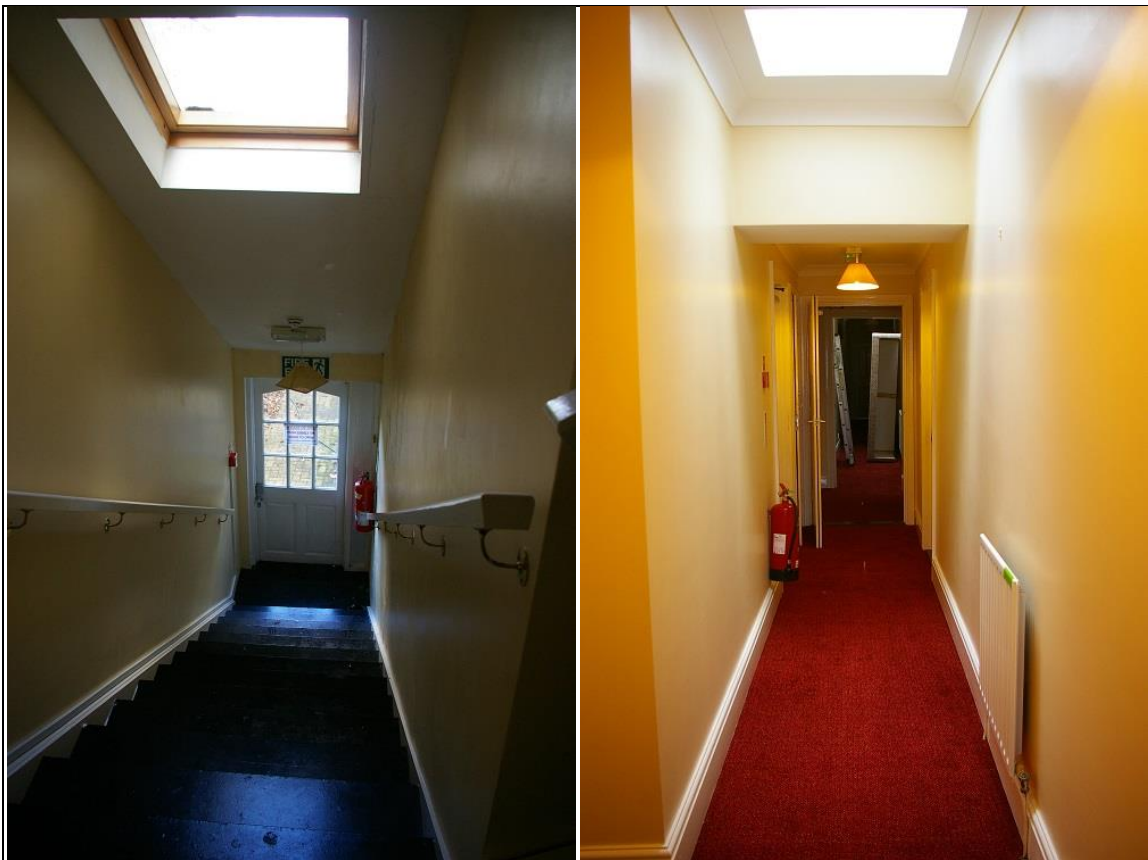
23. LEFT: THE EMERGENCY FIRE SAFETY STAIRS, MODERN; FROM THE SOUTH.
