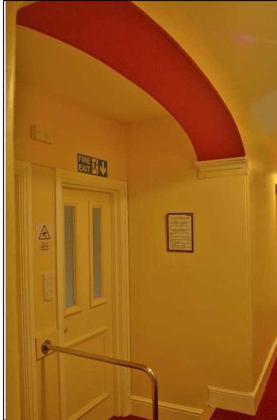
FIGURE 14: THE ARCHWAY AT THE TOP OF THE STAIRS, R25A & R25B, BETWEEN THE MAIN AND PARALLEL RANGES; FROM THE SOUTH-WEST.
