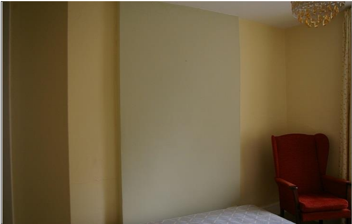
21. THE SHALLOW STACK IN R29A, WITHIN THE CROSS-WING; FROM THE NORTH-WEST.
