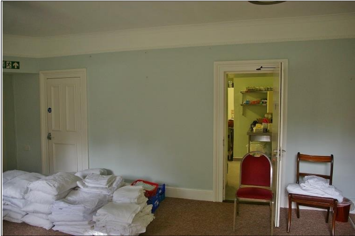
9. R3, THE CUPBOARD IN A BLOCKED OPENING AND THE FORCED DOOR TO THE REAR PARALLEL RANGE, R5; FROM THE SOUTH-EAST.
