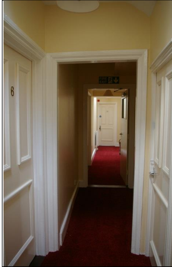
20. THE ORIGINAL TERMINUS OF THE FIRST FLOOR CORRIDOR, WITH PAIRED CONVEX MOULDED DOORS AND OPPOSITE THE LOWER DOORS TO SERVICE STAIR AND CUPBOARD; FROM THE EAST.
