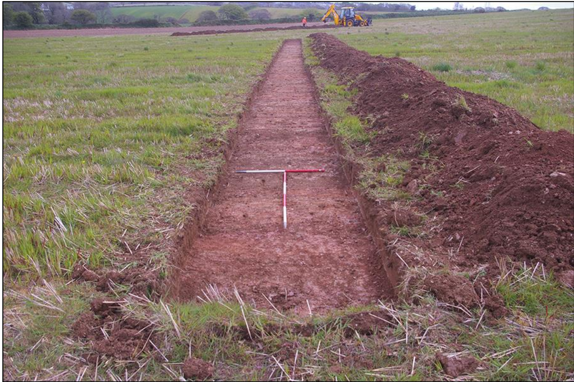
68. TRENCH 15, POST-EXCAVATION; VIEWED FROM THE WEST (1M & 2M SCALES).
