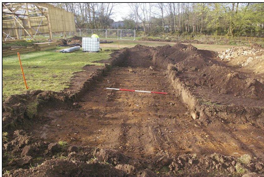
FIGURE 3: EAST SIDE OF THE EXCAVATED AREA FOR THE SWALE; VIEWED FROM THE NORTH (2M SCALE).
