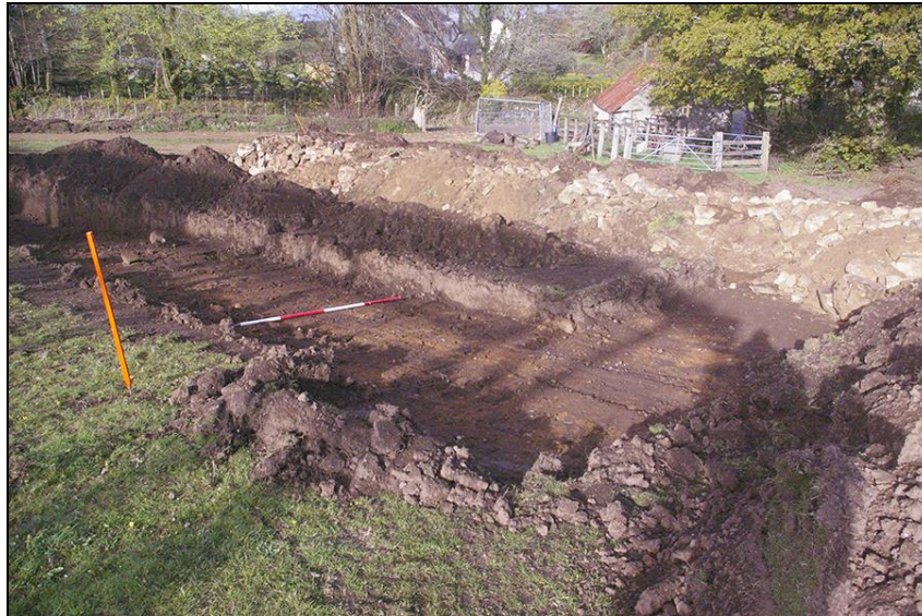
FIGURE 2: EXCAVATED AREA FOR THE SWALE; VIEWED FROM THE NORTH-EAST (2M SCALE).
