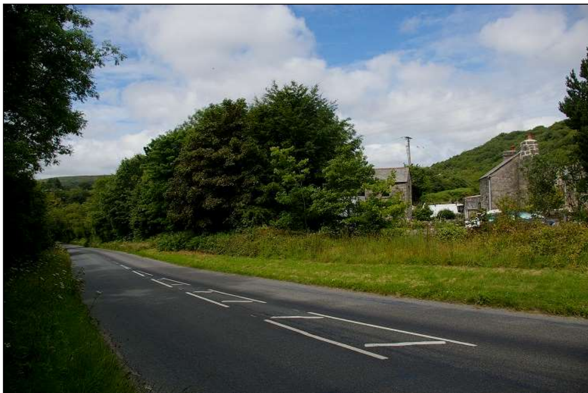
FIGURE 16: CARBEAN FARMHOUSE; VIEWED FROM THE NORTH-EAST, LOOKING DOWN THE VALLEY, ACROSS THE CHINA CLAY WORKING LANDSCAPE.
