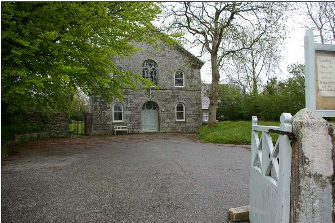
FIGURE 23: THE WESLEYAN METHODIST CHURCH AT ROCHE, AN EXCEPTIONALLY GOOD EXAMPLE OF TYPE AND VERY AUTHENTIC; FROM THE SOUTH-WEST.
