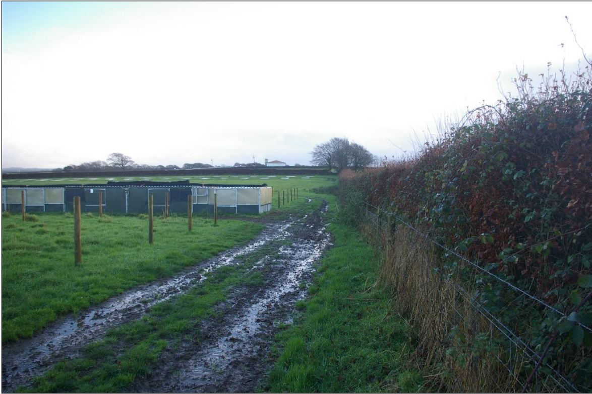
3. VIEW ALONG THE ALREADY EXISTING WORN TRACK ALONG THE WESTERN BOUNDARY TO FIELD F1, SHOWING EXISTING RUTTING WITHIN THE DRIER PART OF THE SITE; VIEWED FROM THE NORTH-WEST (NO SCALE).
