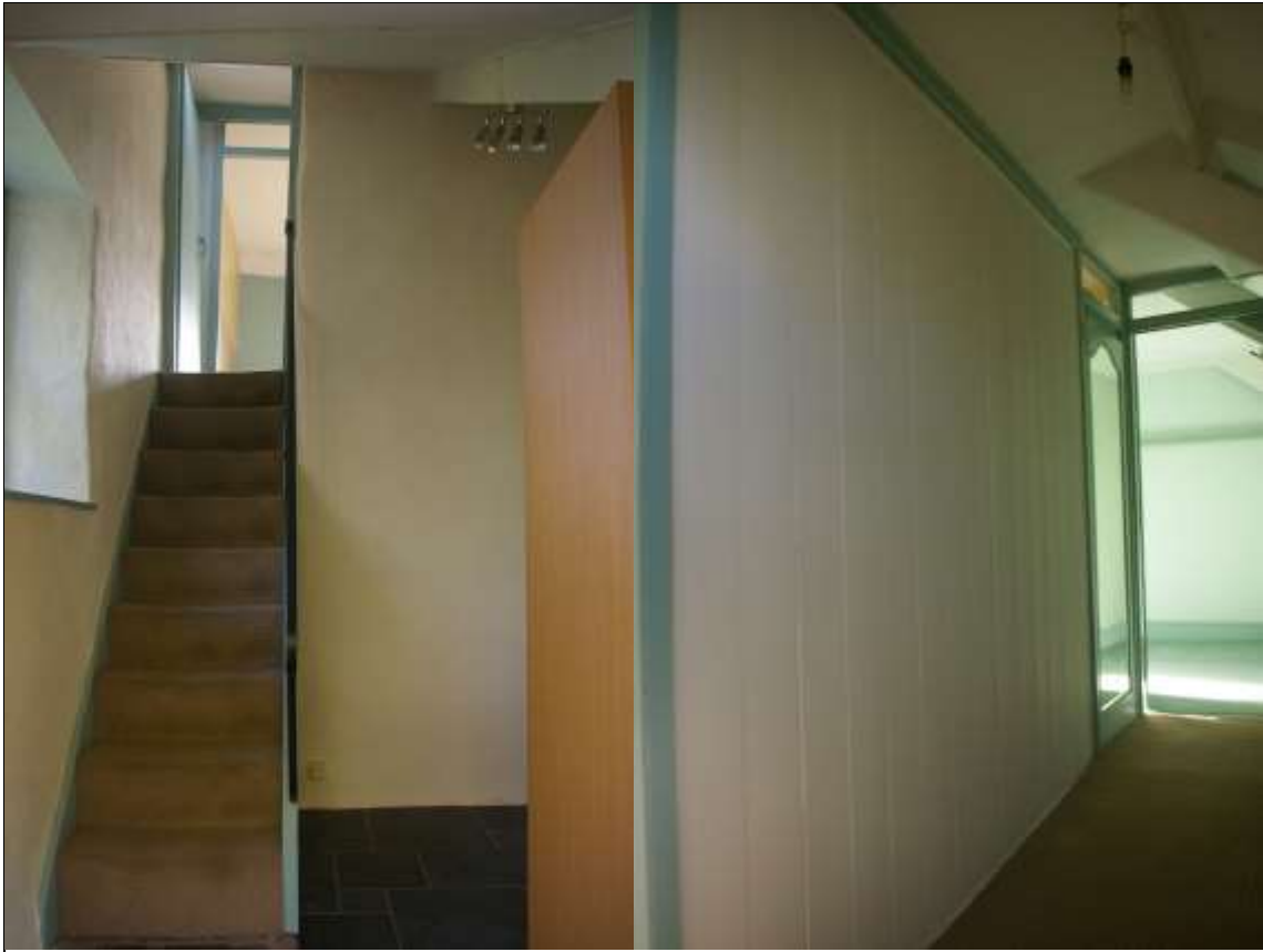
7. LEFT: THE STAIRS FORCED THROUGH THE REAR WALL OF THE MILL HOUSE; FROM THE NORTH.
