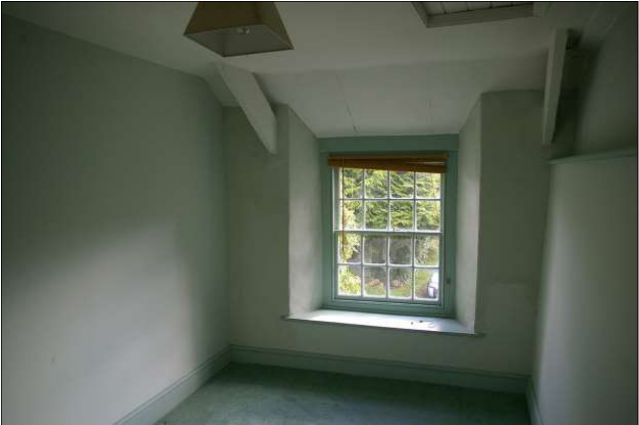
10. THE WESTERN BEDROOM; FROM THE NORTH-WEST.
