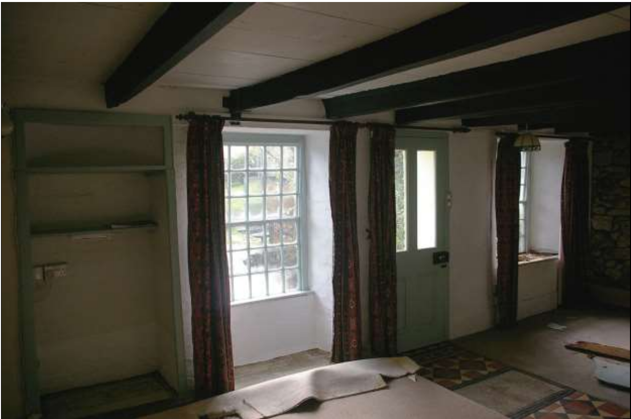
2. THE MAIN GROUND FLOOR SPACE IN THE MILL HOUSE, FORMERLY TWO ATTACHED COTTAGES; FROM THE NORTH-EAST.
