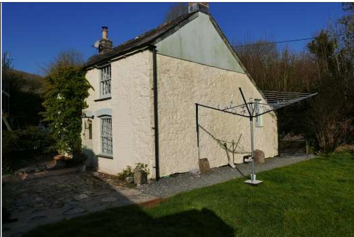
14. THE GABLED ELEVATION OF THE MILL-HOUSE; AS OF 2021; FROM THE
