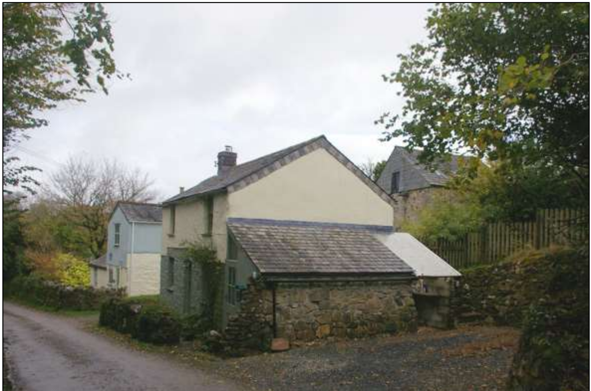
FIGURE 5: THE SITE AT HOOPER'S BRIDGE MILL; THE MILLER'S COTTAGE, THE MILL HOUSE AND WATERMILL BEHIND; FROM THE WEST-NORTH-WEST.
