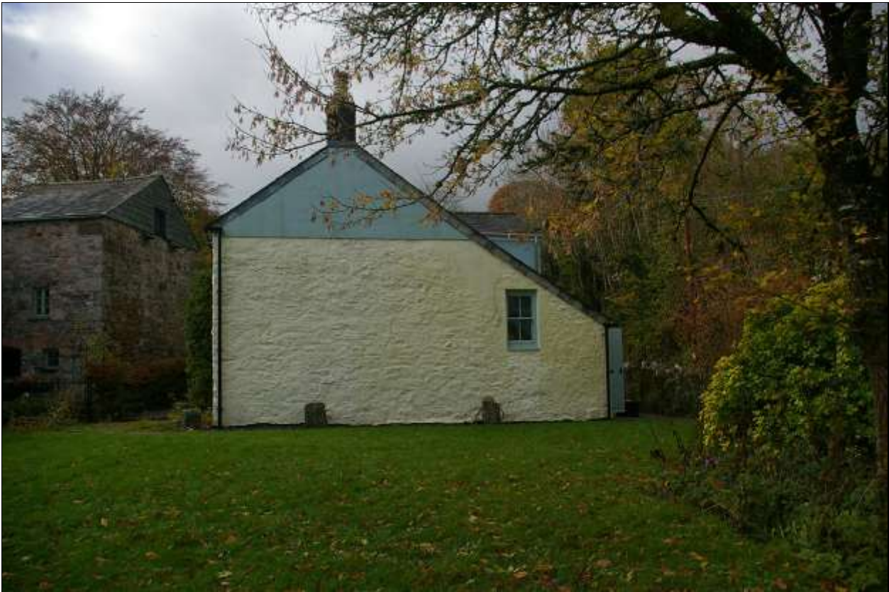
1. THE EAST ELEVATION OF THE MILL HOUSE; FROM THE EAST.
