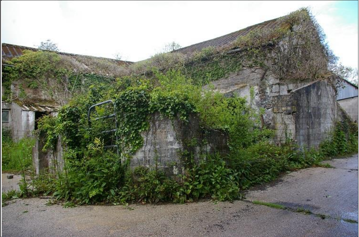
13. THE SOUTH FRONT OF BARN RANGE 4 WITH RUINED CONCRETE BLOCK BUILDINGS ATTACHED; FROM THE SOUTH-EAST.
