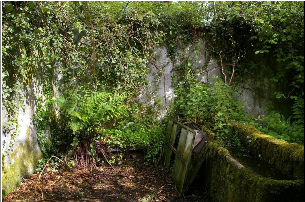
38. THE INTERIOR OF BUILDING A, BARN RANGE 1; FROM THE SOUTH.
