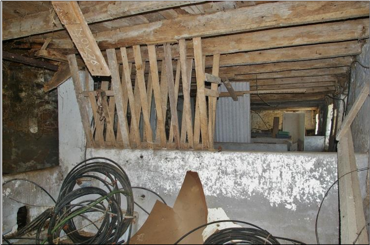
29. THE GROUND FLOOR INTERIOR OF BARN RANGE 2, BUILDING B, WITH MODERN CONCRETE PENS BREAKING UP THE SPACE; FROM THE SOUTH-EAST.
