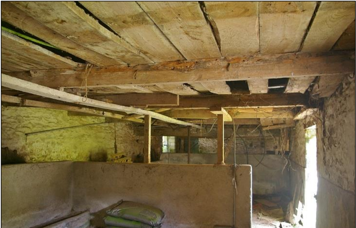
FIGURE 23: THE INTERIOR OF BARN RANGE 3; FROM THE SOUTH-SOUTH-EAST.
