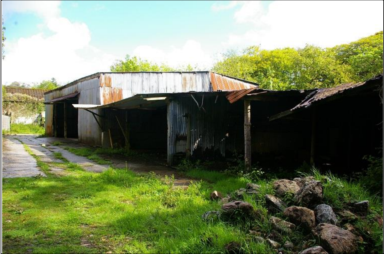
27. LONG VIEW OF THE MODERN POLE BARNs IN THE EAST YARD; FROM THE SOUTH-WEST.
