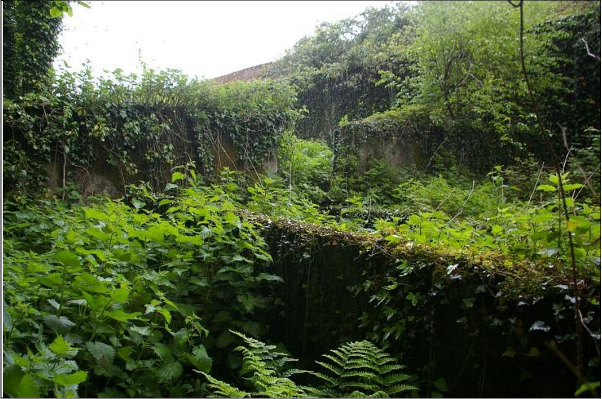
39. THE OVERGROWN INTERIOR OF BUILDING B BARN RANGE 1, SHOWING BLOCKED WINDOWS AND DOORS TO THE FORMER REAR YARD AND MODERN ANIMAL PENS; FROM THE SOUTH-WEST.
