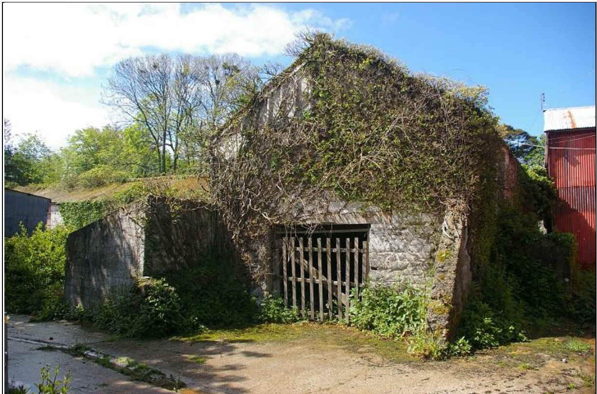
8. BARN RANGE 4, THE EAST GABLE AND CONCRETE BLOCK BUTTRESS, WITH CONCRETE BLOCK PIGSTIES TO THE SOUTH; FROM THE EAST-NORTH-EAST.
