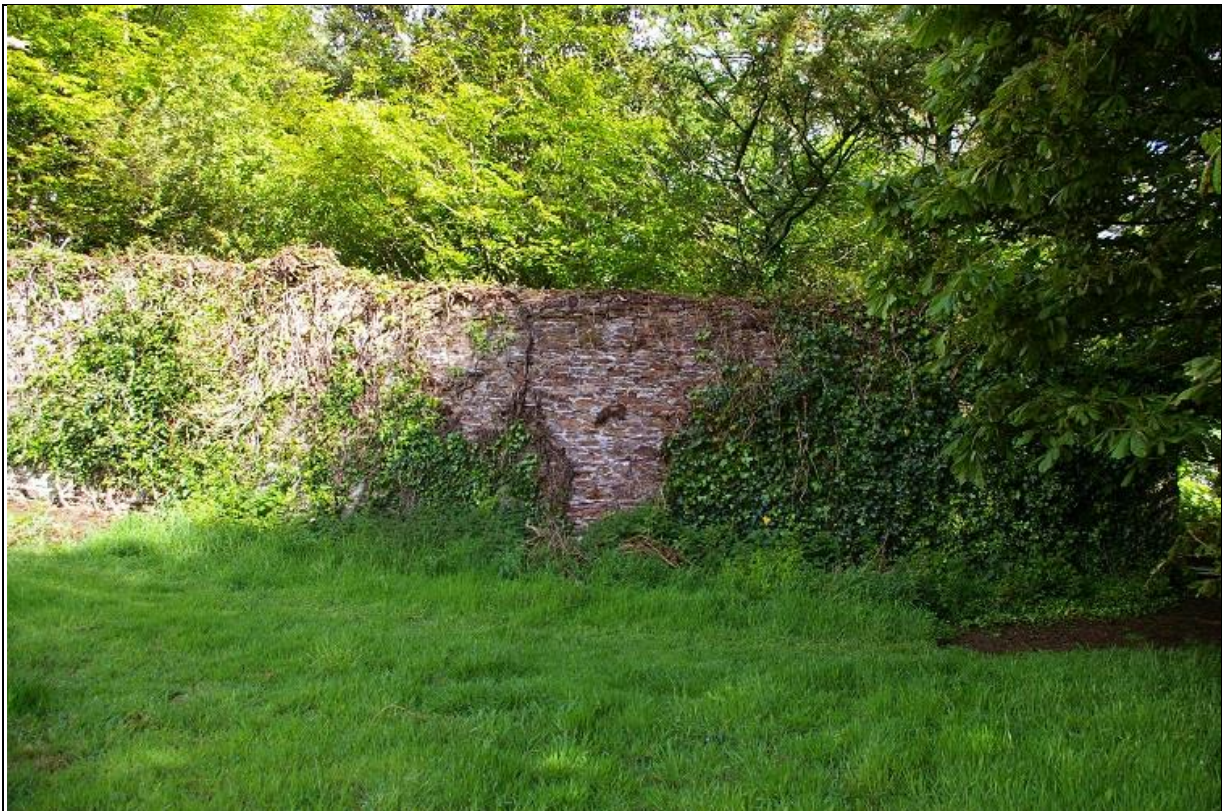
42. THE LISTED FORMER GARDEN WALLS; WEST OF THE BARNs; FROM THE SOUTH.
