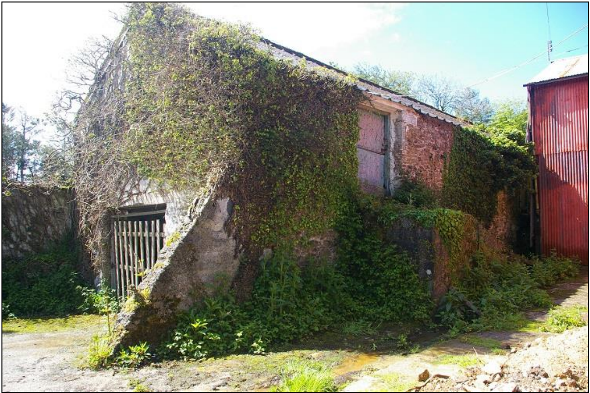
FIGURE 17: BARN RANGE 4, WITH CONCRETE BLOCK BUTTRESSES AND RAMP TO LOFT; FROM THE NORTH-EAST.
