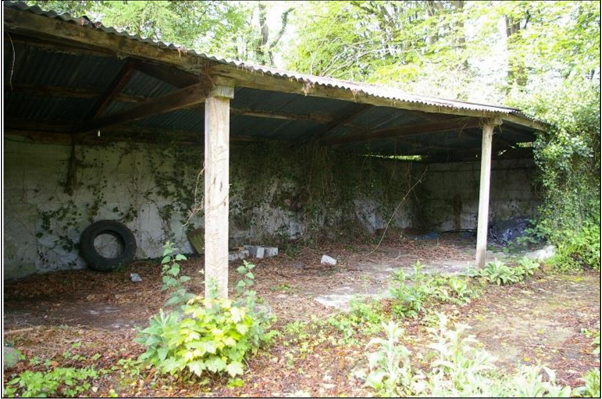
37. THE INTERIOR OF BUILDING A, BARN RANGE 5; FROM THE NORTH-EAST.
