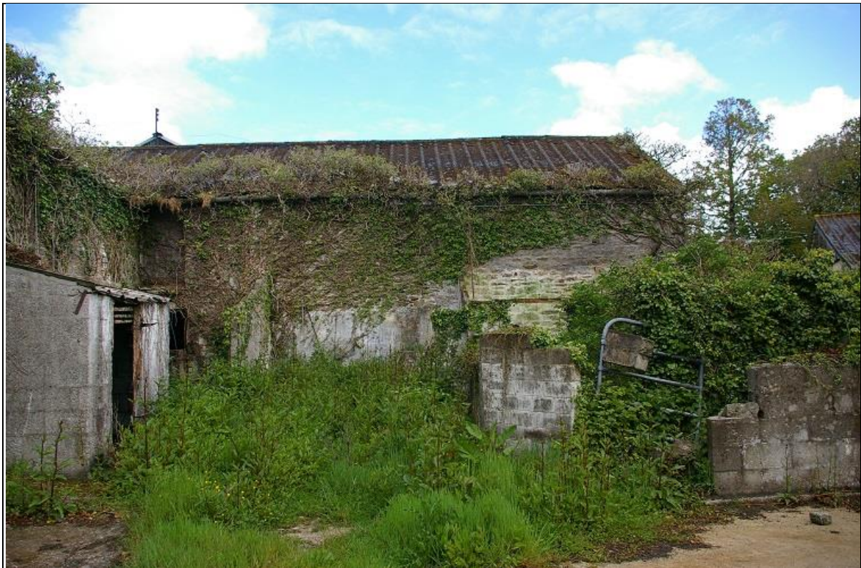
14. THE SOUTH ELEVATION OF BARN RANGE 4, SHOWING THE PROJECTING STUB WALL OF THE FORMER PROJECTION SHOWN ON THE HISTORIC MAPPING; FROM THE SOUTH.
