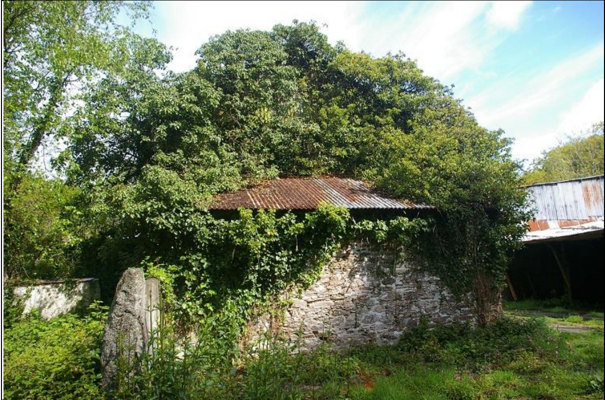
33. BARN RANGE 2, BUILDING A; FROM THE SOUTH.
