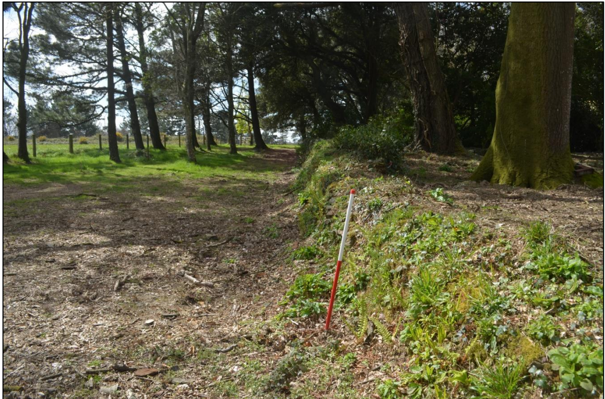
FIGURE 112: THE BOUNDARY CONTINUES TO THE WEST, BECOMING MORE OF A CORNISH HEDGE BANK IN FORM. FROM THE EAST.
