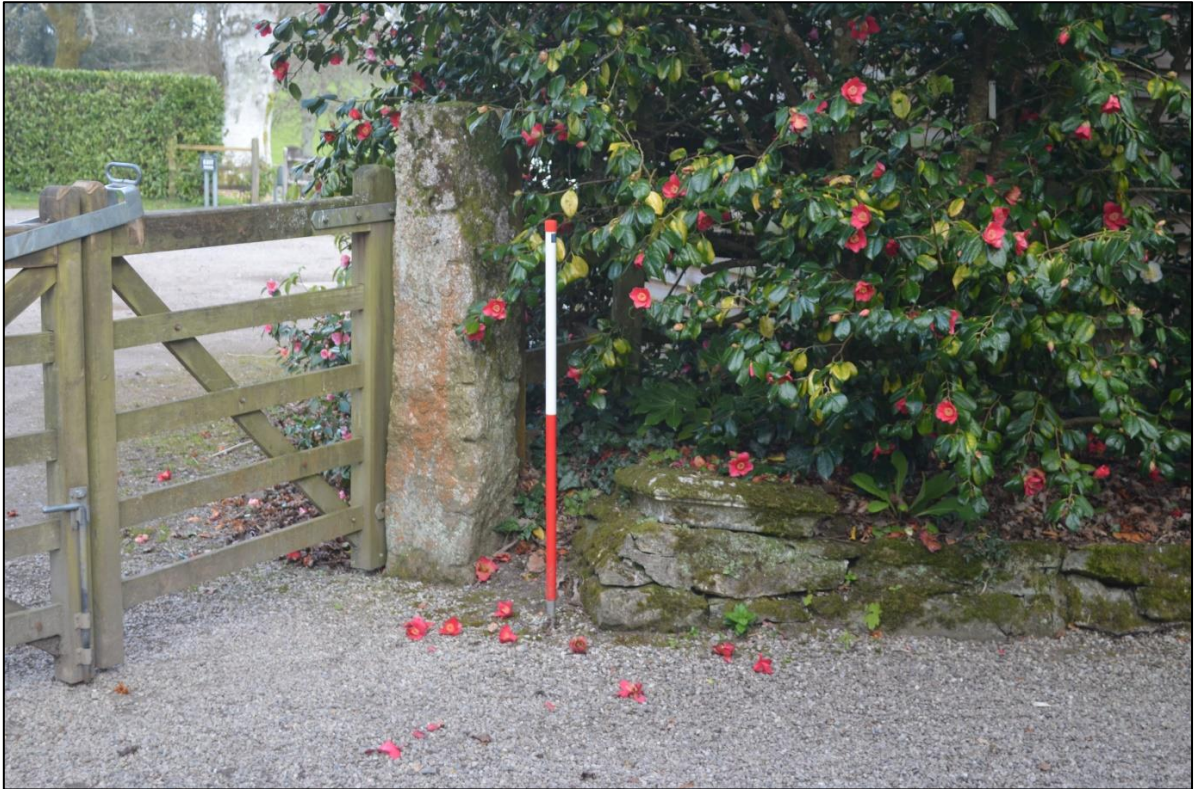
FIGURE 61: STONE GATE POST AND SQUARE CAPPING STONE (JUST TO THE RIGHT OF THE RANGING POLE) RESTING ON A LOW WALL AT AN ENTRANCE INTO TREWITHTEN GARDENS. FROM THE SOUTH
