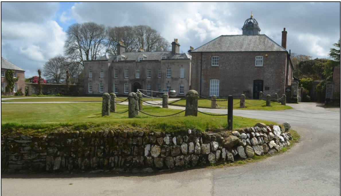
FIGURE 91: CURVED END OF HA-HA IN FRONT OF TREWITHEH HOUSE CONSTRUCTED OF QUARTZ BLOCKS. FROM THE NORTH.
