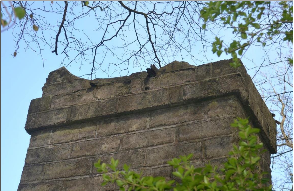
FIGURE 30: DETAIL OF THE SEMI-CIRCULAR TOP TO ONE OF THE PILLARS, NOW BROKEN, WITH EVIDENCE OF IRON FIXINGS. FROM THE SOUTH WEST
