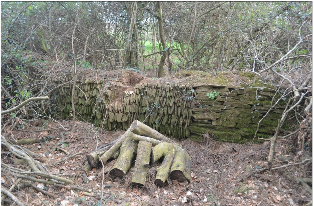
FIGURE 115: SOUTHERN SECTION OF THE BOUNDARY WITH THE STONWORK EVIDENT AND A SMALL AREA OF COLLAPSE. FROM THE WEST.
