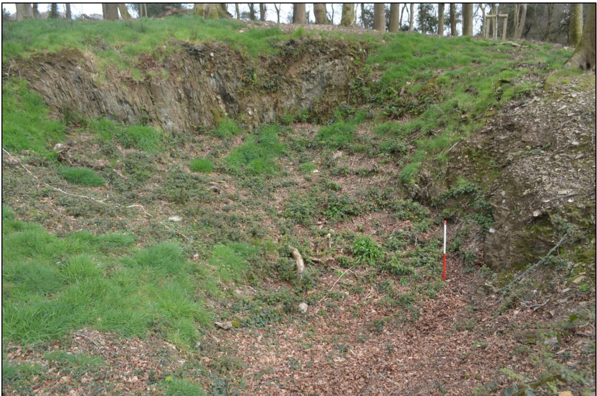
FIGURE 44: HISTORIC QUARRYING, LIKELY TO BE THAT RECORDED ON THE ORDNANCE SURVEY FIRST EDITION MAP AS 'OLD QUARRY'. FROM THE SOUTH
