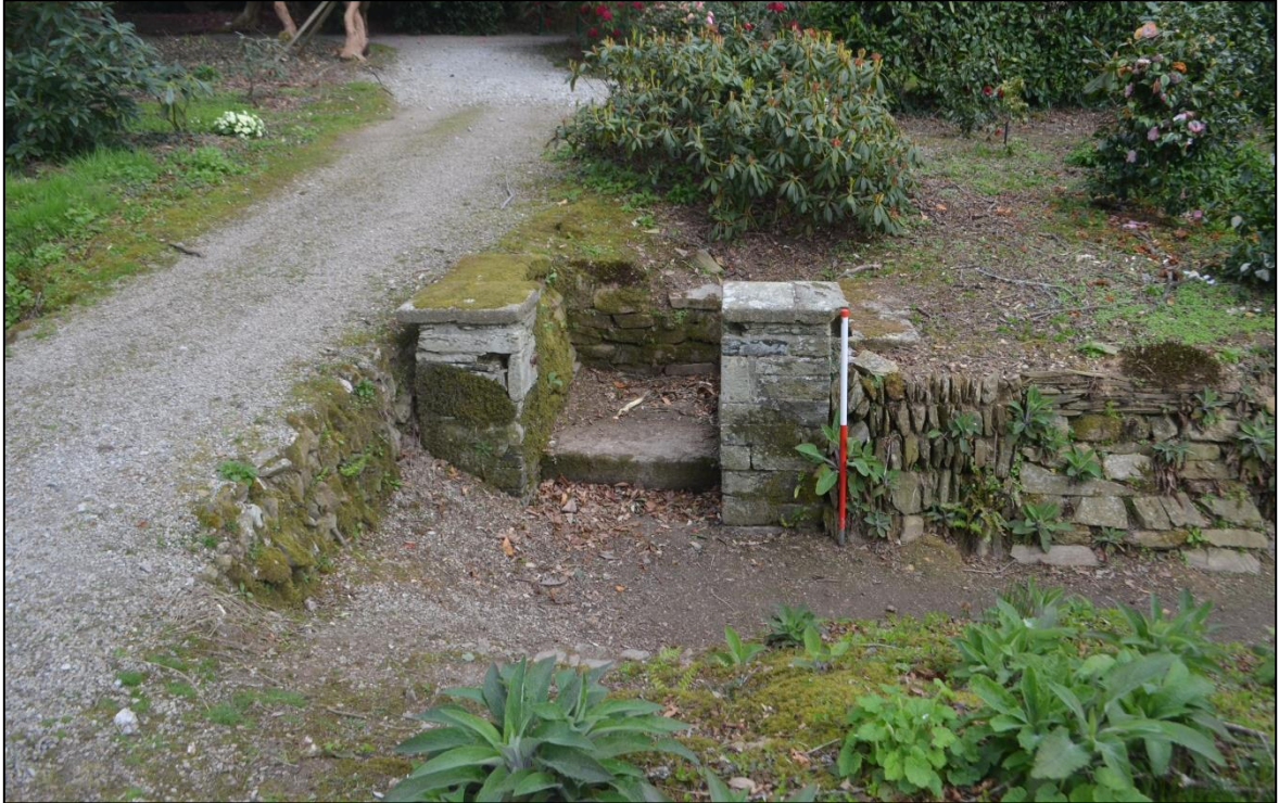
FIGURE 135: SET OF STONE STEPS PROVIDING ACCESS WITH EVIDENCE OF METAL GATE FIXINGS. FROM THE SOUTH
