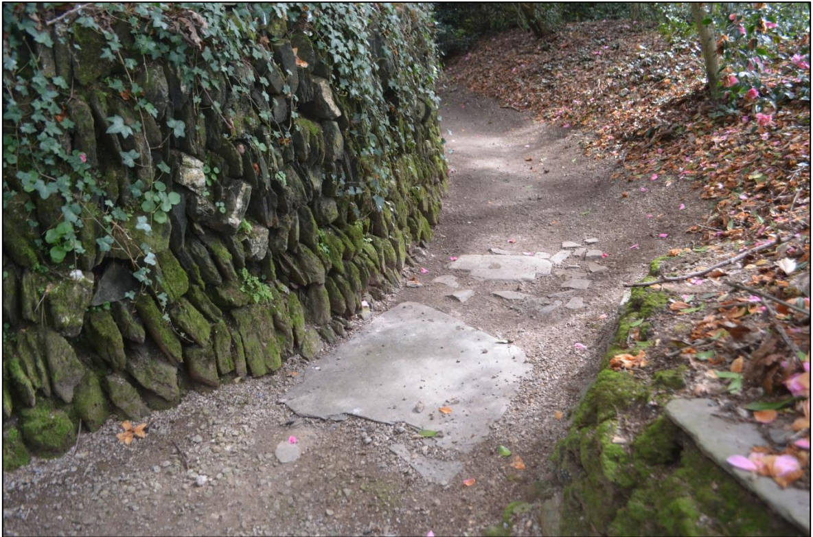
FIGURE 148: ONE LARGE AND ONE SMALLER FLAG STONE APPEAR TO HAVE BEEN LAID AT THE POINT WHERE STEPS DESCEND DOWN INTO THE CURVED SECTION OF THE HA-HA. FROM THE WEST
