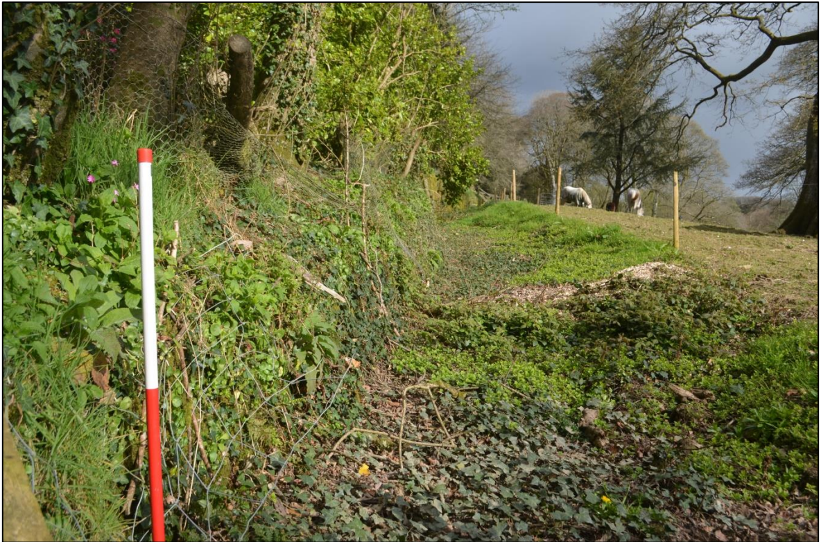
FIGURE 110: A CHANGE IN BUILD FORM AND QUALITY IS DISCERNIBLE AT THE SOUTHERN END OF THE HA-HA WHERE IT APPEARS TO HAVE BEEN EXTENDED AFTER 1747 BUT PROBABLY BEFORE 1841.
