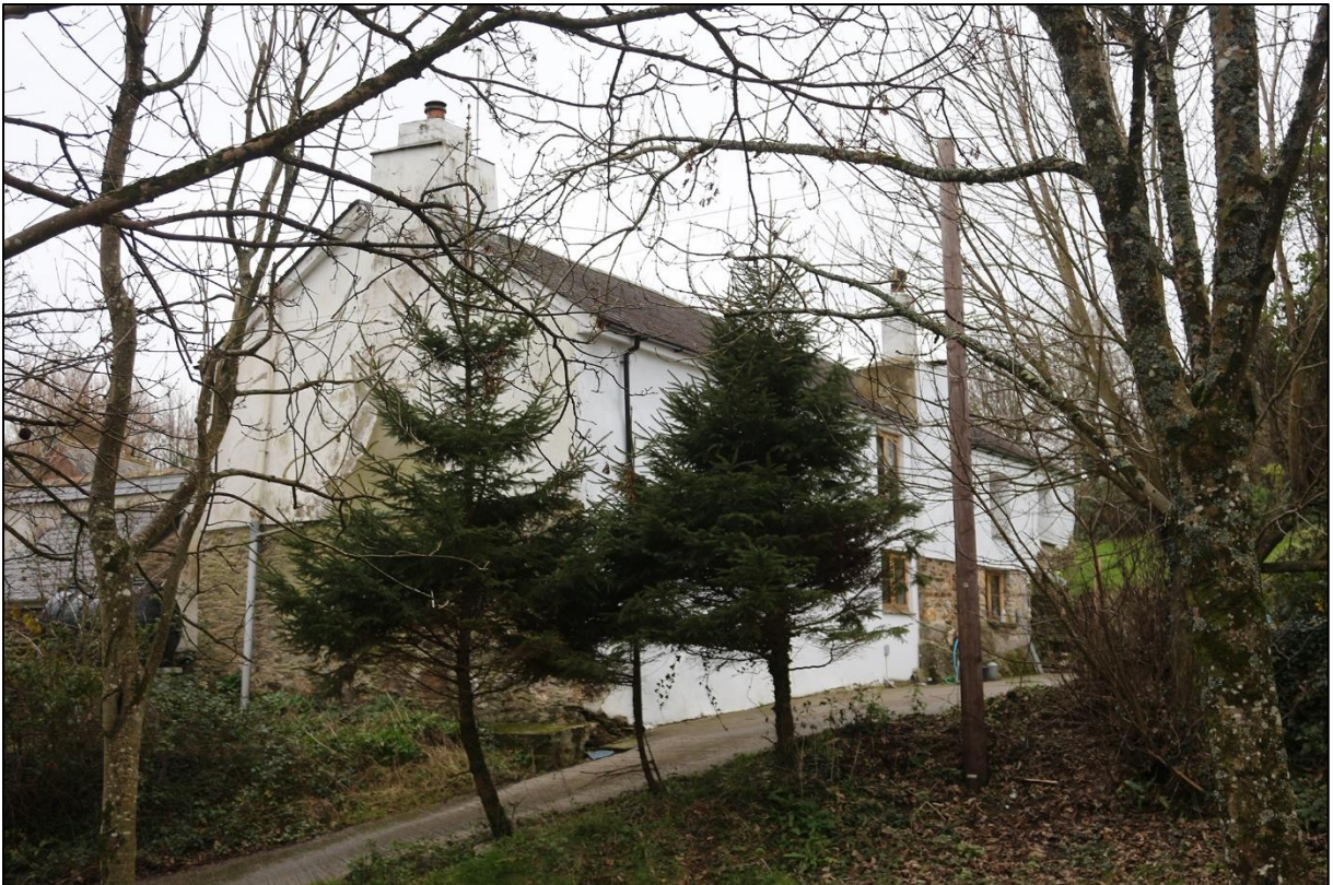
16. THE UNLISTED FARMHOUSE AT LOWERTOWN; NOTED THE MASSIVE GABLE AND LATERAL STACKS; VIEWED FROM THE NORTH.
