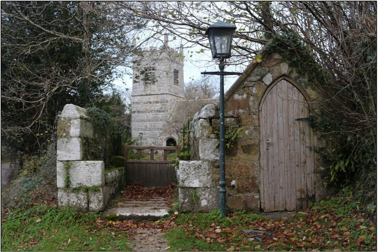
1. THE SOUTH GATE OF THE CHURCHYARD; VIEWED FROM THE SOUTH. THE BIER HOUSE COULD ALSO BE THE WORK OF WILLIAM WHITE.
