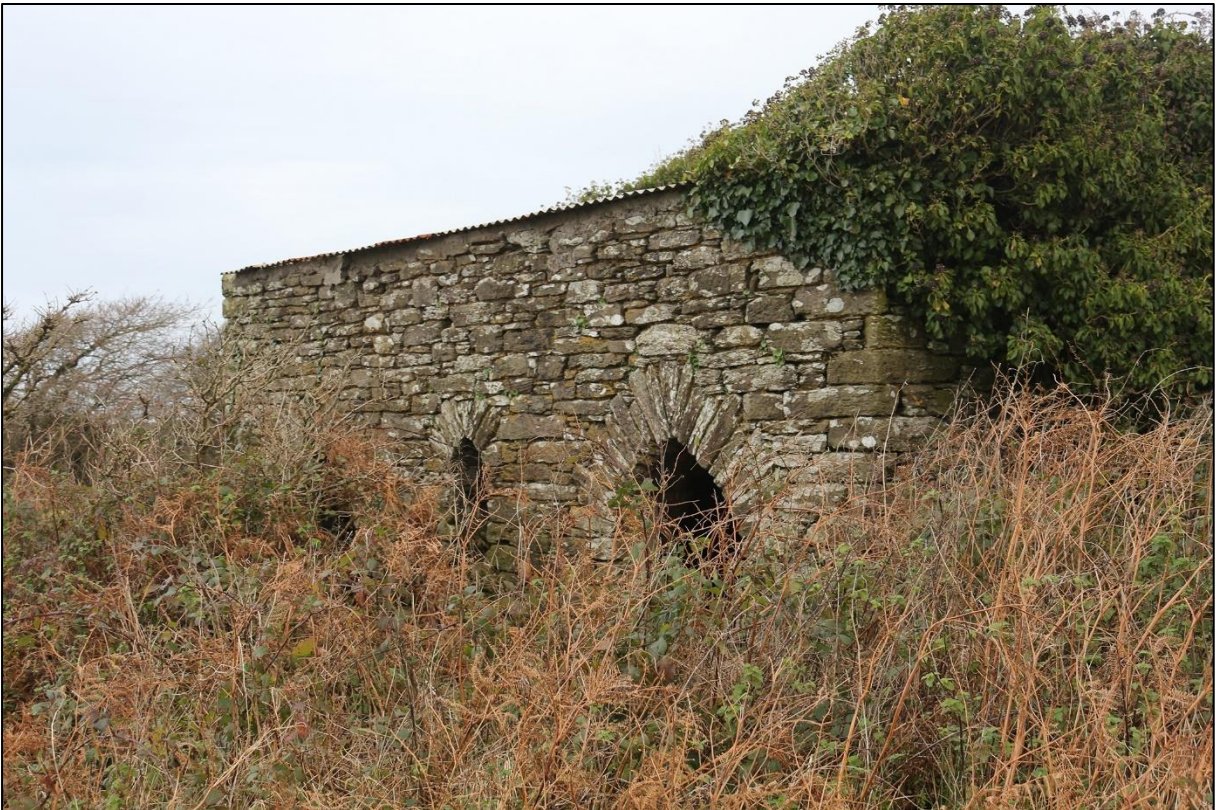
26. THE 'WELLHOUSE' ON THE EDGE OF FIELD 4; VIEWED FROM THE SOUTH.
