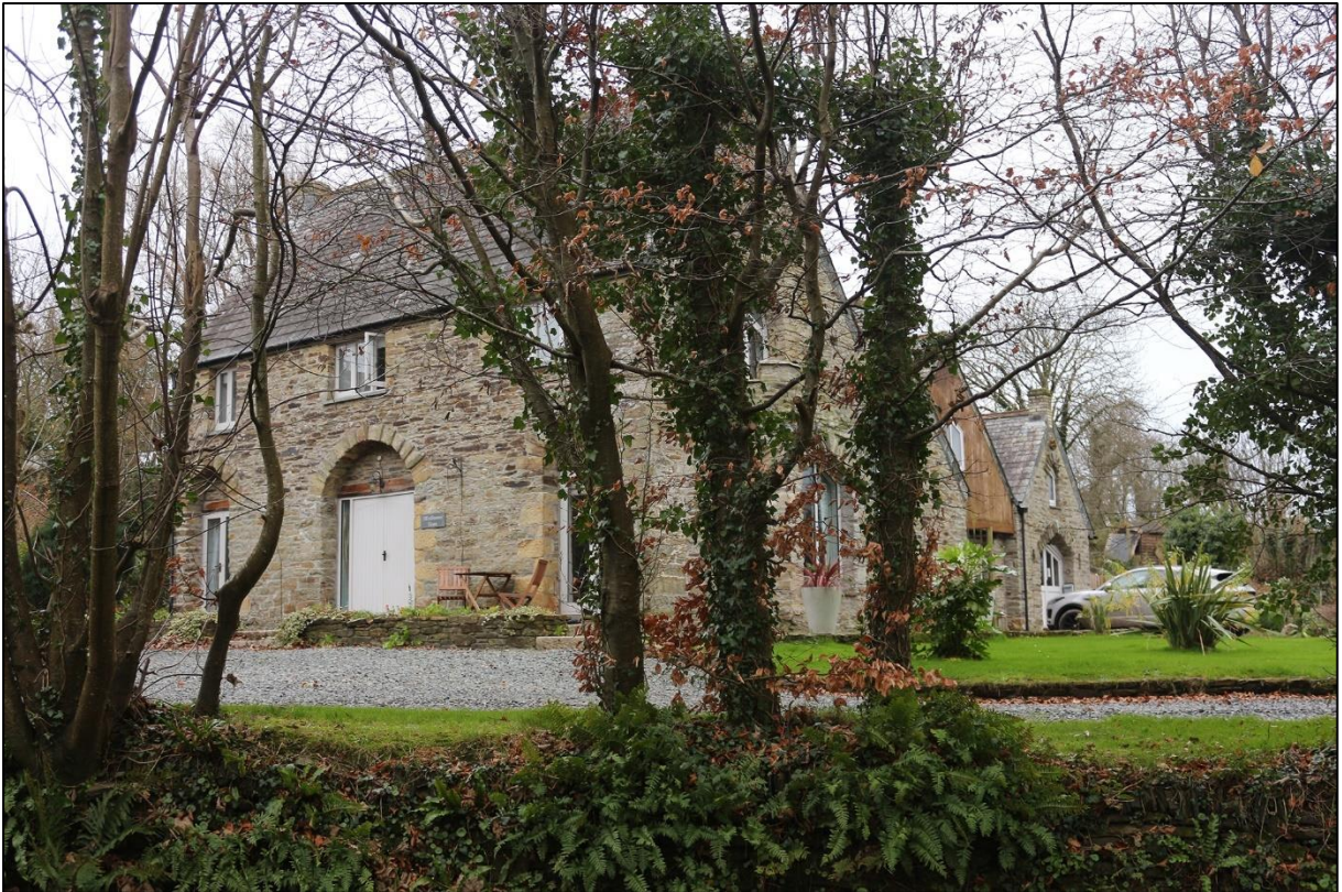
13. THE LISTED 'BARN' AT LOWERTOWN ( MELLIONEC VEAN ), A GOTHIC REVIVAL HOUSE BY WILLIAM WHITE; VIEWED FROM THE NORTH-EAST.
