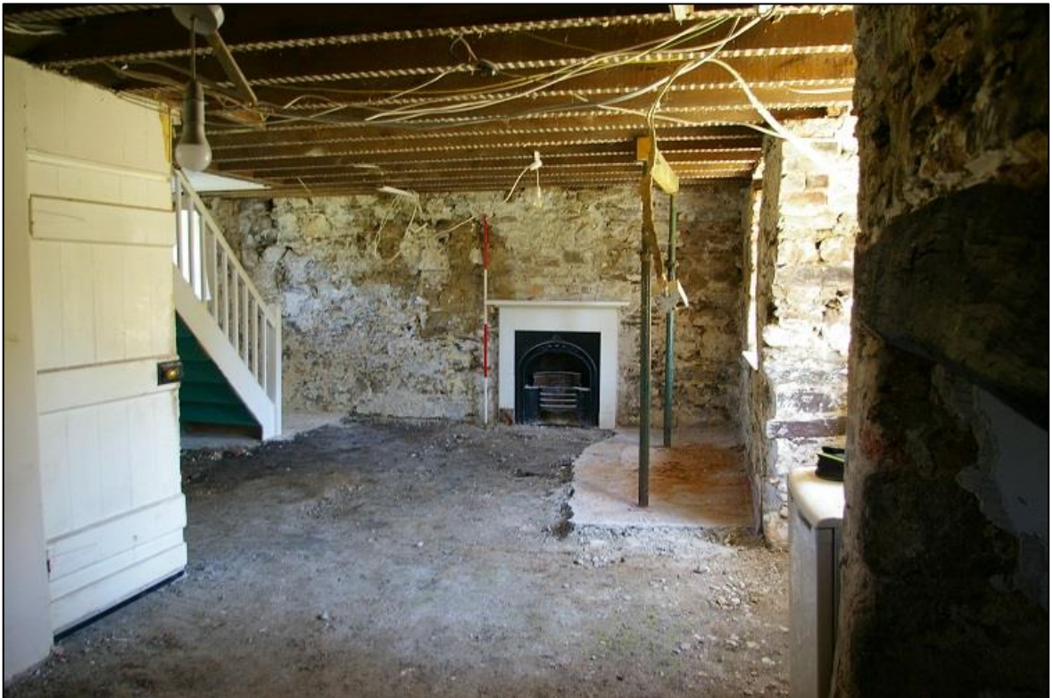
4. THE EXTENDED NORTH GABLE, WITH BOX HEARTH, WITH RAISED BASKET GRATE (2M SCALE); FROM THE SOUTH-EAST.
