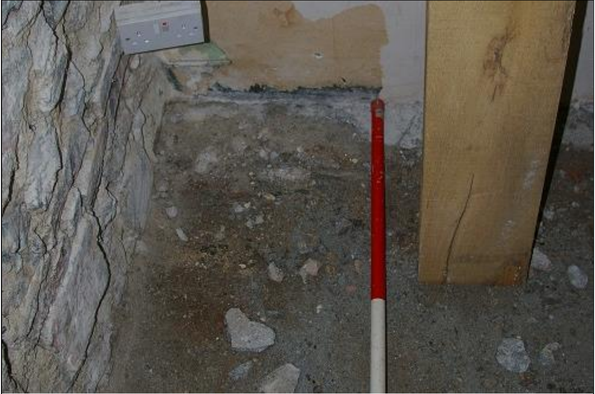
FIGURE 9: NARROW, LINEAR, SPLIT SLATE COBBLES PARALLEL WITH THE PLANK PARTITION WHICH FORMS THE HALLWAY TO THE SOUTH END OF FORMER COTTAGE NO.2; FROM THE NORTH (2M SCALE).
