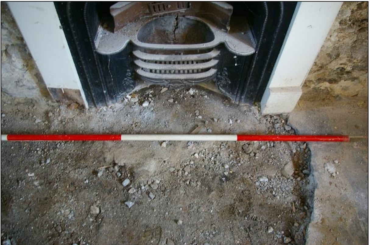
FIGURE 6: PATCH OF COBBLES IN FRONT OF BOX HEARTH, PARTIALLY OBSCURED BY LOWER LAYERS OF CEMENT FLOOR; FROM THE SOUTH (2M SCALE).
