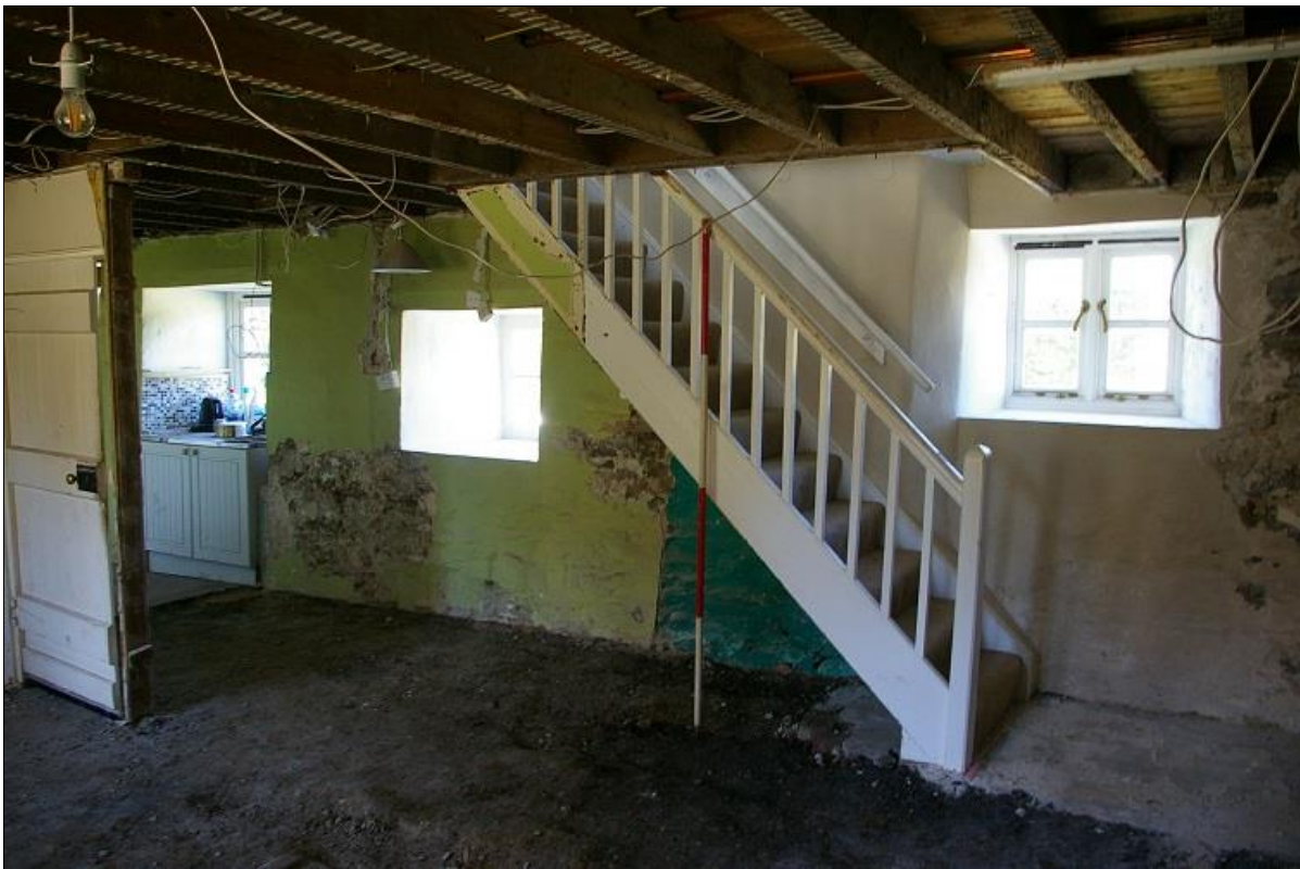
2. THE REAR WALL OF THE COTTAGES, WITH MODERN STAIRCASE TO THE FIRST FLOOR; FROM THE EAST-NORTH-EAST, WITH 2M SCALE.
