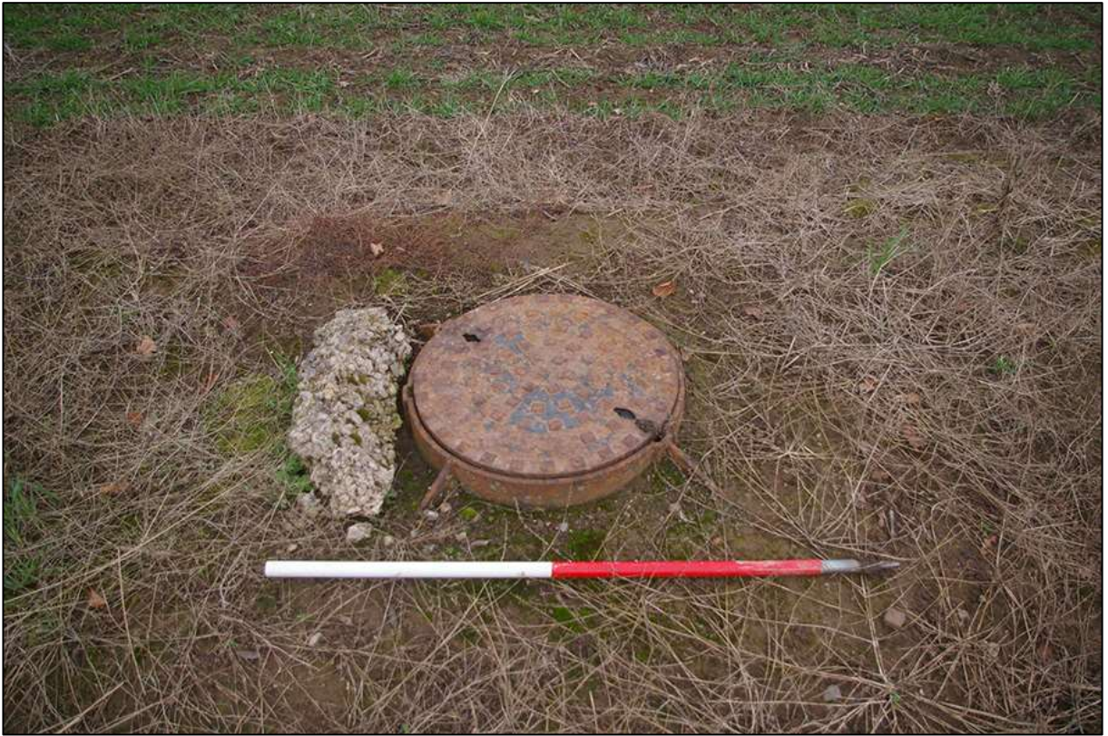
7. DETAIL OF THE MAN-HOLE COVER TOWARDS THE MIDDLE OF FIELD F1; VIEWED FROM THE SOUTH (1M SCALE).
