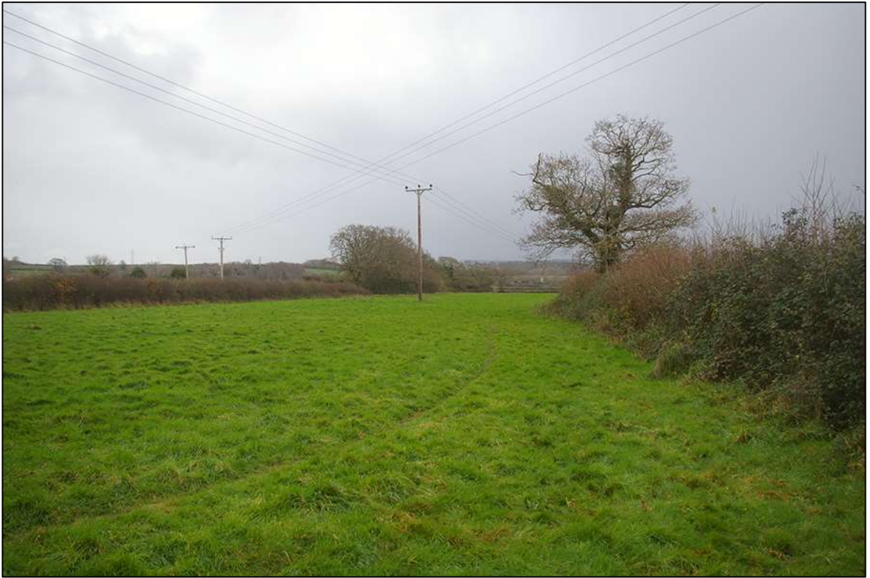
55. VIEW ACROSS FIELD F9 FROM THE NORTH-WEST CORNER, SHOWING DETAIL OF OVERHEAD CABLES; VIEWED FROM THE NORTH-WEST (NO SCALE).
