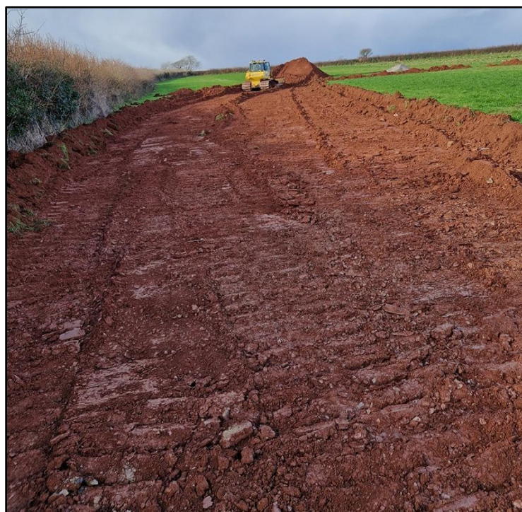
FIGURE 4: SHOT OF AREA STRIP FROM SE CORNER LOOKING WEST (NO SCALE).
