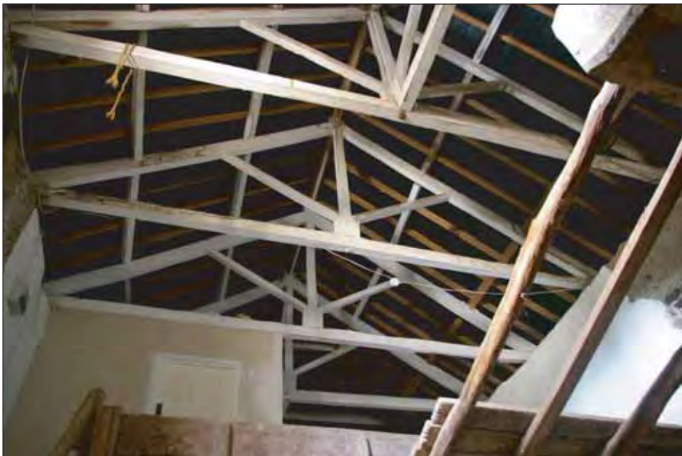
Plate 2: The roof structure viewed from the north.
