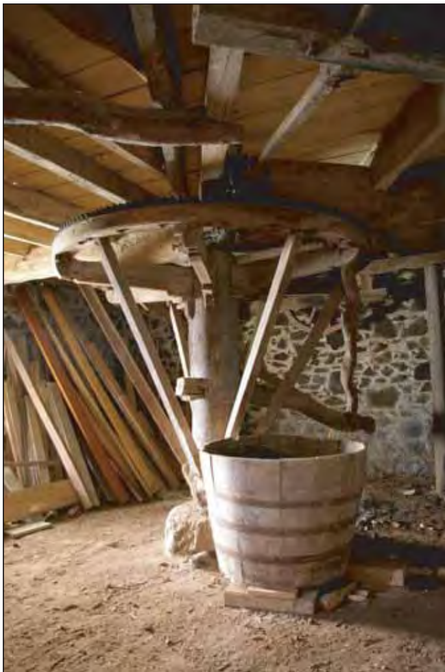
Plate 4. The interior of the Cider Barn viewed from the north west.
