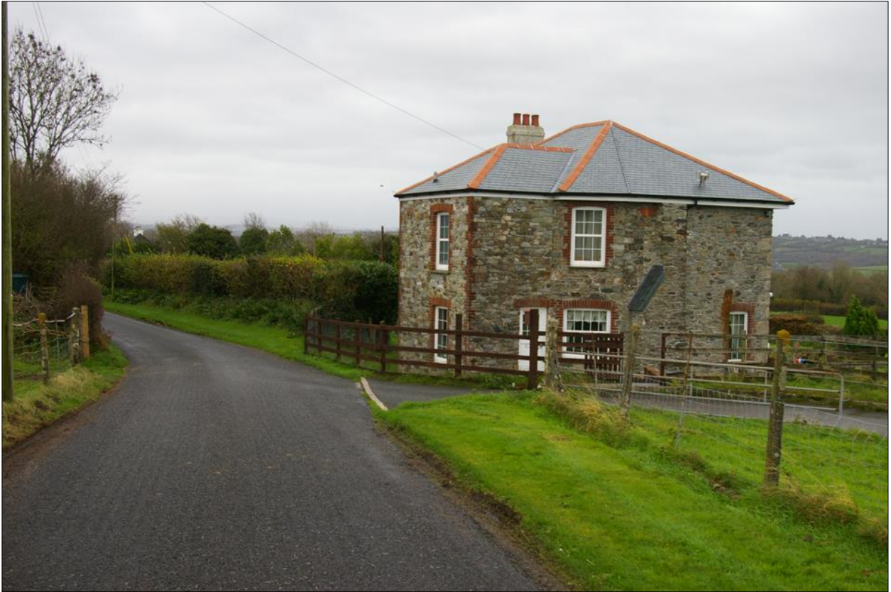
52. Another GII Listed asset at East Calstock Mine; viewed from the west.
