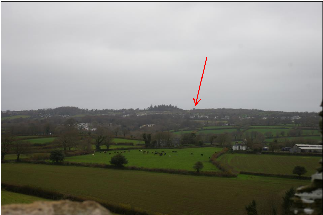
63. As above, detail. The Listed engine house at the Hingston Down Mine is indicated.
