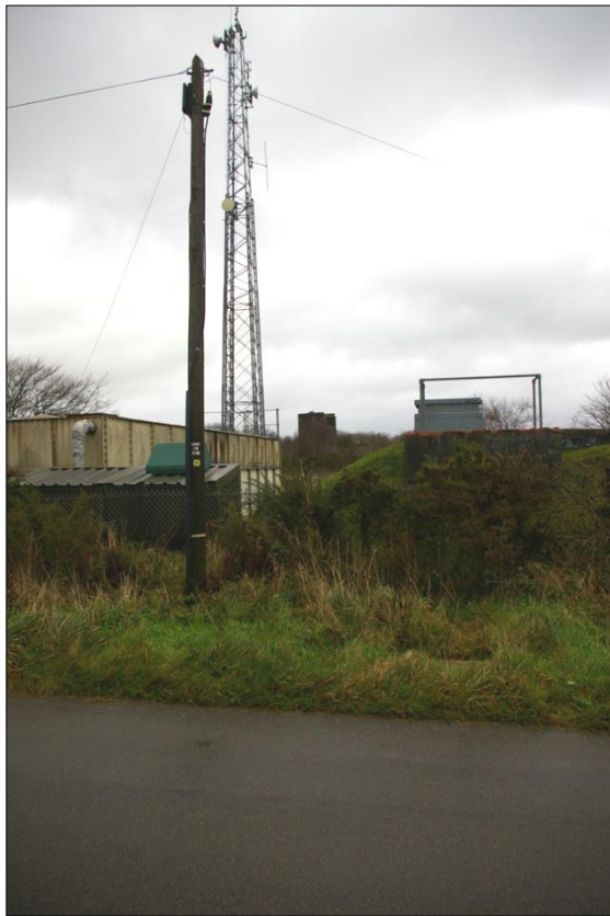
14. The telecoms mast and compound next to the west access to the Hingston Down Mine site; viewed from the west.
