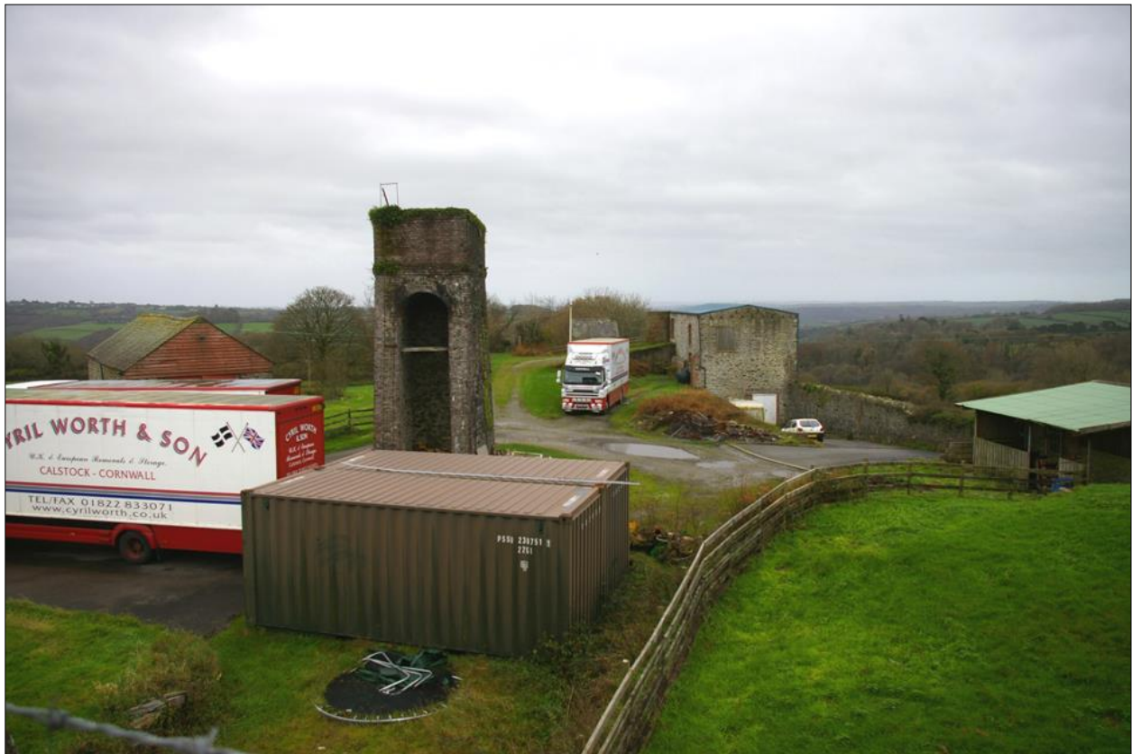
51. The water tower at East Calstock Mine, viewed from the north.
