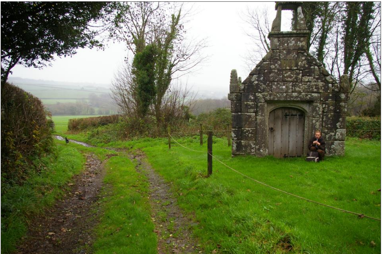
81. As above, viewed from the south.
