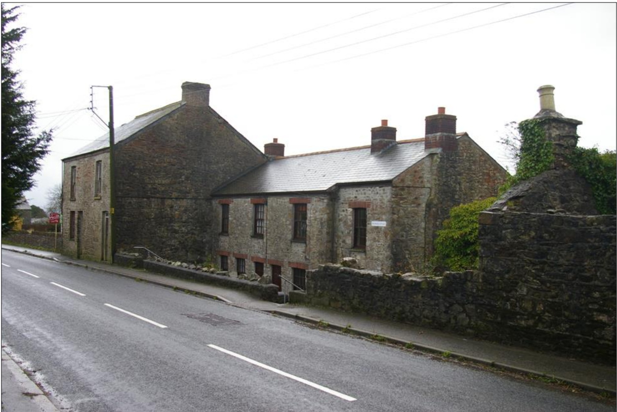
32. View of the GII Listed cottages in St Ann's Chapel, Candycroft and Vendor; viewed from the north-west.
