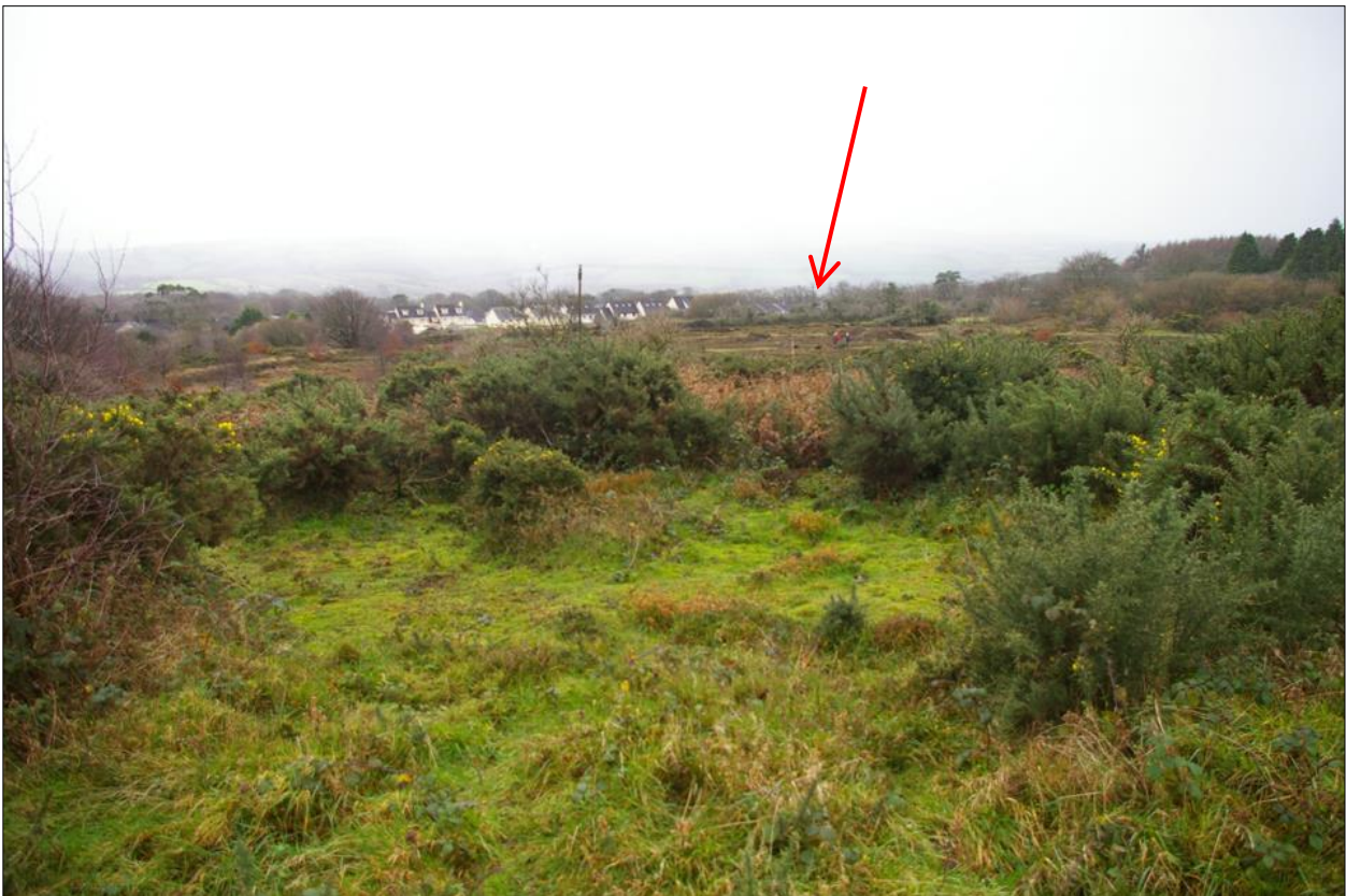
21. View across the Hingston Down Mine site from the north-east, looking down and across the site to the location of the proposed development; viewed from the north-east.
