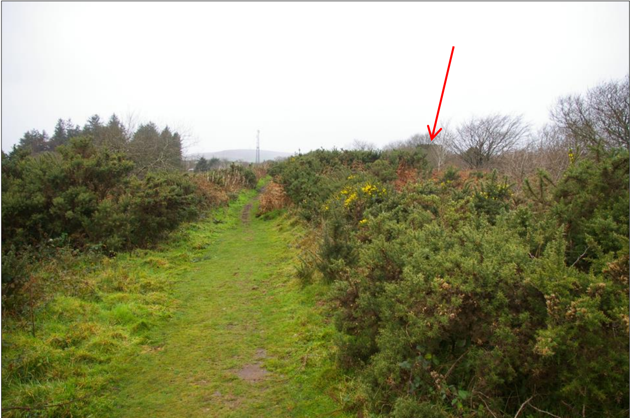
20. View across the Hingston Down Mine site from the east; the engine house is just visible on the right (indicated).
