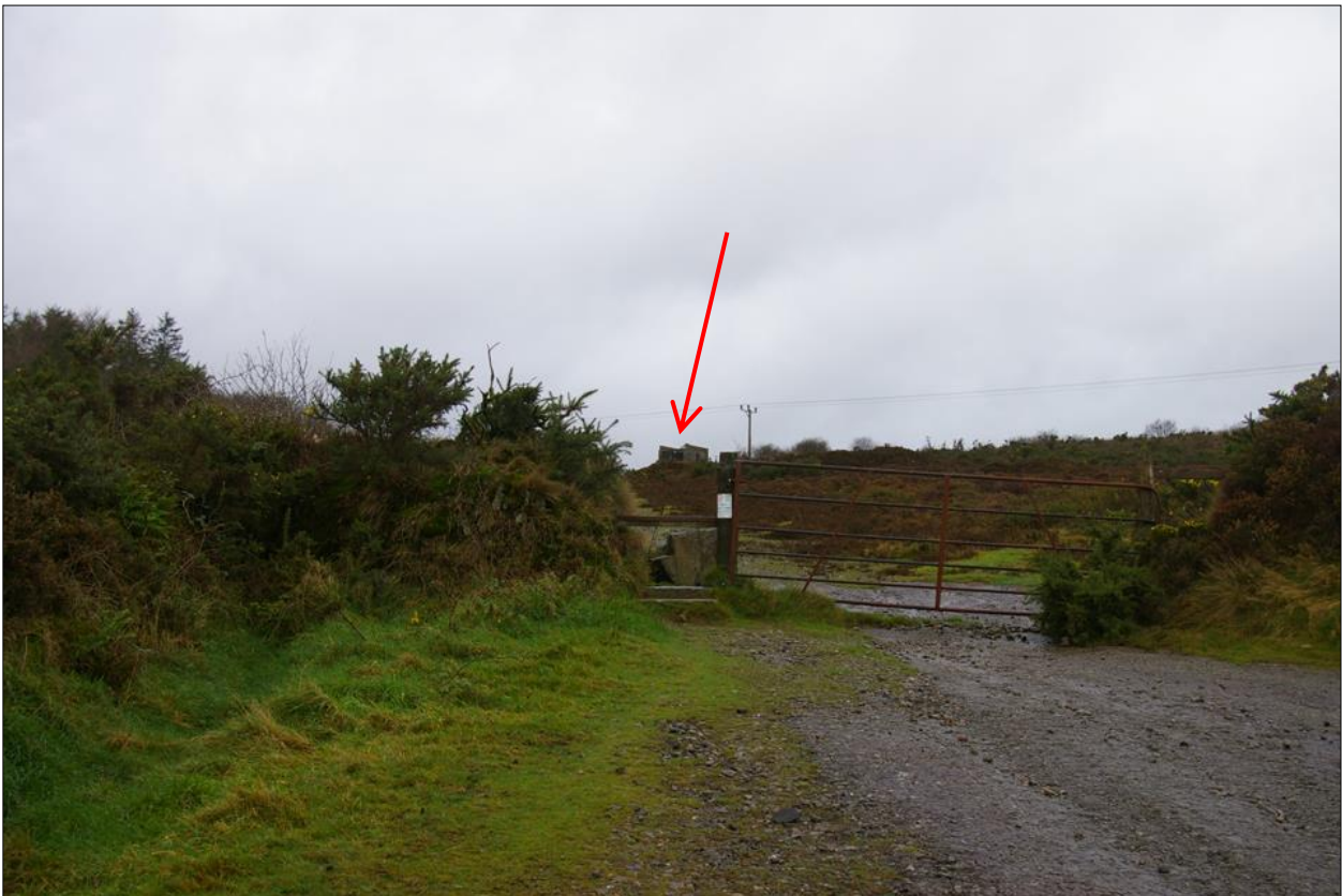
24. The end of Old Mine Road and the entrance to the Hingston Down Mine site; viewed from the south. The engine house is indicated.
