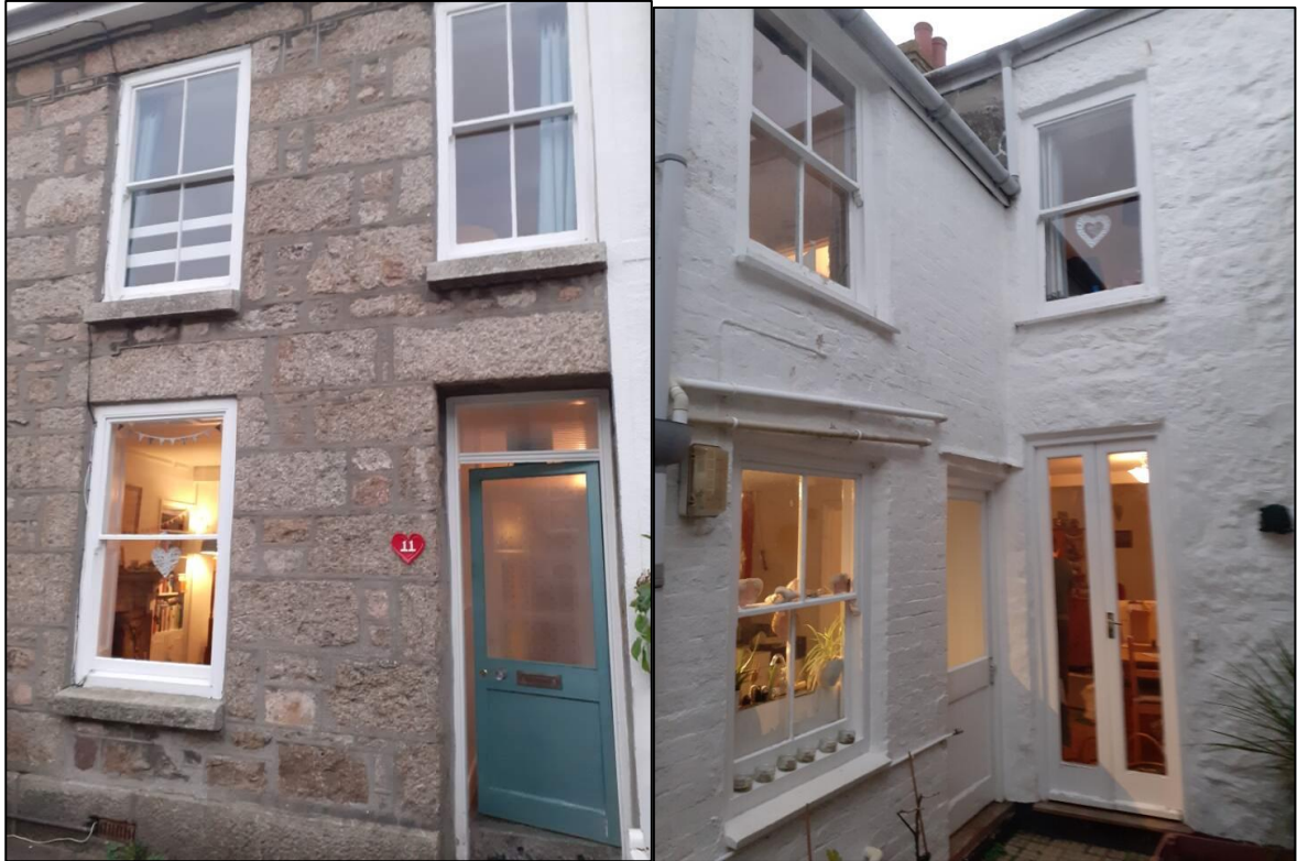
FIGURE 4 (LEFT): THE WINDOWS AT THE FRONT OF THE PROPERTY.
