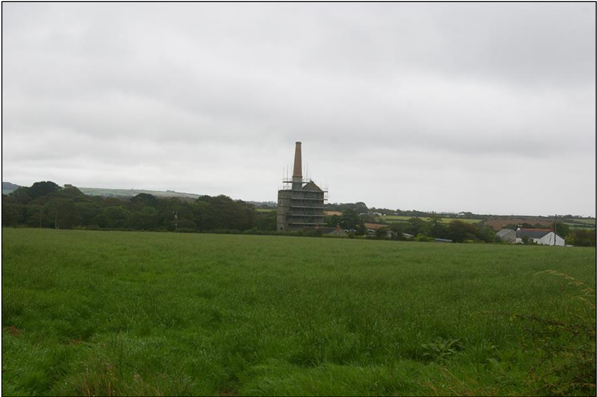
17. THE ENGINE HOUSE AT IVEY'S SHAFT; VIEWED FROM THE WEST.
