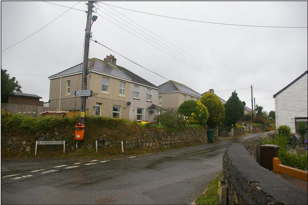
25. DETAIL OF THE SETTLEMENT OF CARLEEN WITHIN THE WHS MINING AREA, SHOWING 20 TH CENTURY HOUSING OF TREGONNING TERRACE; VIEWED FROM THE EAST-SOUTH-EAST.
