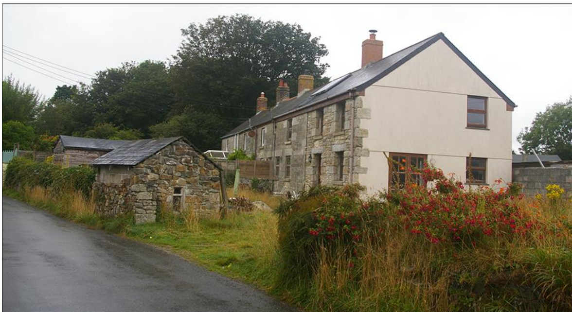
FIGURE 22: THE TRADITIONAL MINERS COTTAGES OF GILBERTS ROW, CARLEEN; VIEWED FROM THE EAST.
