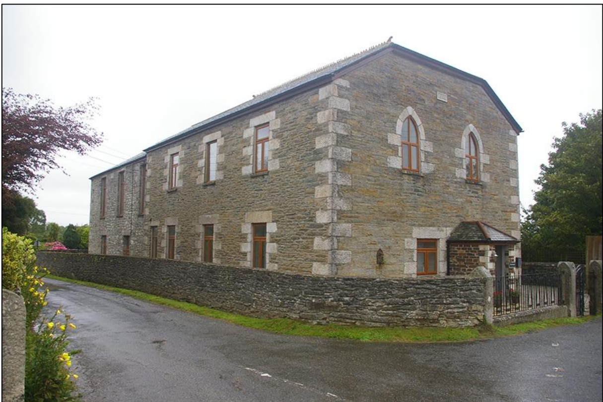
26. DETAIL OF THE SETTLEMENT OF CARLEEN WITHIN THE WHS MINING AREA, SHOWING THE CONVERTED METHODIST CHAPEL; VIEWED FROM THE WEST-NORTH-WEST.
