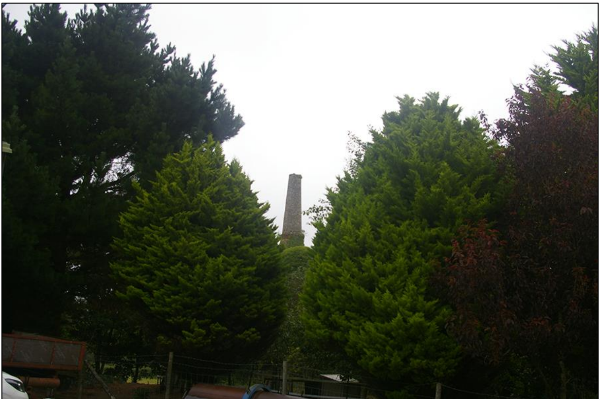
20. THE CHIMNEY WITH THE ENGINE HOUSE AT POLROSE FARM, DEMONSTRATING MAINTAINED WOODLAND SURROUNDING THE MONUMENT; VIEWED FROM THE NORTH-WEST.
