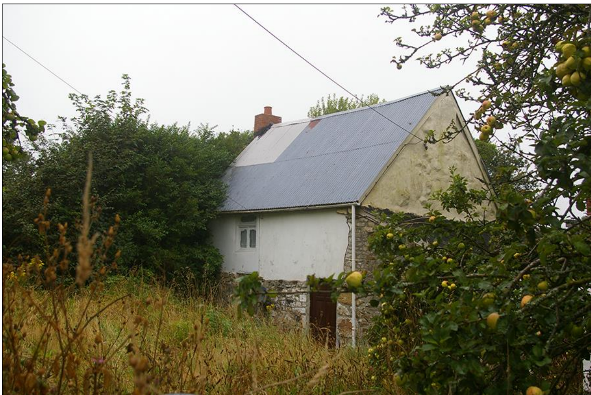
FIGURE 18: MERRIFIELD'S COTTAGE; VIEWED FROM THE EAST-SOUTH-EAST.
