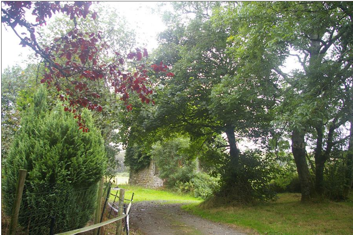
FIGURE 16: THE ENGINE HOUSE AT POLROSE MINES; VIEWED FROM THE SOUTH-WEST.
