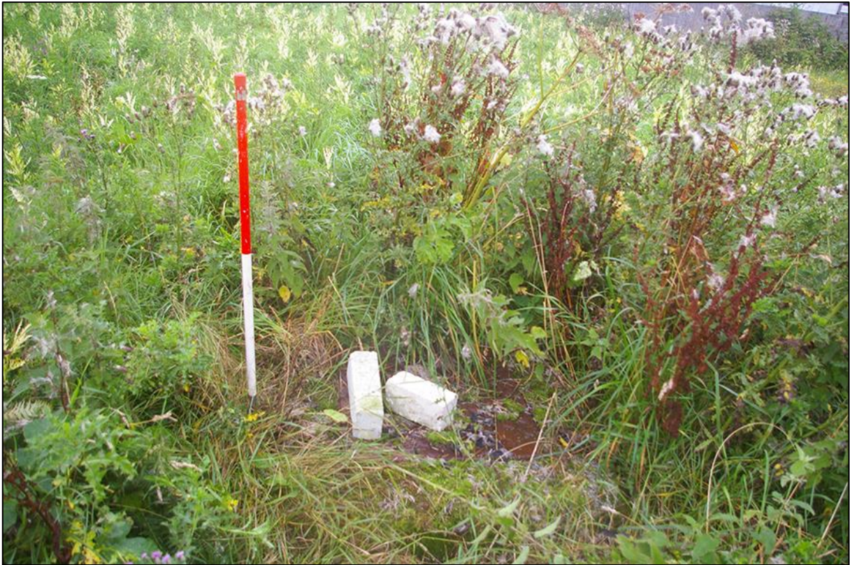
15. DETAIL OF THE MODERN MANHOLE TOWARDS THE SOUTH-EASTERN CORNER OF THE SITE; VIEWED FROM THE SOUTH (1M SCALE).
