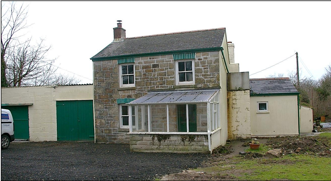
FIGURE 9: FRONT ELEVATION OF THE PROPERTY, VIEWED FROM THE SOUTH.
