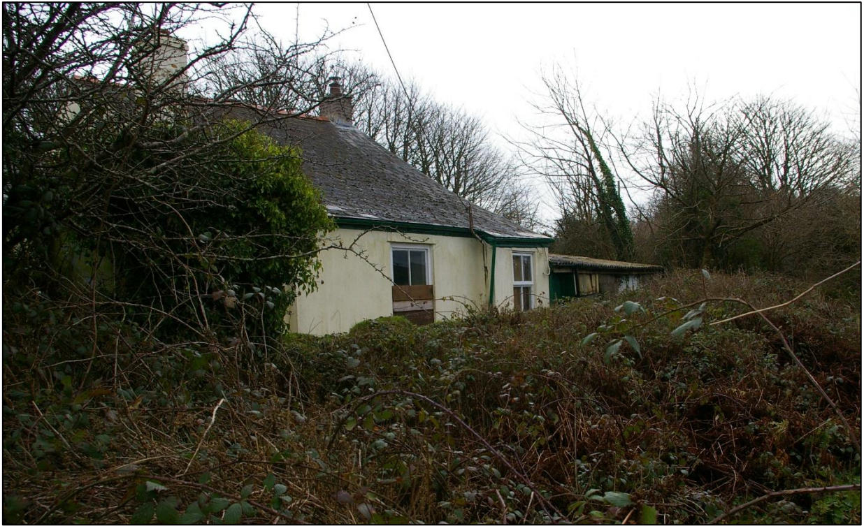
FIGURE 11: NORTHERN ELEVATION OF THE PROPERTY AS VISIBLE FROM THE LANE TO THE EAST OF THE HOUSE, VIEWED FROM THE NORTH-EAST.
