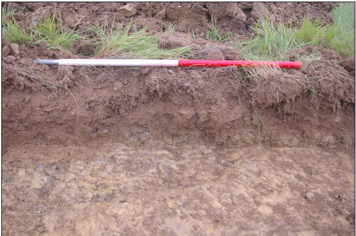
8. DRAIN/GULLY [205] SLOT 1, WEST FACING TRENCH SECTION; VIEWED FROM THE WEST (1M SCALE).
