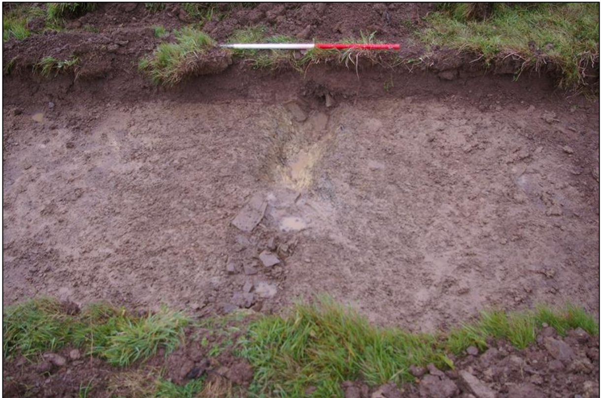
20. DRAIN [308], POST-EXCAVATION; VIEWED FROM THE WEST (1M SCALE).
