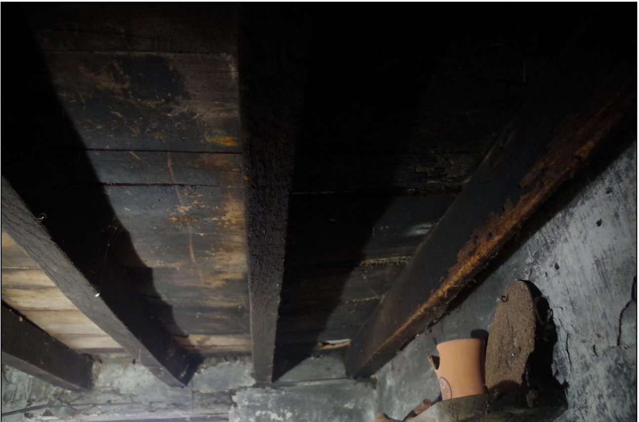
26. THE SMOKE-BLACKENED FLOORBOARDS SURROUNDING FIREPLACE; VIEWED FROM BELOW.
