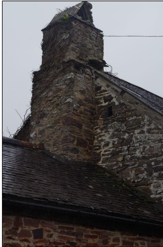
33. THE CHUNKY STEPPED STACK OF B5; VIEWED FROM THE SSE.
