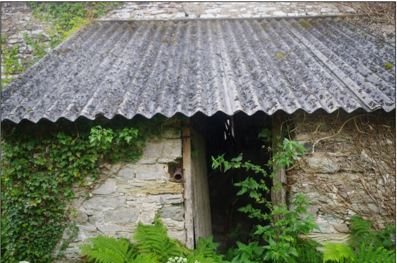
16. ENTRANCE TO B3 FROM THE PRIVY; VIEWED FROM THE W.
