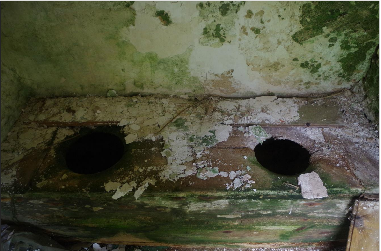
13. BOXED TIMBER IN DOUBLE PRIVY, STONE DRAIN BELOW; VIEWED FROM ABOVE.
