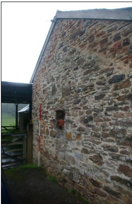
FIGURE 17: THE SOUTH GABLE OF B6, WITH CLEAR BUILD LINE AT ROOF AND 2M SCALE; FROM THE EAST-SOUTH-EAST.
