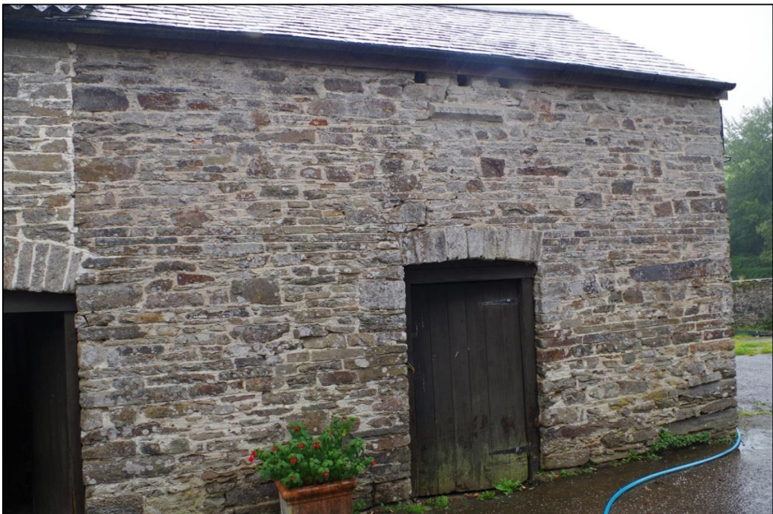
FIGURE 14: B4 SHOWING DATE STONE AND DOVEHOLES TO THE EAVES.
