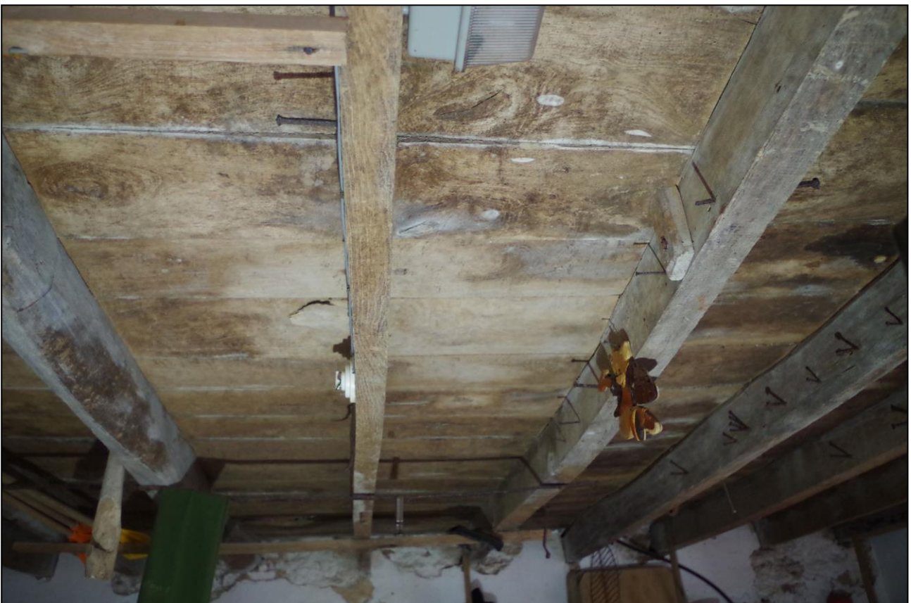
20. INTERIOR FLOOR JOISTS OF B4; VIEWED FROM BELOW.
