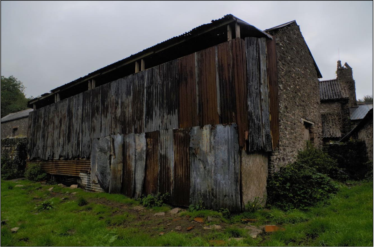
7. B1 WESTERN ELEVATION SHOWING TIN CANOPY; VIEWED FROM THE SW.
