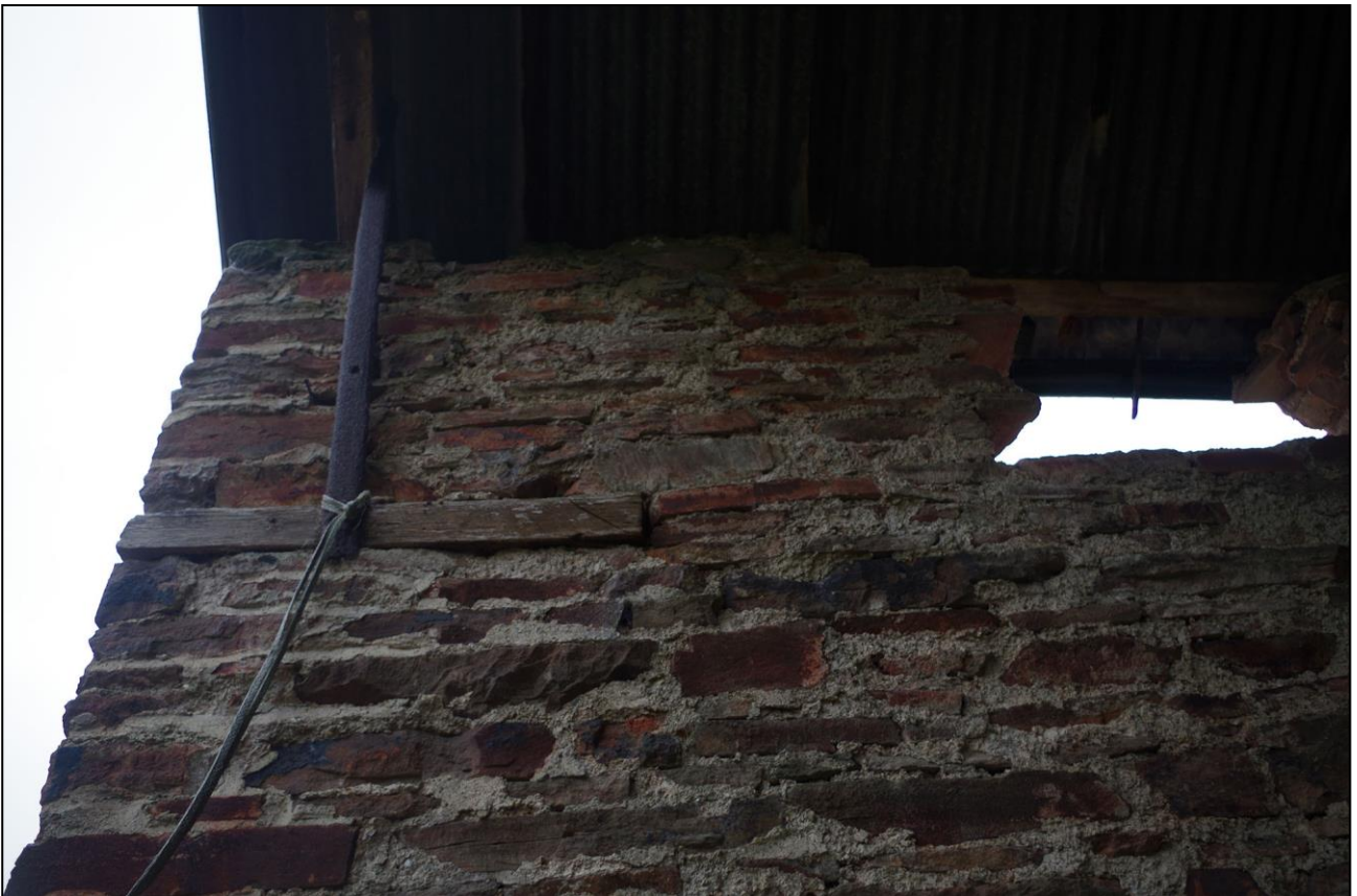
6. B1 IRON ROOF STRAP SUPPORTS ON TIMBER STRAPS; VIEWED FROM BELOW.
