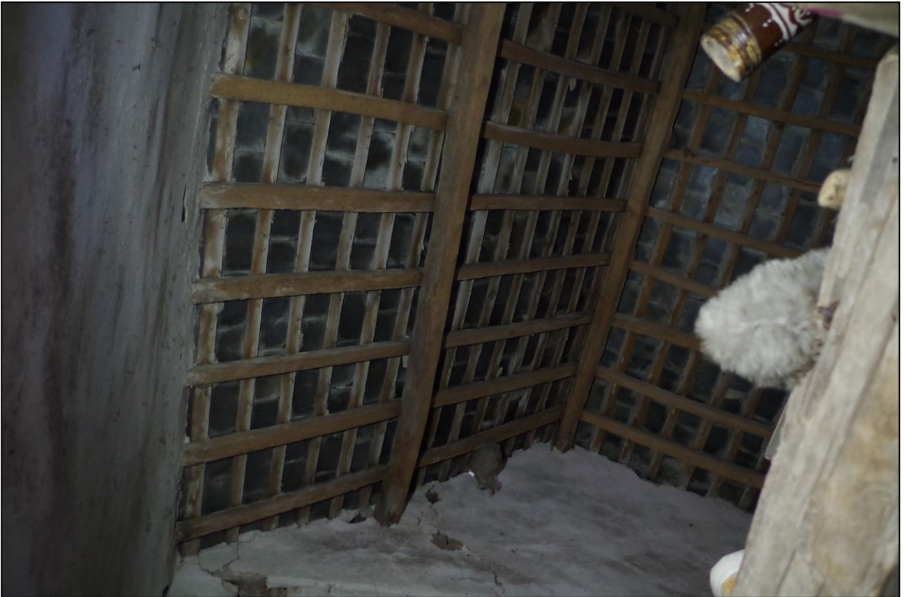
21. B4 INTERNAL VIEW OF ROOF STRUCTURE; VIEWED FROM BELOW.
