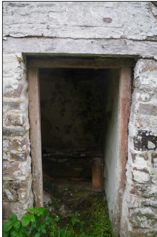
12. ENTRANCE TO DOUBLE PRIVY B2; VIEWED FROM THE E.
