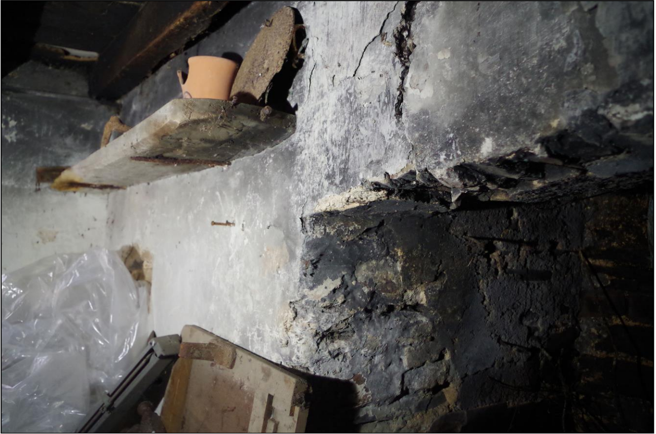
25. THE SHELVING INTACT NEXT TO THE FIREPLACE; VIEWED FROM THE WNW.
