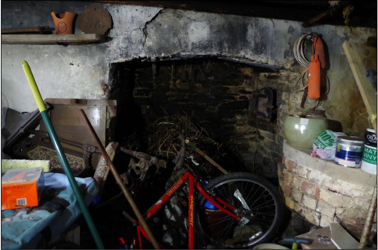
FIGURE 18: FIREPLACE AND COPPER IN B5.
