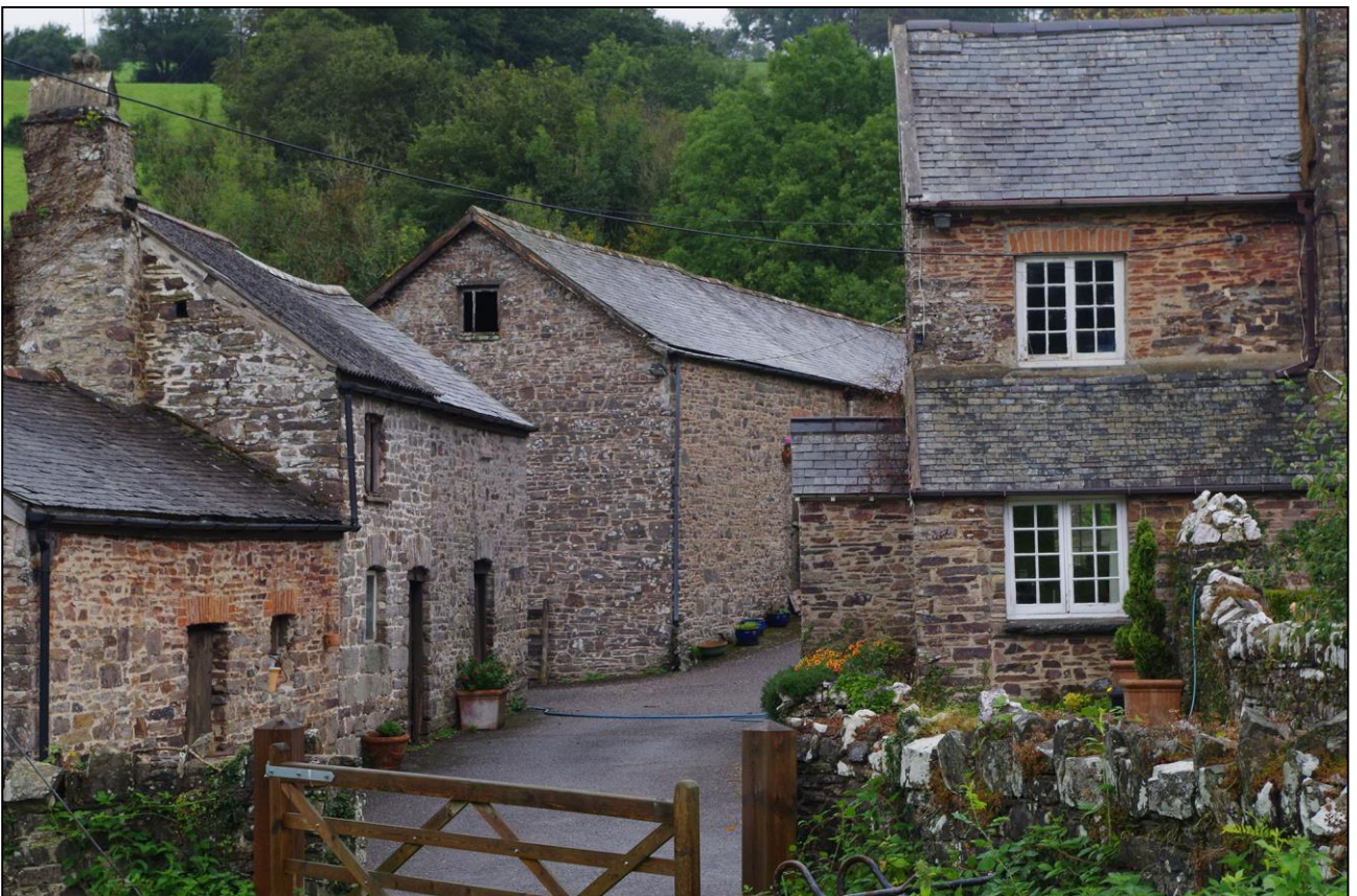
46. THE BARNS AND RELATIONSHIP WITH THE HOUSE, LOOKING UP TO THE BANK BARN; VIEWED FROM THE S.
