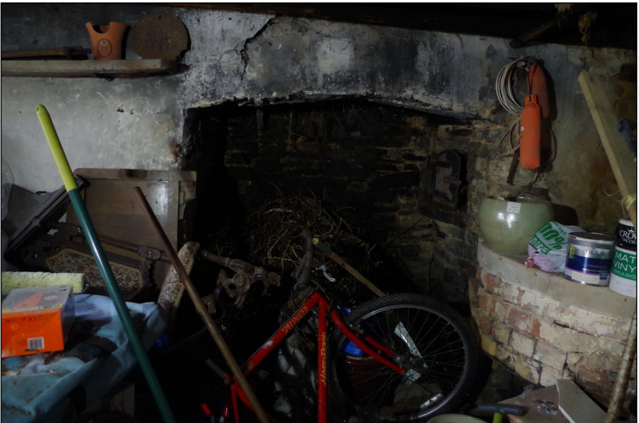
24. THE TUDORESQU ARCH TO THE FIREPLACE IN B5 WITH COPPER BASIN STRUCTURE TO THE RIGHT; VIEWED FROM THE N.
