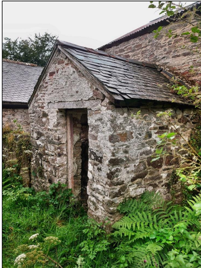
FIGURE 13: THE GRADE II LISTED PRIVY BUILDING; FROM THE NORTH-EAST.
