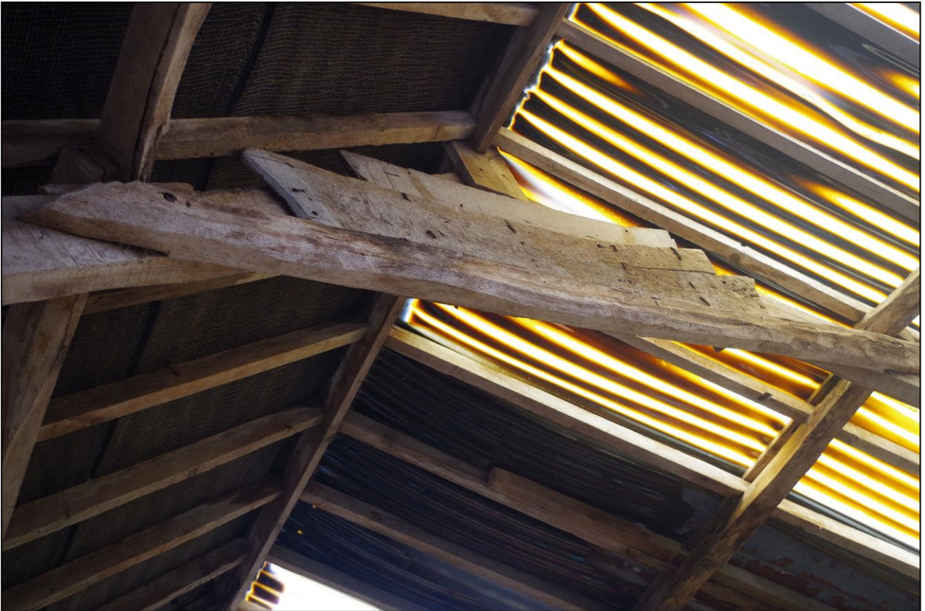
37. THE ROOF TRUSS IN B6; VIEWED FROM BELOW.
