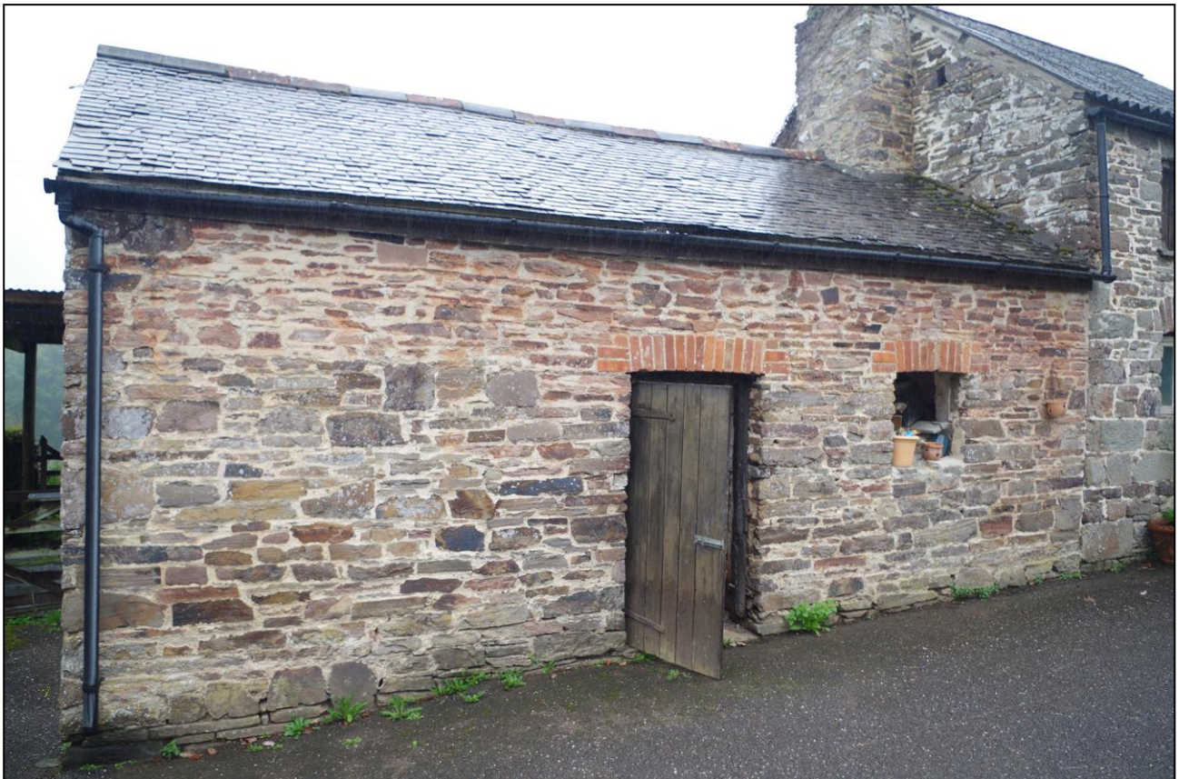
34. THE EAST ELEVATION OF B6, SANDSTONE RAISE IS VISIBLE; VIEWED FROM THE SSE.
