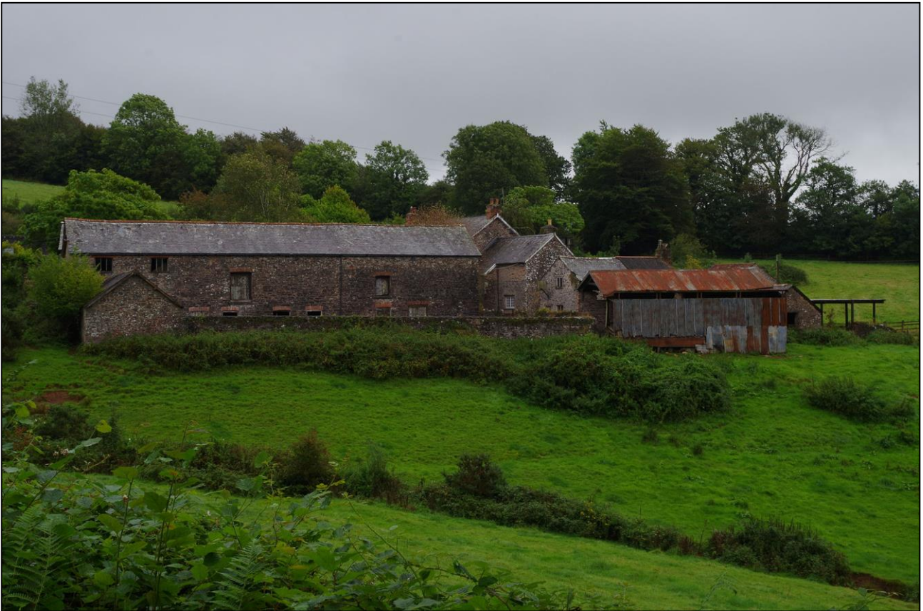
1. THE BARNs AS VIEWED FROM THE DRIVE; VIEWED FROM THE WNW.
