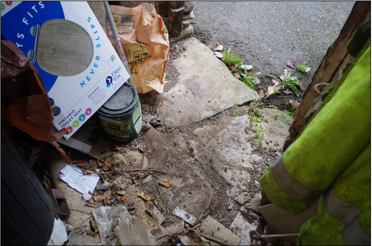
39. THE GOOD FLAGSTONE HEARTH TO B6; VIEWED FROM ABOVE.
