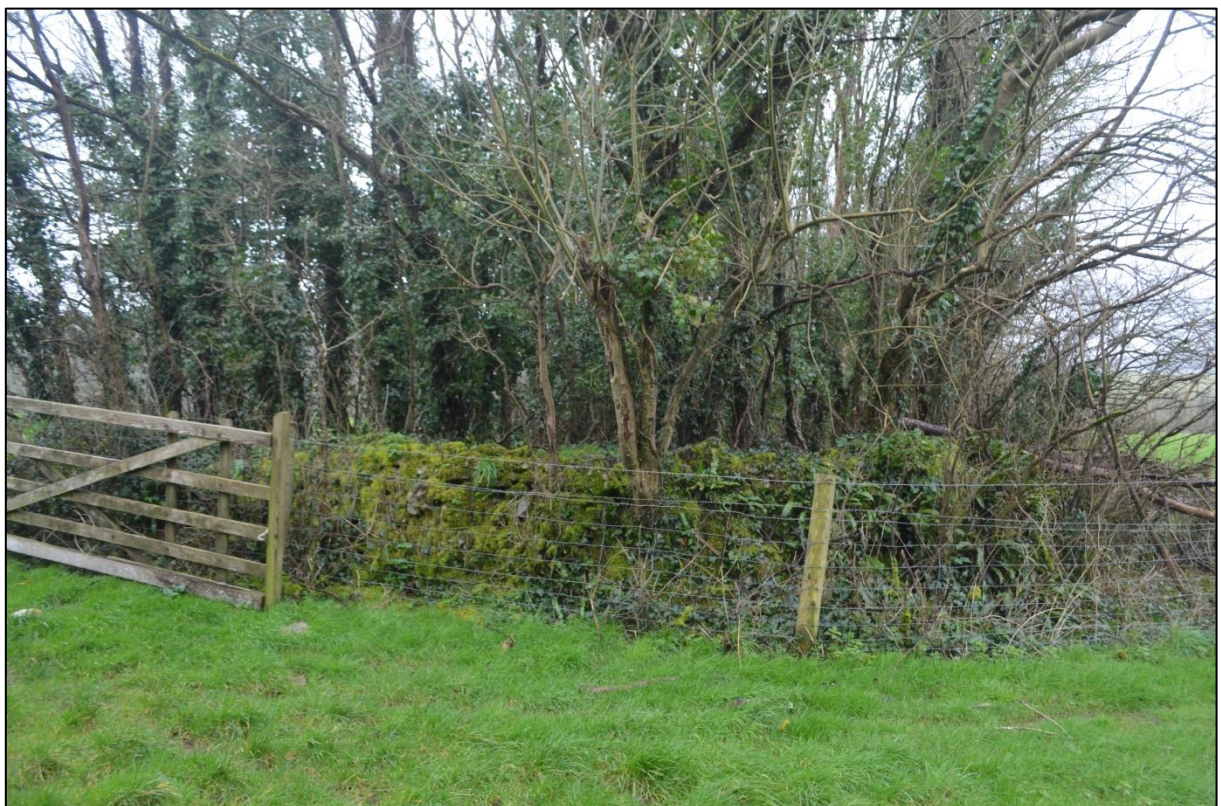
FIGURE 93: STONE FACED BANK WITH MODERN FENCING ON THE EASTERN END OF THE WESTERN SECTION OF WIXENFORD BRAKE. FROM THE EAST.
