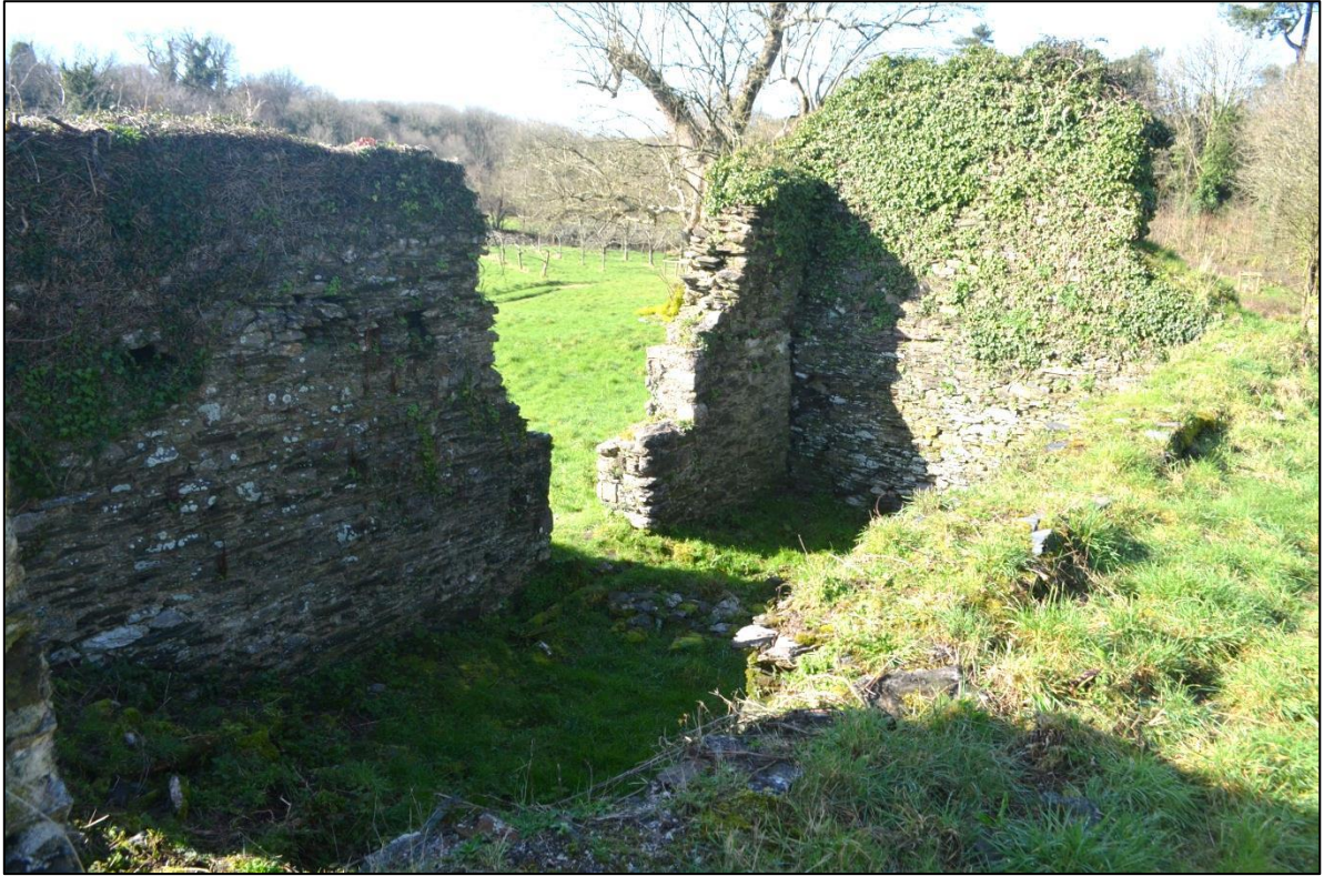
FIGURE 76: THE INSIDE OF BICKHAM BARN; FROM THE NORTH EAST
