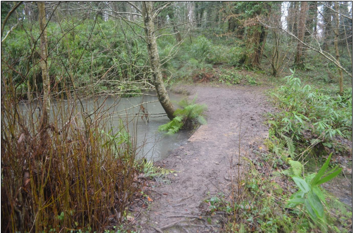
FIGURE 62: DAM/BRIDGE AT THE SOUTHERN END OF POND 2; FROM THE WEST
