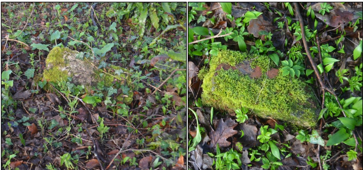
FIGURE 32: BLOCKS OF CONCRETE AND BRICK WERE OBSERVED AMONG THE VEGETATION ON THE SURFACE OF THE TWO POSSIBLE FEATURES OPPOSITE THE PATH INTO THE DELL.
