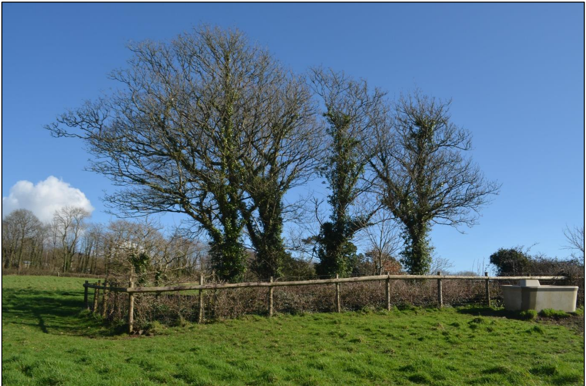
FIGURE 68: PHOTOGRAPH OF BICKHAM CLUMP, FROM THE WEST.
