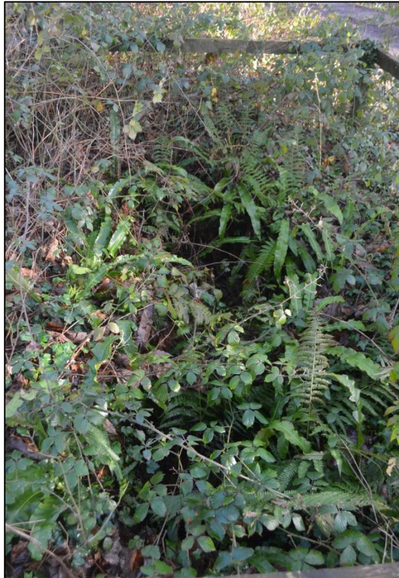
FIGURE 45: FENCED OFF CUT FEATURE TO THE WEST OF THE MAIN PATH THROUGH THE DELL; FROM THE SOUTH
