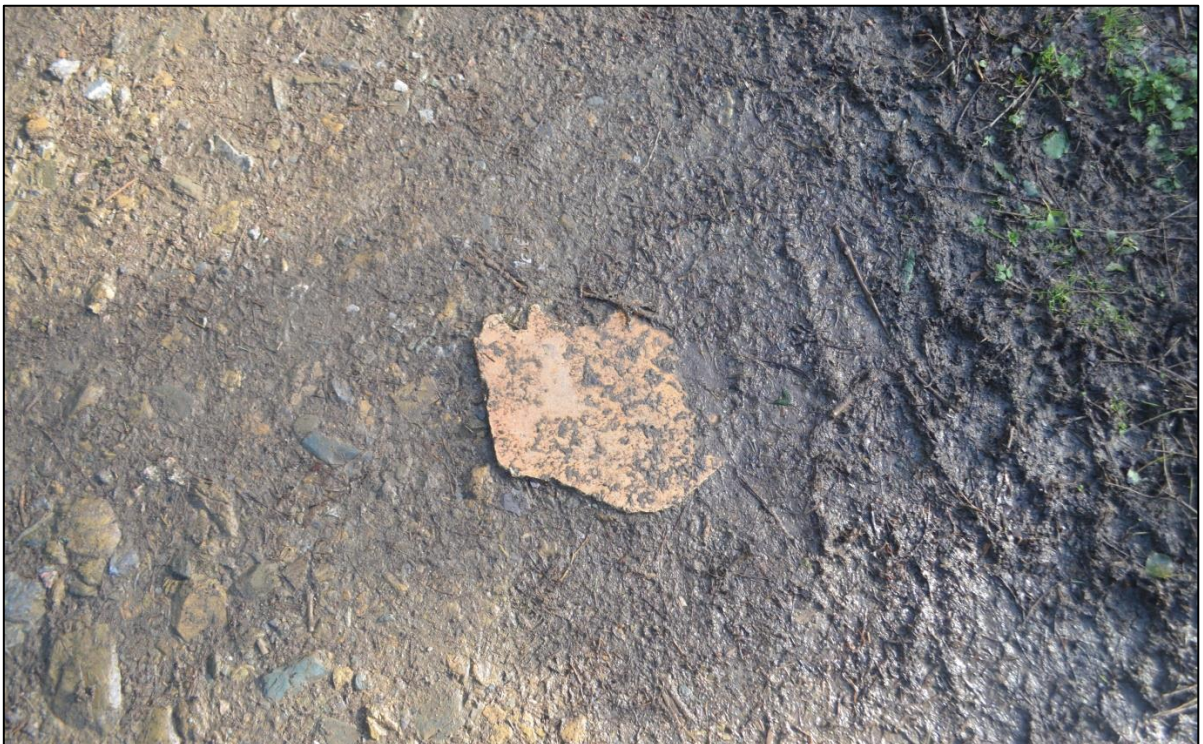
FIGURE 54: OCCASIONAL ROOF TILES APPEAR TO HAVE BEEN BUILT INTO THE PATH SURFACE
