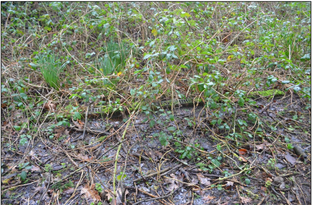
FIGURE 40: CONCRETE PLATFORM WITH 1 BRICK HIGH SURVIVING EDGING IN SOME AREAS; FROM THE EAST
