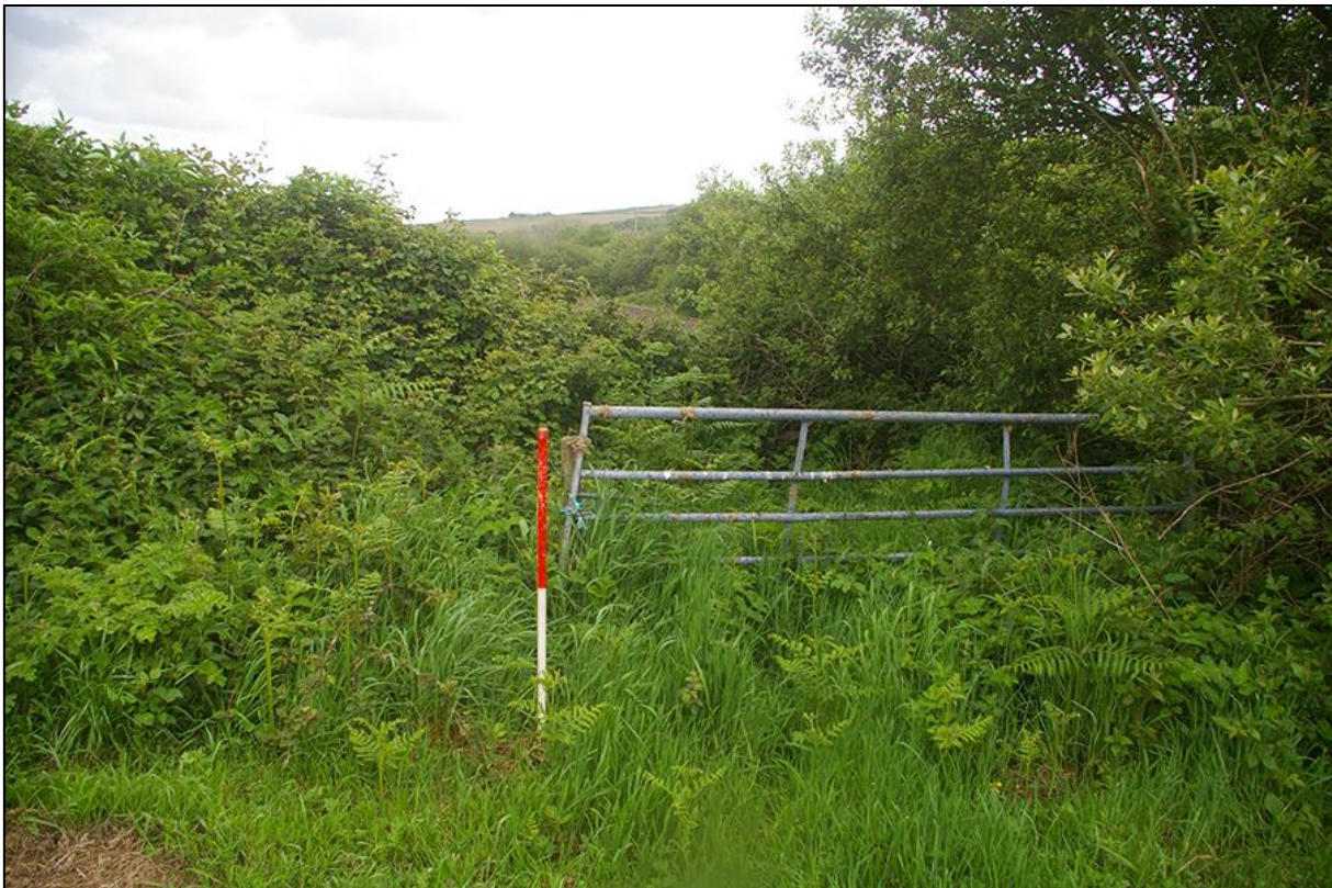
32. F2, DETAIL OF THE GATED ACCESS AT THE SOUTH-WESTERN END OF THE SOUTH-EASTERN BANK BOUNDARY; VIEWED FROM THE NORTH-WEST (1M SCALE).
