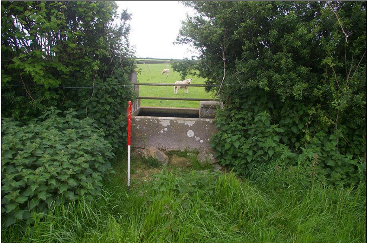
12. F1, DETAIL OF THE STONE TROUGH IN THE BREACH MID-WAY ALONG THE SOUTH-WESTERN HEDGEBANK BOUNDARY; VIEWED FROM THE NORTH-EAST (1M SCALE).
