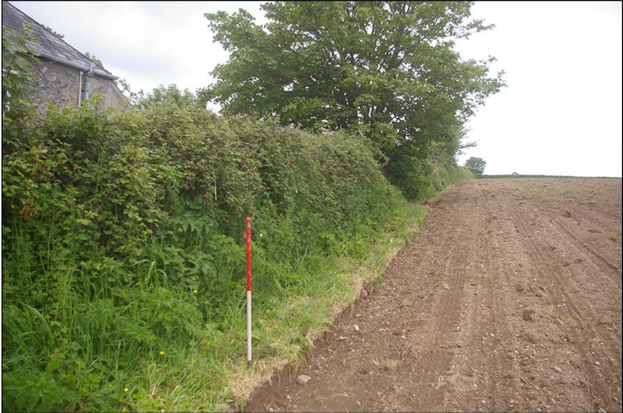
35. F2, DETAIL OF THE SOUTH-WESTERN HEDGEBANK BOUNDARY NORTH OF PENHALLOW HOUSE; VIEWED FROM THE EAST (1M SCALE).
