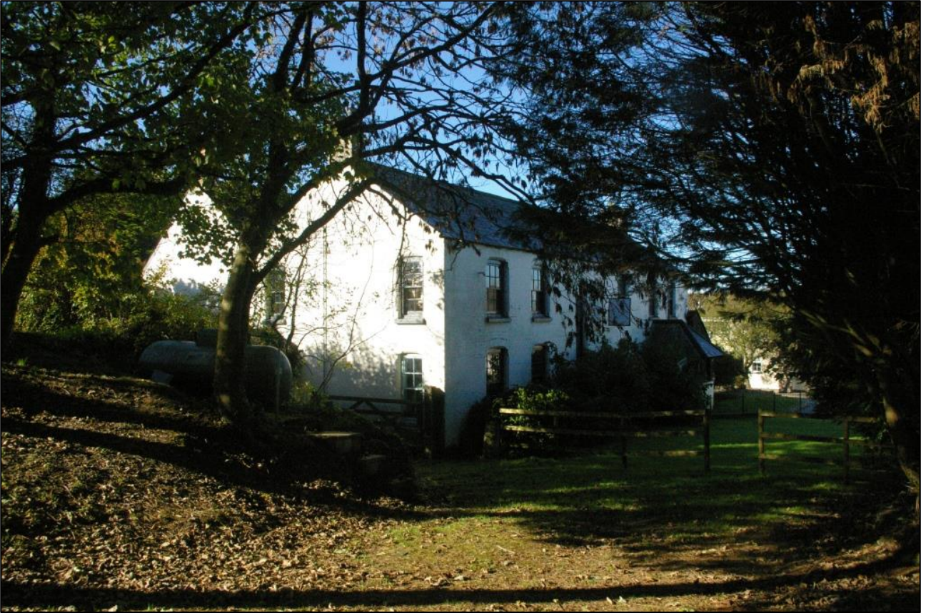
5. THE REAR OF THE FORMER FARMHOUSE WITHIN ITS ENCLOSED GARDEN SETTING, WITH BY OIL TANK, IRON RAILINGS AND VARIOUS SECTIONS OF FENCING DIVIDING OFF AREAS OF THE PUB GARDENS; VIEWED FROM THE EAST.
