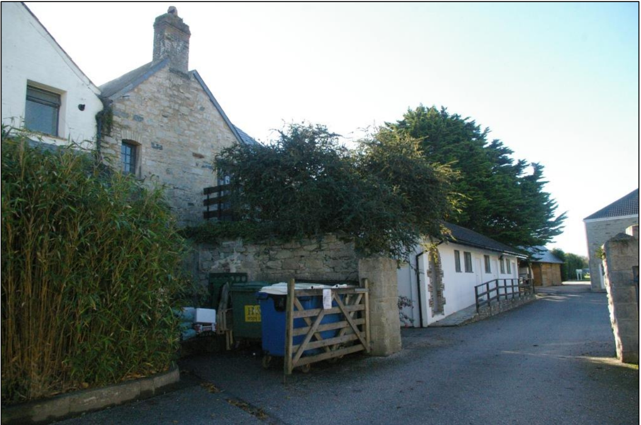
3. VIEW OF THE FORMER FARMHOUSE AND ADJACENT SERVICE BUILDINGS, INCLUDING LAUNDRIES; VIEWED FROM THE NORTH.
