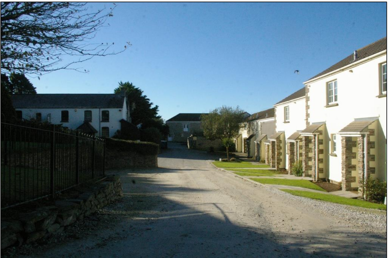
2. VIEW OF THE TERRACED HOLIDAY COTTAGES AND REAR ELEVATION OF THE FORMER FARMHOUSE (LEFT), SHOWING ITS ENCLOSED AND CROWDED SETTING; VIEWED FROM THE NNE.
