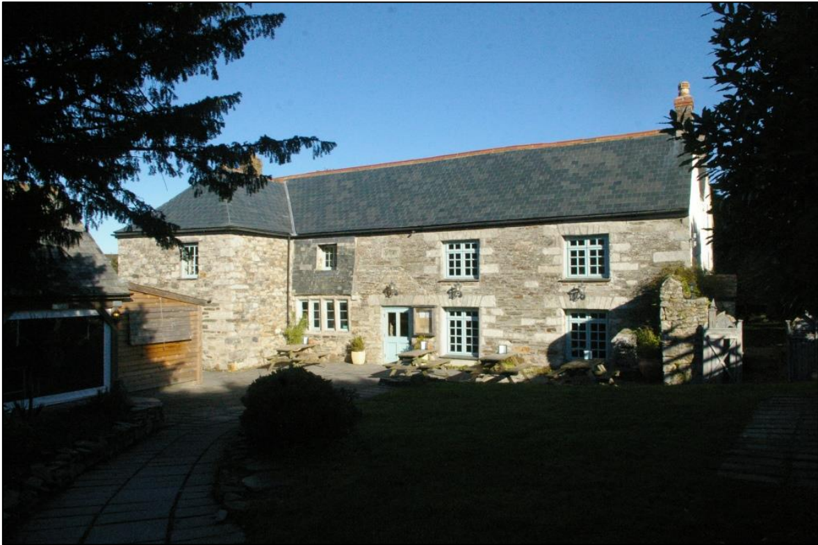
FIGURE 10: VIEW OF CARVYNICK HOUSE WITHIN ITS ENCLOSED PUB GARDEN SETTING. THE EXTREME SHADOWS EVIDENCE THE LOOMING HEDGES THAT ENCLOSE IT, SCREENING OUTWARD VIEWS; VIEWED FROM THE SOUTH (2018 PHOTO).
