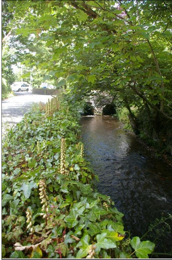
5. The canalised river in the centre of the village; from the east.
