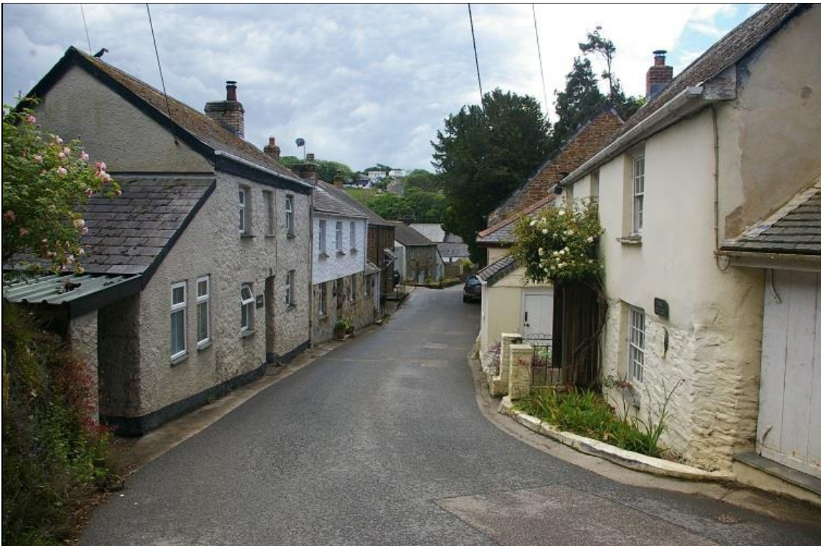
20. The post medieval settled core to the north of the conservation area, with narrow street lined with small cottages, centred around a nonconformist chapel; from the north.
