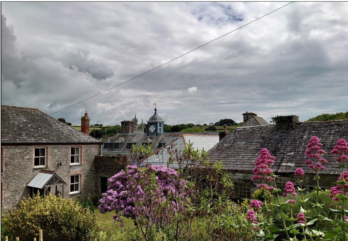
18. View across and into the walled convent site, showing a cluster of tightly packed building and few outward views, although there are historic dormers at roof height and they will have landscape-valley views; from the south-west.
