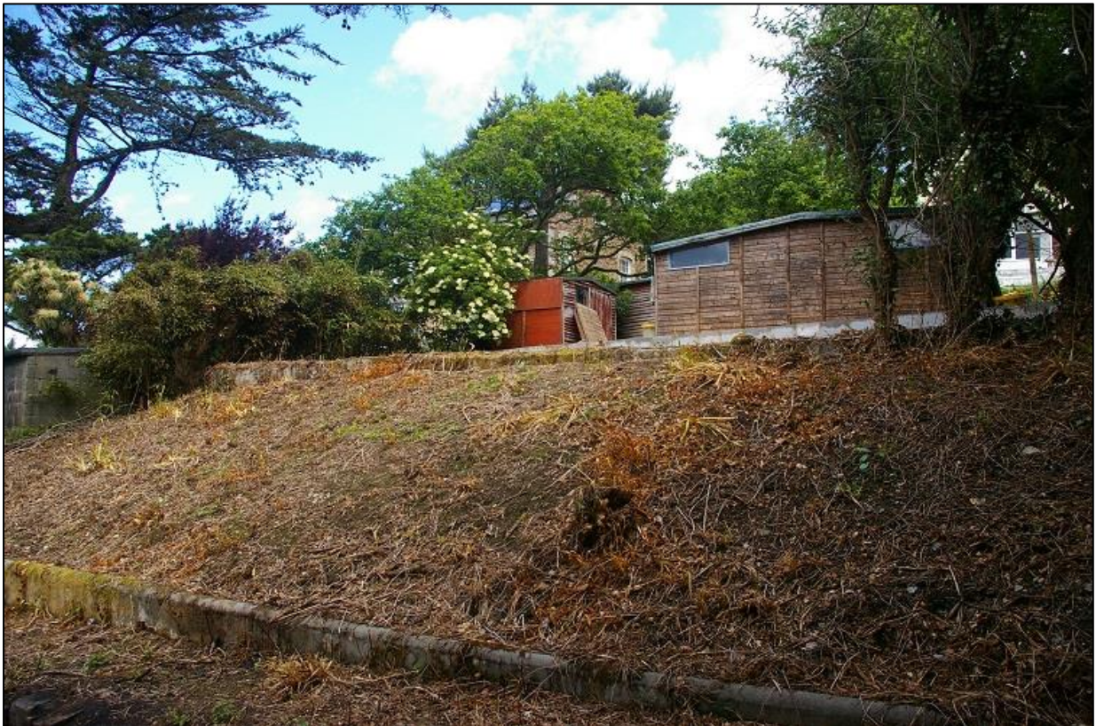
FIGURE 10: THE UPPER TERRACED AREA, WITH SOME CONCRETE KERB STONES AND BLOCKS FORMING RETAINING BANKS; FROM THE SOUTH-EAST.
