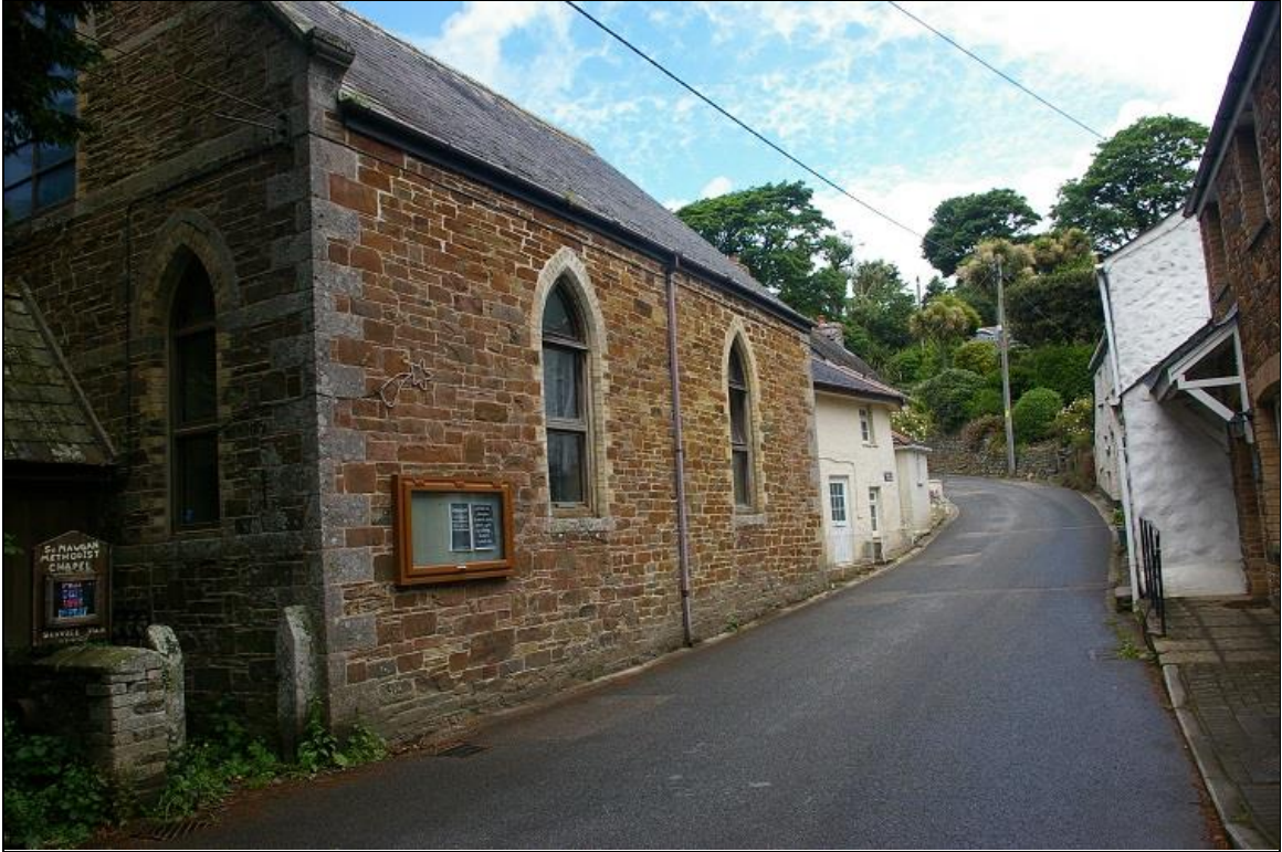
21. The nonconformist chapel in the post medieval core of the village to the north of the river; from the south-east.
