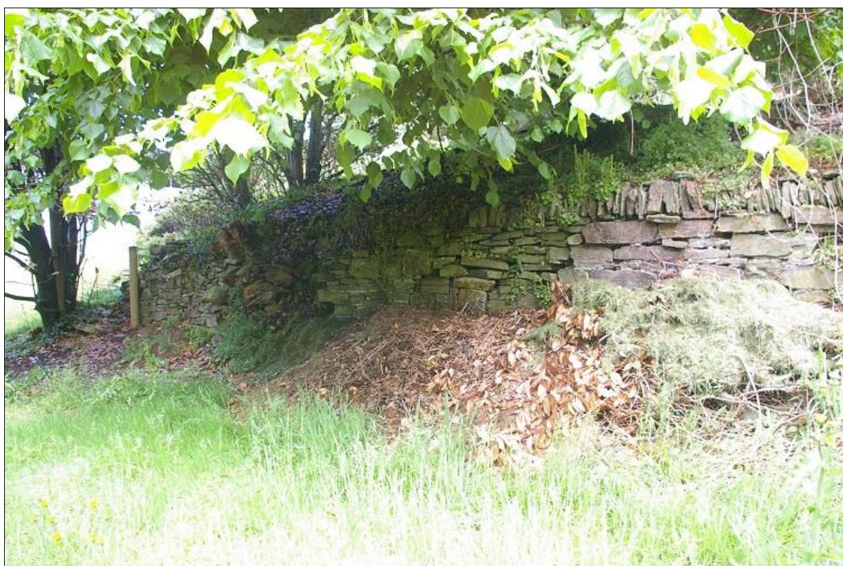
FIGURE 13: DETAIL OF THE STONE WALL, LIKELY A 19TH CENTURY FEATURE; FROM THE EAST-SOUTH-EAST.
