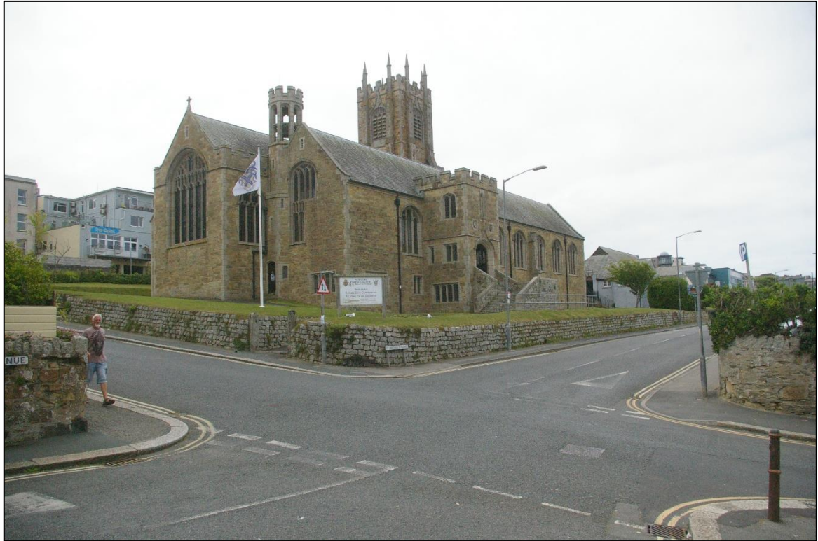
1. ST. MICHAELS CHURCH, VIEWED FROM THE SOUTH-EAST.
