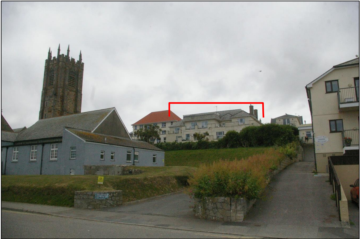
FIGURE 14: ST MICHAEL'S CHURCH AND CHURCH HALL VIEWED FROM ST. MICHAEL'S ROAD, PRIORY LODGE IS INDICATED (FROM THE NORTH-NORTH-EAST).
