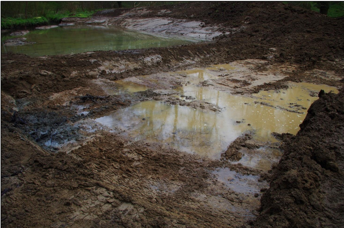
FIGURE 4. MIDWAY THROUGH DE-SILTING: HALF OF THE EXCAVATED AREA HAS ALREADY BEEN FLOODED. THE DARKER AREA TO THE LEFT OF THE IMAGE INDICATES LOCATION OF A PREVIOUS TREE. VIEWED FACING NORTH-WEST.
