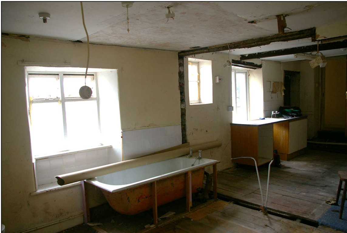
45. LONG VIEW DOWN THE EAST WALL OF ROOM 20; FROM THE NORTH-WEST.
