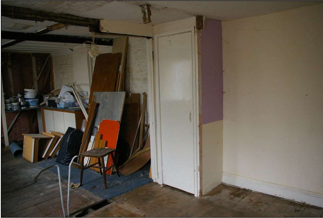
50. THE LONG WEST WALL OF ROOM 20; FROM THE NORTH-EAST.
