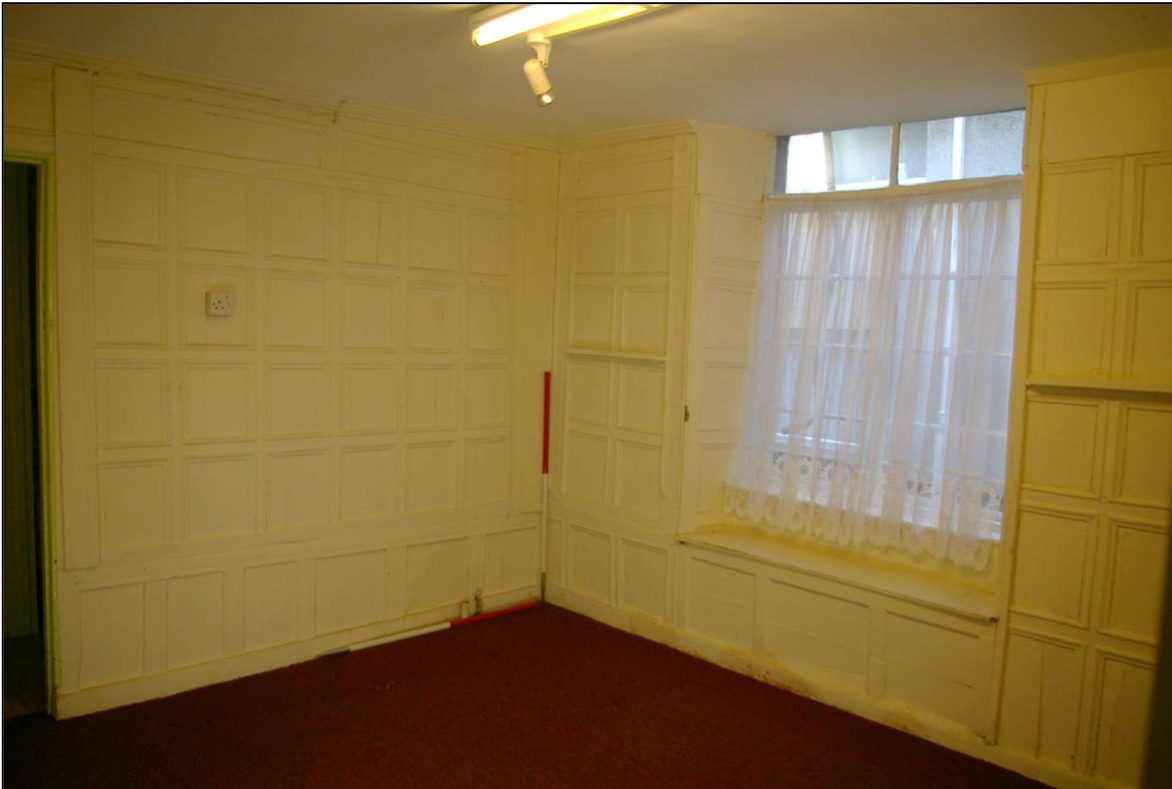
53. THE NORTH AND EAST WALL, WITH 1M SCALE; FROM THE SOUTH-WEST.
