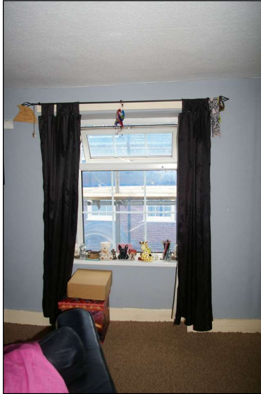
28. THE PVC SASH EFFECT MODERN WINDOW FITTED TO THE WESTERNMOST WINDOW IN THE FRONT WALL OF THE SECOND FLOOR LEVEL, ROOM 15; FROM THE NORTH, NORTH-WEST.
