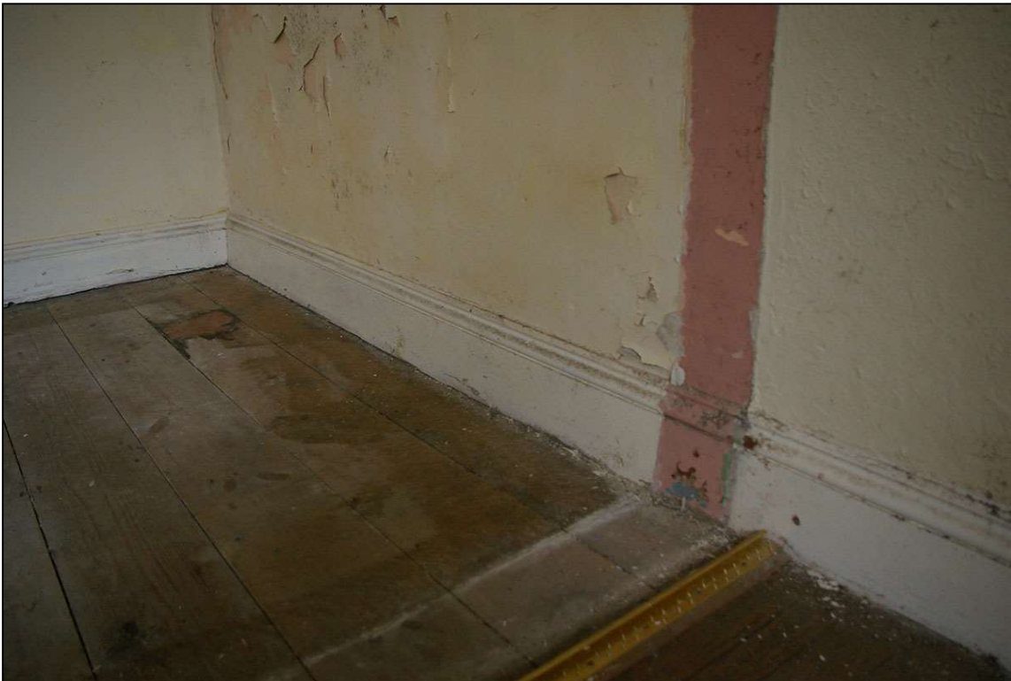
51. THE BEADED SKIRTING, IN ROOM 20, VICTORIAN IN STYLE WHICH RUNS ALONG THE WEST AND NORTH WALLS OF BR4; FROM THE EAST.
