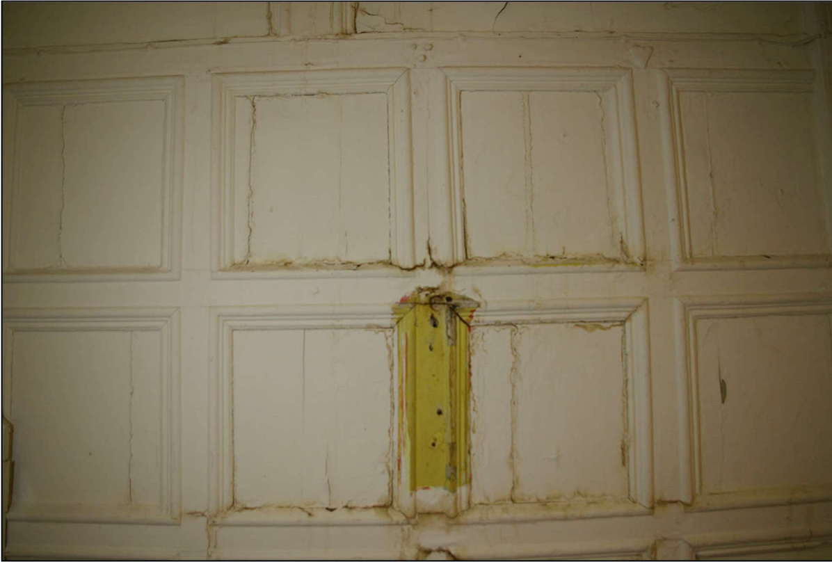
79. LAYERS OF HISTORIC PAINTWORK, SHOWING A DEEP PINKISH TERRACOTTA, A CHARTREUSE AND THE EARLIEST, A FOREST GREEN, ALL UNDER THE THICK MODERN CREAM EMULSION; FROM THE NORTH.
