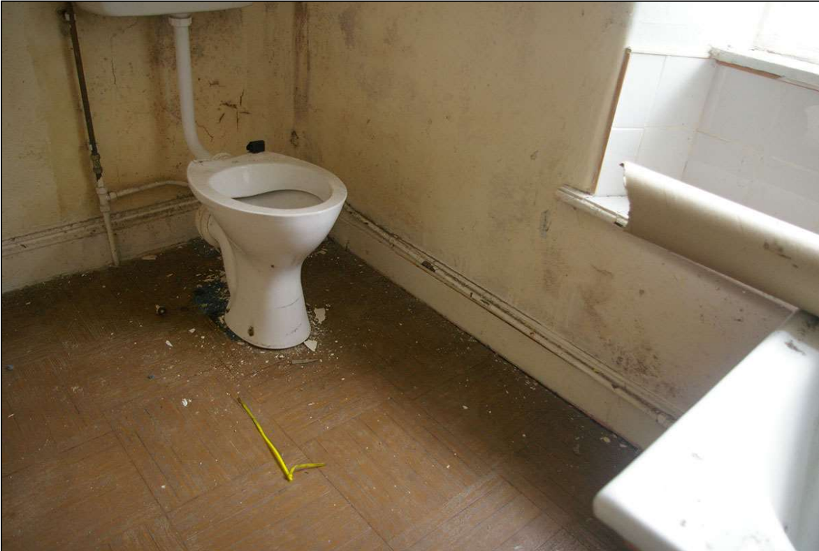
52. R20, THE BEADED SKIRTING RUNS BEHIND, AND IS CUT BY, THE MID-20 TH CENTURY TOILET SUGGESTING IT MAY BE VICTORIAN OR EDWARDIAN; FROM THE SOUTH-WEST.
