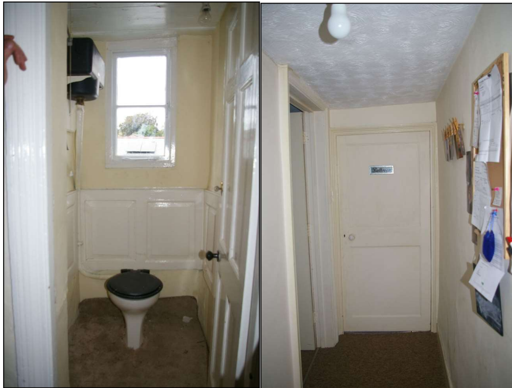
FIGURE 6 A & B: (LEFT) - R11A, THE LONG-DROP TOILET, WITH RESET, 18 TH CENTURY PANELLING AND (RIGHT) - DOOR TO R16 ON THE SECOND FLOOR, ALSO AN 18 TH CENTURY FEATURE.
