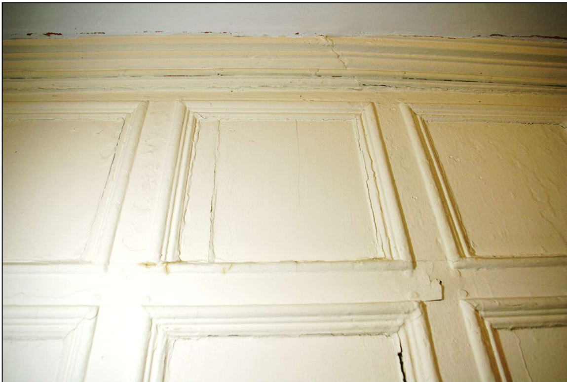
89. DETAIL OF THE TYPE 3 BOLECTION MOULDING; FROM THE EAST.
