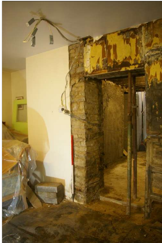
100. THE FRAGMENT OF GOOD HEAVY MEDIEVAL WALLING, WITH FORMAL LEVELLING COURSES — HACKED INTO TO CREATE OPENING, WITH TIMBER TIES INSERTED; FROM THE SOUTH-EAST (1M SCALE).
