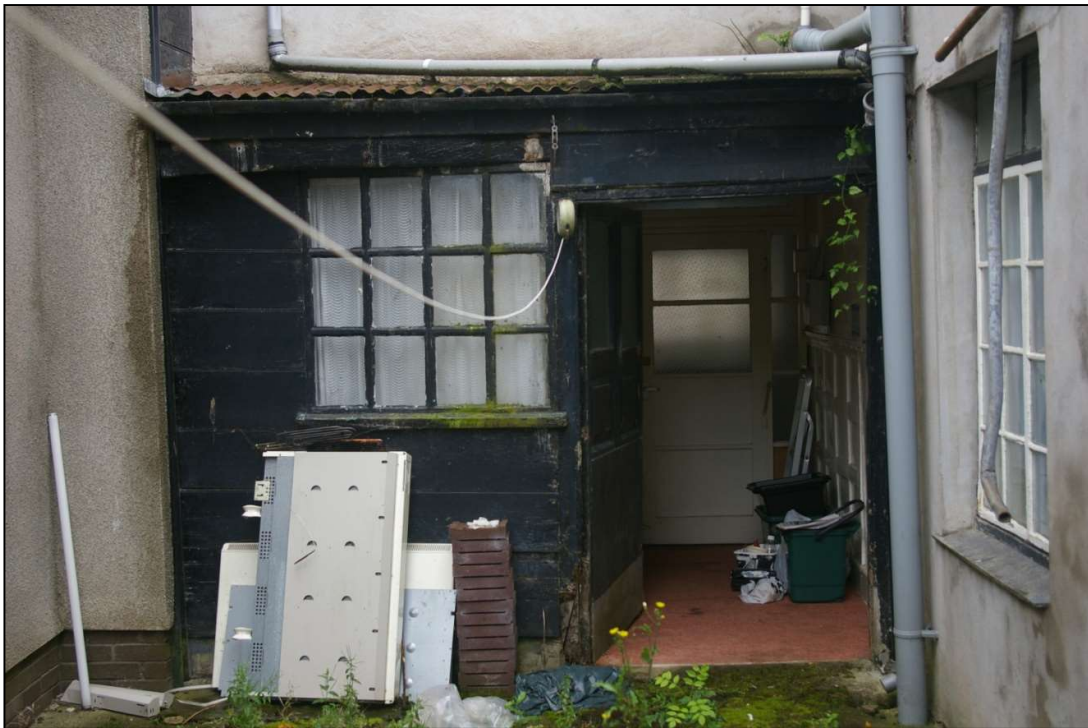
FIGURE 3: THE BEADED PLANK TIMBER STRUCTURE WHICH ENCLOSES THE GROUND FLOOR OF THE REAR ELEVATION; FROM THE NORTH.
