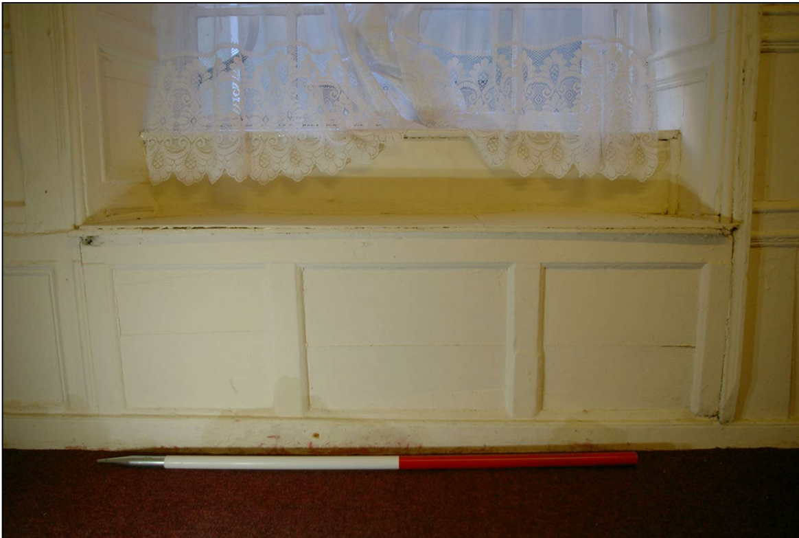
70. THE PANEL UNDER THE WINDOW SEAT AND W13, WITH 1M SCALE, THIS TYPE 9 PANEL IS LIKELY 19 TH CENTURY; FROM THE WEST.
