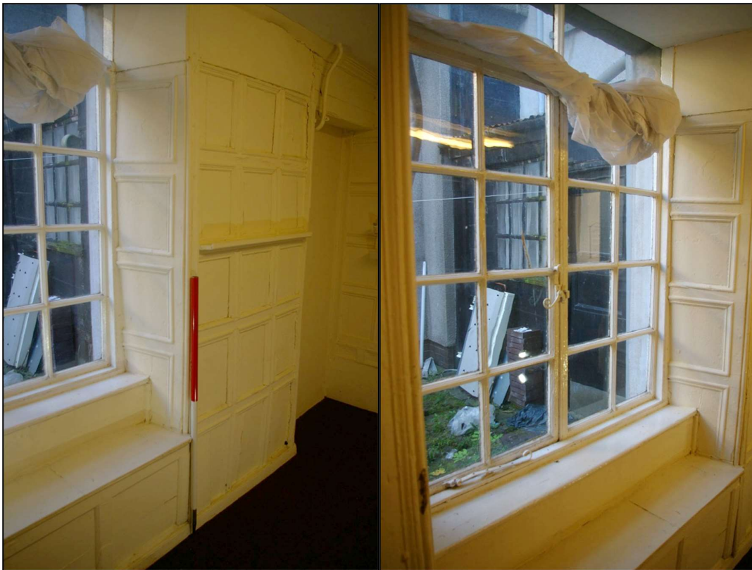
73. LEFT: THE PANELLED SHUTTERS TO THE SOUTH SIDE OF W13, WITH 1M SCALE; FROM THE NORTH-NORTH-EAST.
