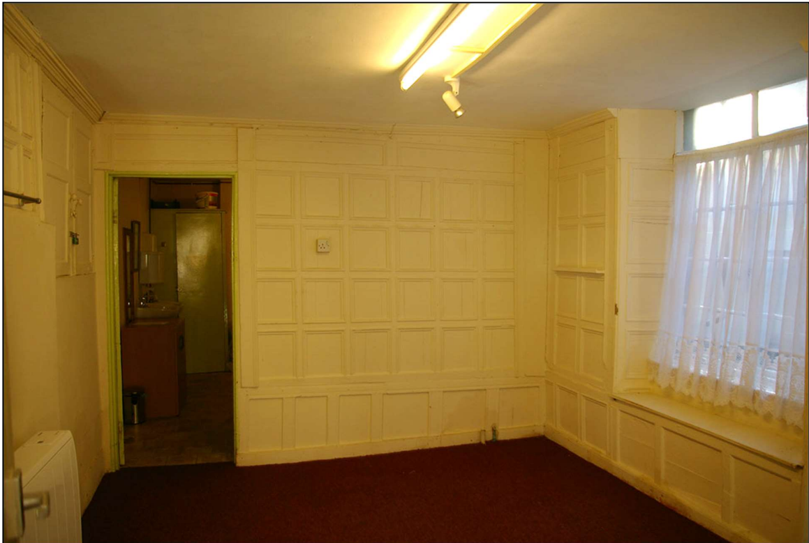
30. R17, SHOWING RESET 17 TH CENTURY PANELLING SECTIONS ON THE WALLS; FROM THE SOUTH-WEST.
