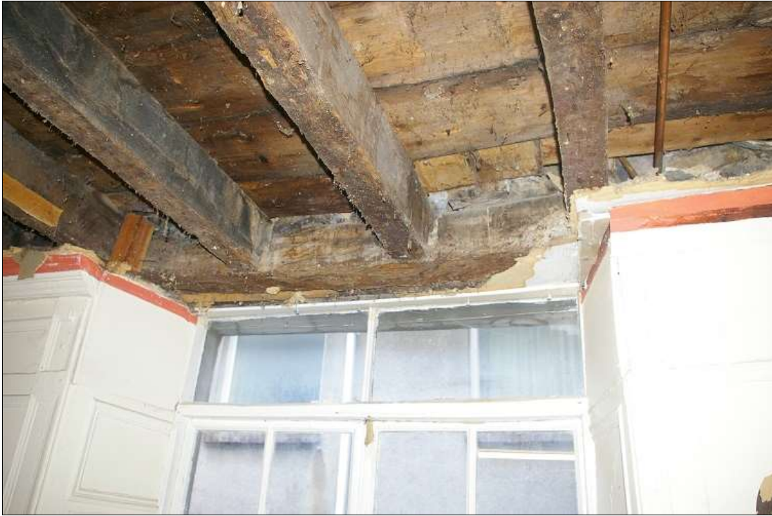
95. CHUNKY 19 TH CENTURY JOISTS AND LINTEL OVER WINDOW, R17 – EVIDENCE OF THE REMODEL OF THIS RANGE; FROM THE WEST.
