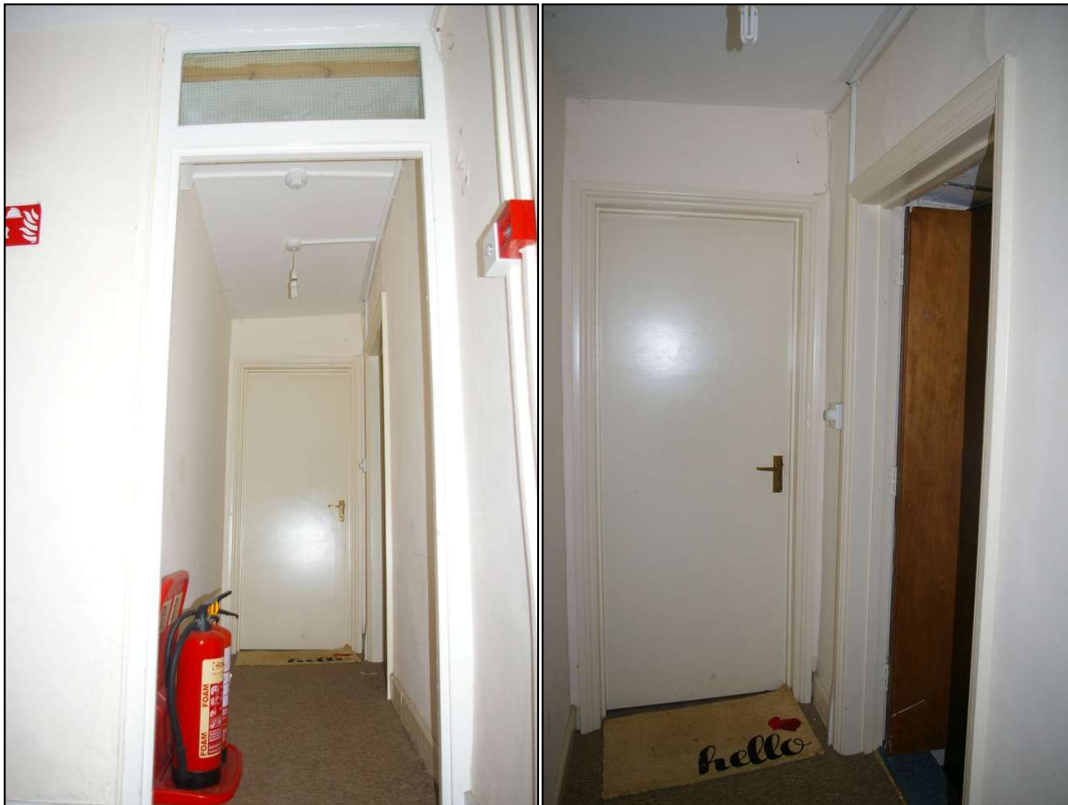
22. LEFT & RIGHT: ROOM 6A, THE SHORT SECTION OF CORRIDOR AND THE FORCED DOOR TO BUILDING 2; FROM THE EAST.
