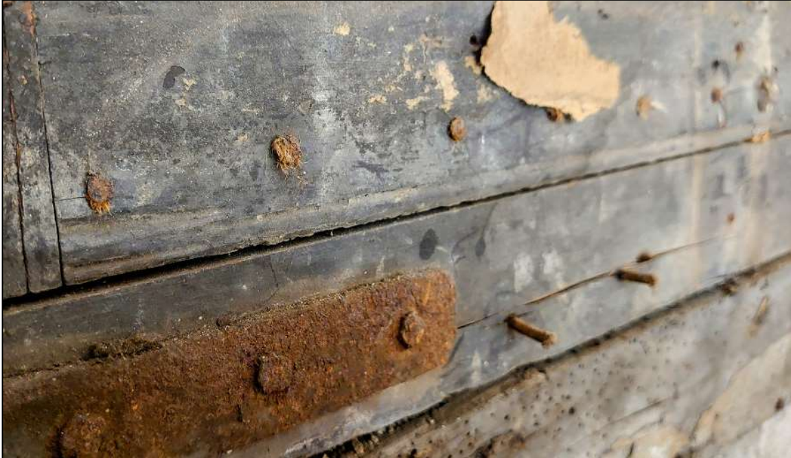
FIGURE 26: ROW OF TACKS AND NAILS, SOME WITH HESSIAN FABRIC ON THEM, SUGGESTING THE BOARDING WAS LATER COVERED WITH FABRIC.
