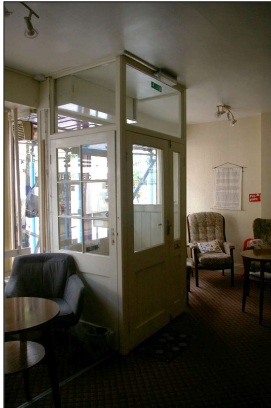
15. THE MODERN PLATE GLASS FACIA OF R2, WITH A RECYCLED COMBINATION OF DOORS AND FRAMEWORK FORMING A SMALL LOBBY; FROM THE EAST-NORTH-EAST.
