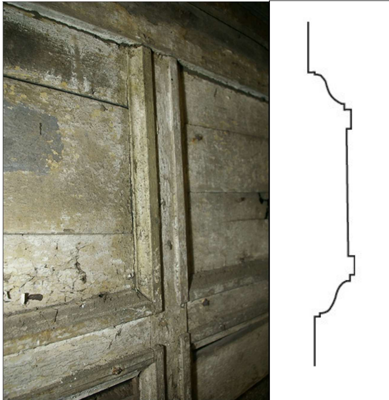
FIGURE 30: PROFILE OF THE OGEE/CAVETTO MOULDINGS ON THE RECYCLED PANELLING IN R2, THE MOULDINGS MAY BE ADDED LATER TO PLAIN STYLES, HENCE WHY THEY ARE PROUD.
