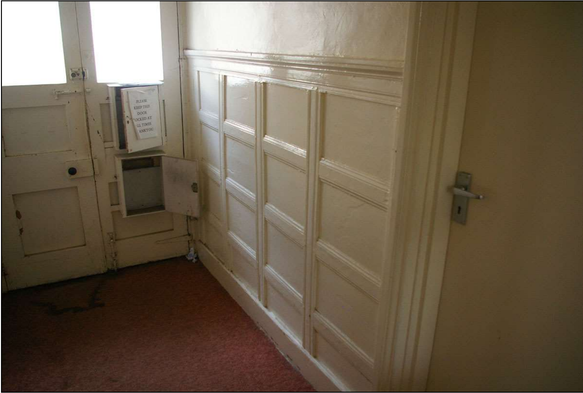
9. FINE 18 TH CENTURY PANELLING, RESET HERE TO THE WEST WALL; FROM THE NORTH-EAST.
