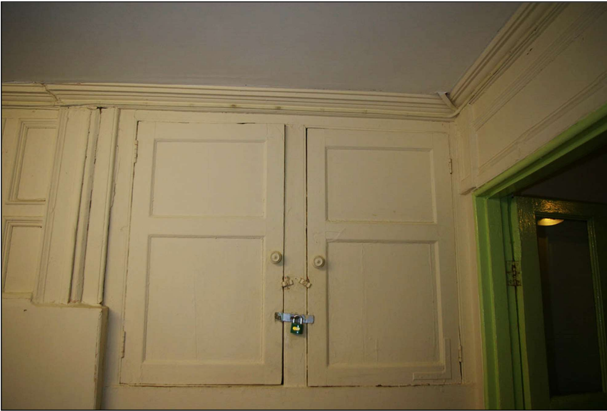
92. THE EARLY 19 TH CENTURY CUPBOARD, TYPE 9 BEADED DOORS; FROM THE EAST.
