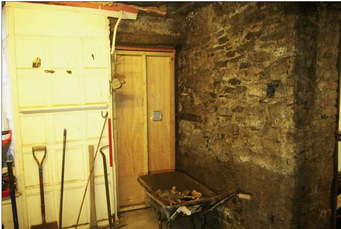
96. VIEW OF THE SOUTH-EAST CORNER OF R17, WHERE THE DOOR TO R1 IS BLOCKED, SHOWING THE EAST AND SOUTH WALL ARE COHESIVE HERE, THE DOOR HOWEVER IS FORCED; FROM THE WEST-NORTH-WEST (1M SCALE).
