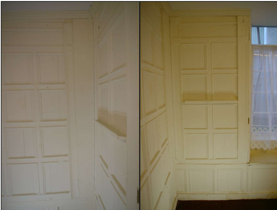
67. LEFT: THE END PILASTER OF THE NORTH WALL TO THE EAST, TYPE 5, WITH PLAIN PLANKS IN THE CORNERS; FROM THE SOUTH.
