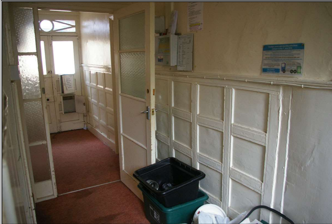
FIGURE 4: VIEW ALONG THE WEST WALL OF R1 AND R1A, SHOWING TWO PHASES OF PANELLING; FROM THE NORTH-EAST.
