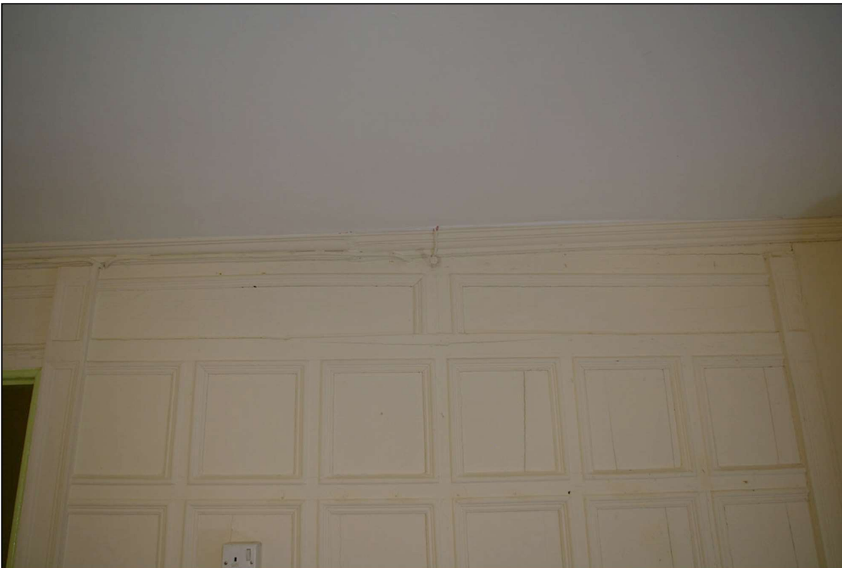
62. THE TYPE 8 TOP PANELS ON THE NORTH WALL; FROM THE SOUTH.
