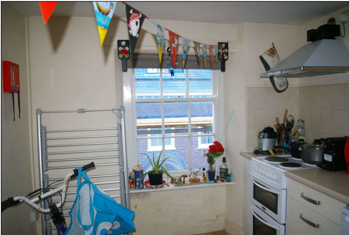
27. THE LATER HORNED SASH WINDOW WHICH LIGHTS THE KITCHEN, R14. ALSO SHOWING AN AWKWARD STEP IN THE WALL, THICKER TO THE WEST AND MAY SUGGEST INFILL BETWEEN BUILDINGS, FURTHER PHASING; FROM THE NORTH.
