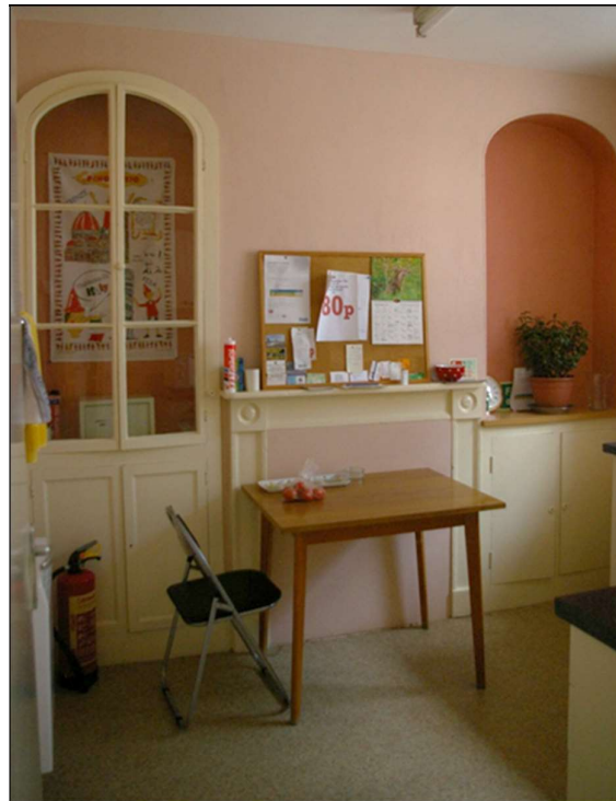
FIGURE 5: THE EAST WALL OF R3, SHOWING CENTRAL FIREPLACE AND TWO BEADED ARCHED ALCOVES, ONE TO NORTH WITH SURVIVING CUPBOARD AND DISPLAY CABINET; FROM THE WEST-NORTH-WEST.
