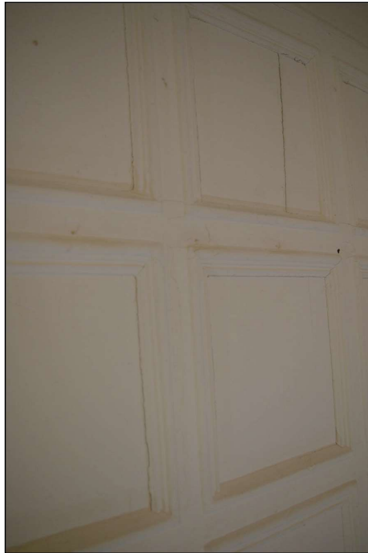
63. DETAIL OF THE BOLECTION MOULDINGS TO THE PANELLING; FROM THE SOUTH-WEST.
