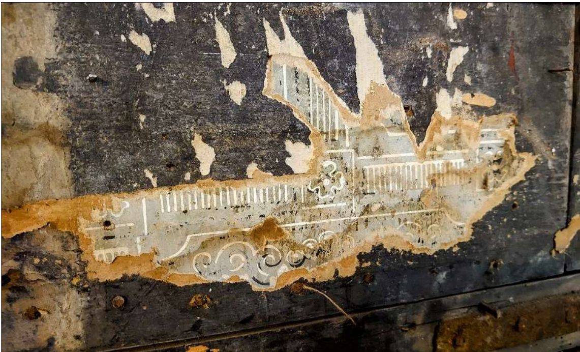
FIGURE 29: THE EARLIEST LAYER OVER THE SHUTTERS, A REGENCY STYLE BLOCK-PRINTED WALLPAPER, OVERLAID BY FRAGMENTS OF NEWSPAPER.
