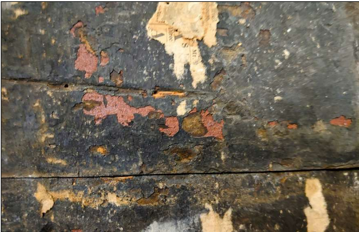
FIGURE 27: FRAGMENTS OF RED PAINT, UNDER A BITUMEN-LIKE BLACK TAR PAINT ON THE LARGEST OF THE SHUTTERS USED ON THE WALL OF R2.
