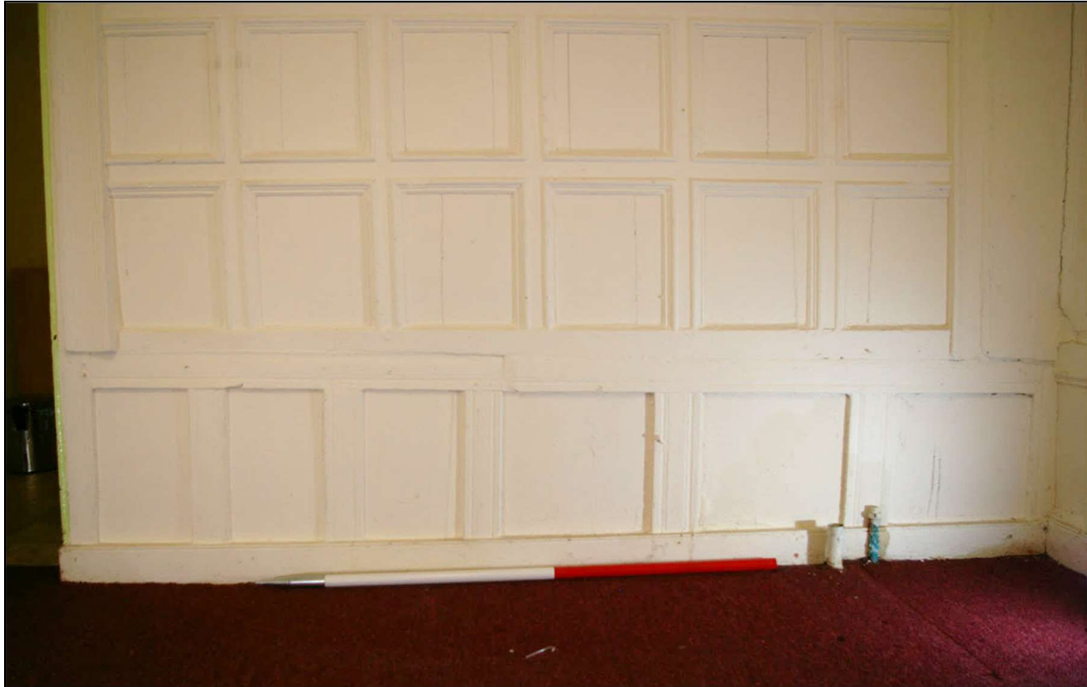
FIGURE 11: TWO PHASES OF PANELLING AT THE BASE OF THE NORTH WALL, TYPE 1 AND TYPE 2; FROM THE SOUTH (1M SCALE).
