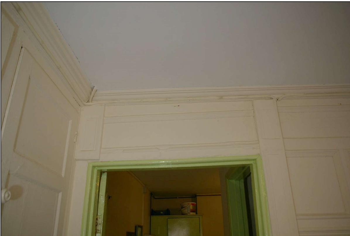
60. THE RESET PANELS ABOVE D25 ON THE NORTH WALL; FROM THE SOUTH.
