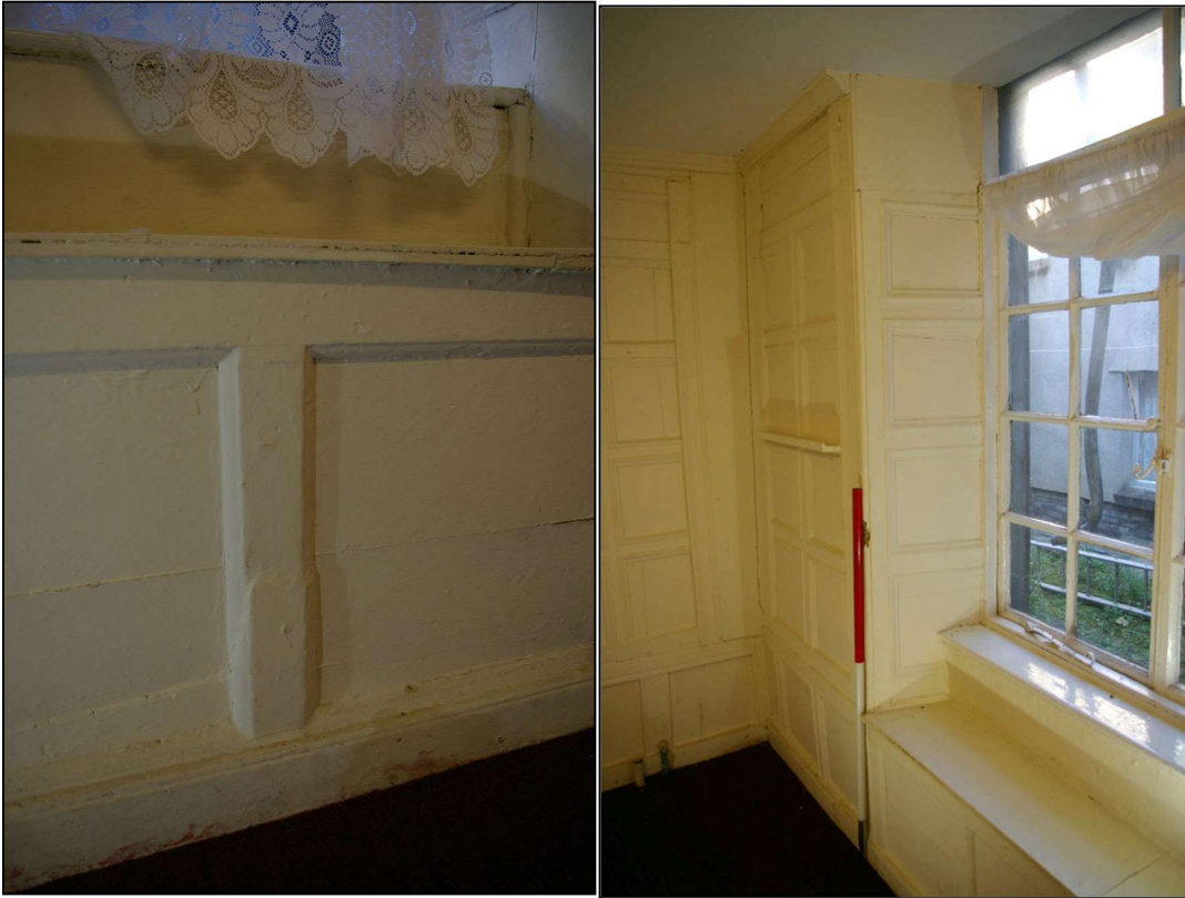
71. LEFT: THE CHUNKY BEAD MOULDING UNDER THE WINDOW SEAT, ON THE EAST WALL; FROM THE NORTH-WEST.
