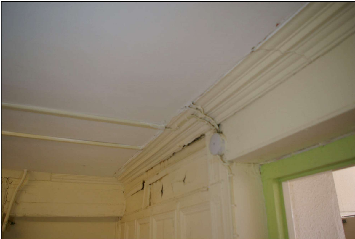
78. THE COMPLEX DEEP CORNICE OF OGEE, CAVETTO, OVOLO AND BEADING, ALONG THE SOUTH WALL; FROM THE WEST-NORTH-WEST.
