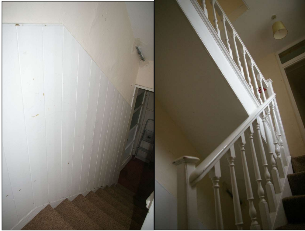
FIGURE 17 A & B: A (LEFT) THE BEADED PLANK PANELLING ON THE PARTITION WALL BETWEEN R5 AND R3; FROM THE NORTH-EAST. B (RIGHT) THE MOULDED HANDRAIL ATTACHED TO THE NEWEL POST, THE BANISTERS AND DETAILED VIEW OF THE TURNED BALUSTERS; FROM THE EAST-NORTH-EAST.
