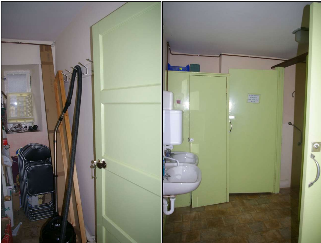
35. LEFT: R18, THE MID-20 TH CENTURY CUPBOARD STRUCTURE; FROM THE WEST.
