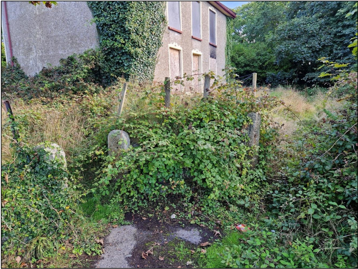
FIGURE 16: GATE POSTS GIVING ACCESS TO THE FRONT AND REAR GARDENS, VIEWED FROM THE NORTH-WEST.
