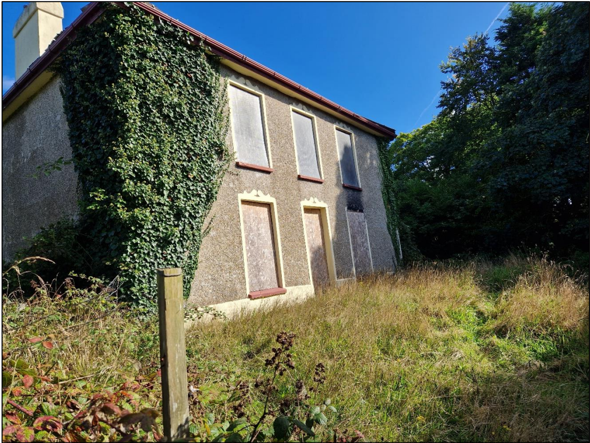
3. CHURCH VIEW, WEST ELEVATION, VIEWED FROM THE NORTH-WEST.
