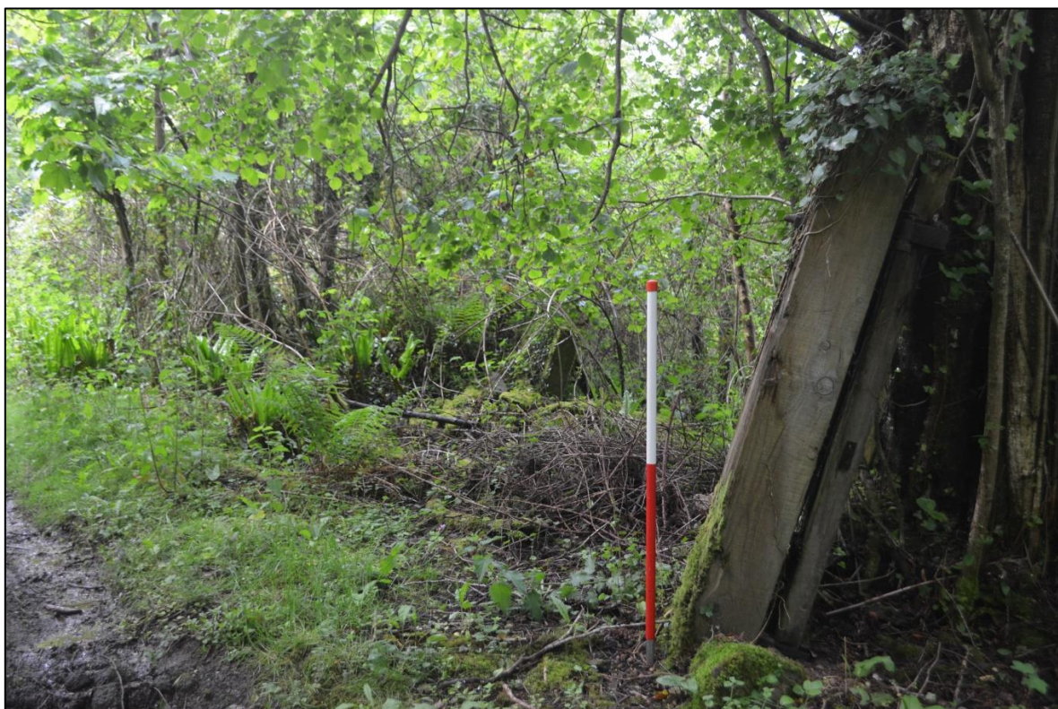
FIGURE 42: SHORT SECTION OF CONCRETE BLOCK WALL IN BACKGROUND WITH WOODEN GATEPOST AND FENCE IN FOREGROUND; FROM THE NORTH (1M SCALE).
