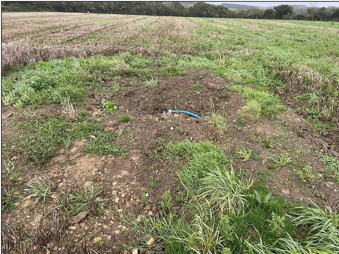
4. F1, DETAIL OF THE PARTIALLY BURIED WATER PIPE; VIEWED FROM THE NORTH-WEST (NO SCALE).
