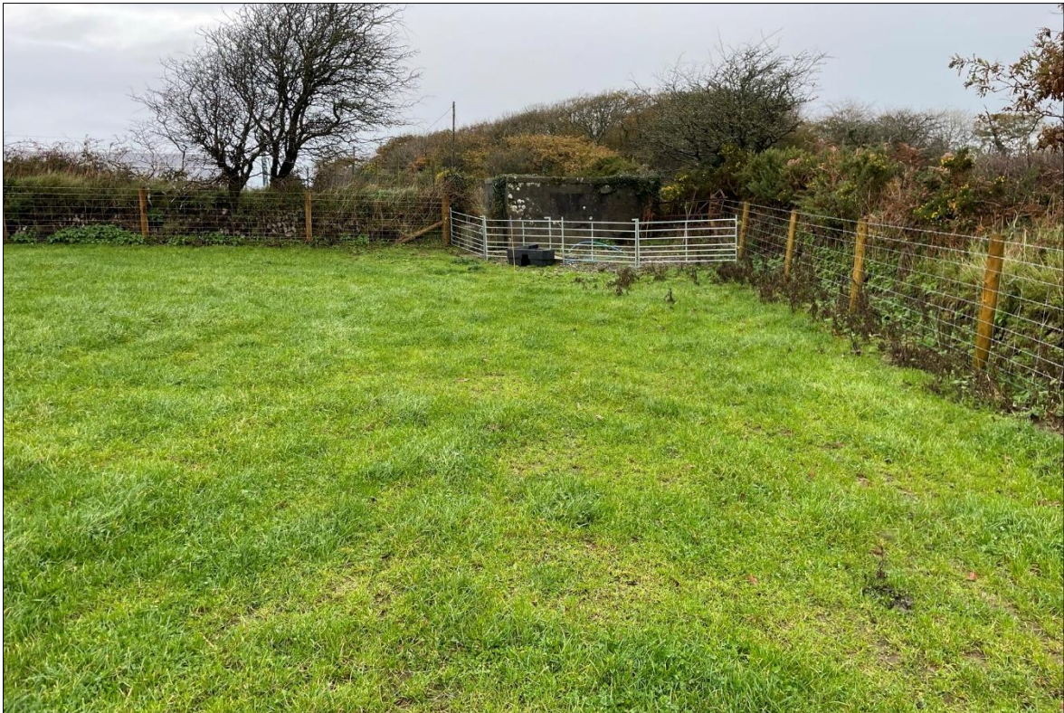
FIGURE 15: F2, VIEW OF THE CONCRETE BLOCKWORK STRUCTURE IN THE NORTH-EASTERN CORNER OF THE FIELD, WITH DETAIL OF THE HEDGEBANK AND FENCE-LINE BOUNDARIES; VIEWED FROM THE SOUTH (NO SCALE).
