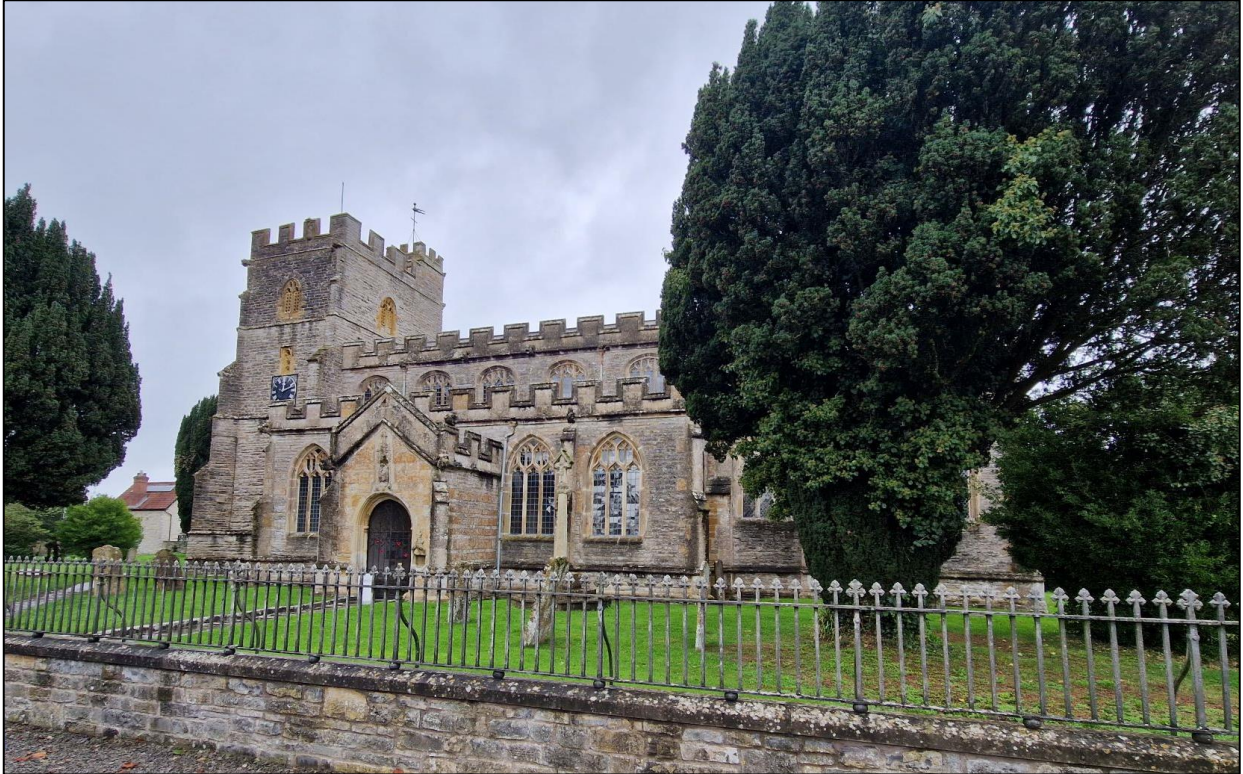
1. ST ANDREWS CHURCH, HIGH HAM; VIEWED FROM THE SOUTH.
