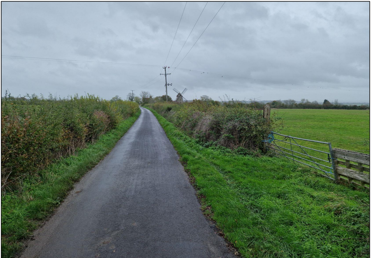
2. STEMBRIDGE TOWER WINDMILL, VIEWED FROM THE WEST.
