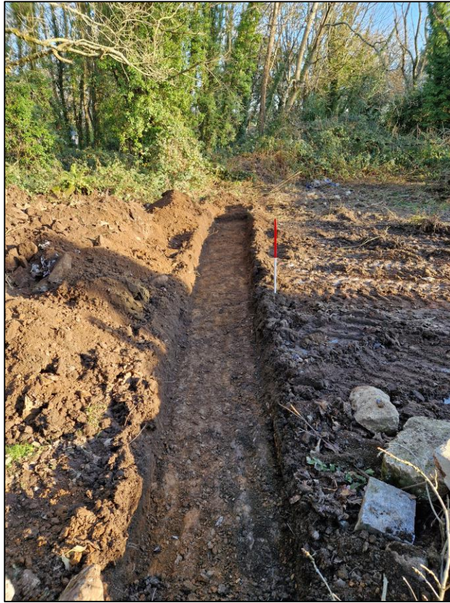
FIGURE 2: TRENCH 4, VIEWED FROM THE SOUTH (1M SCALE).
