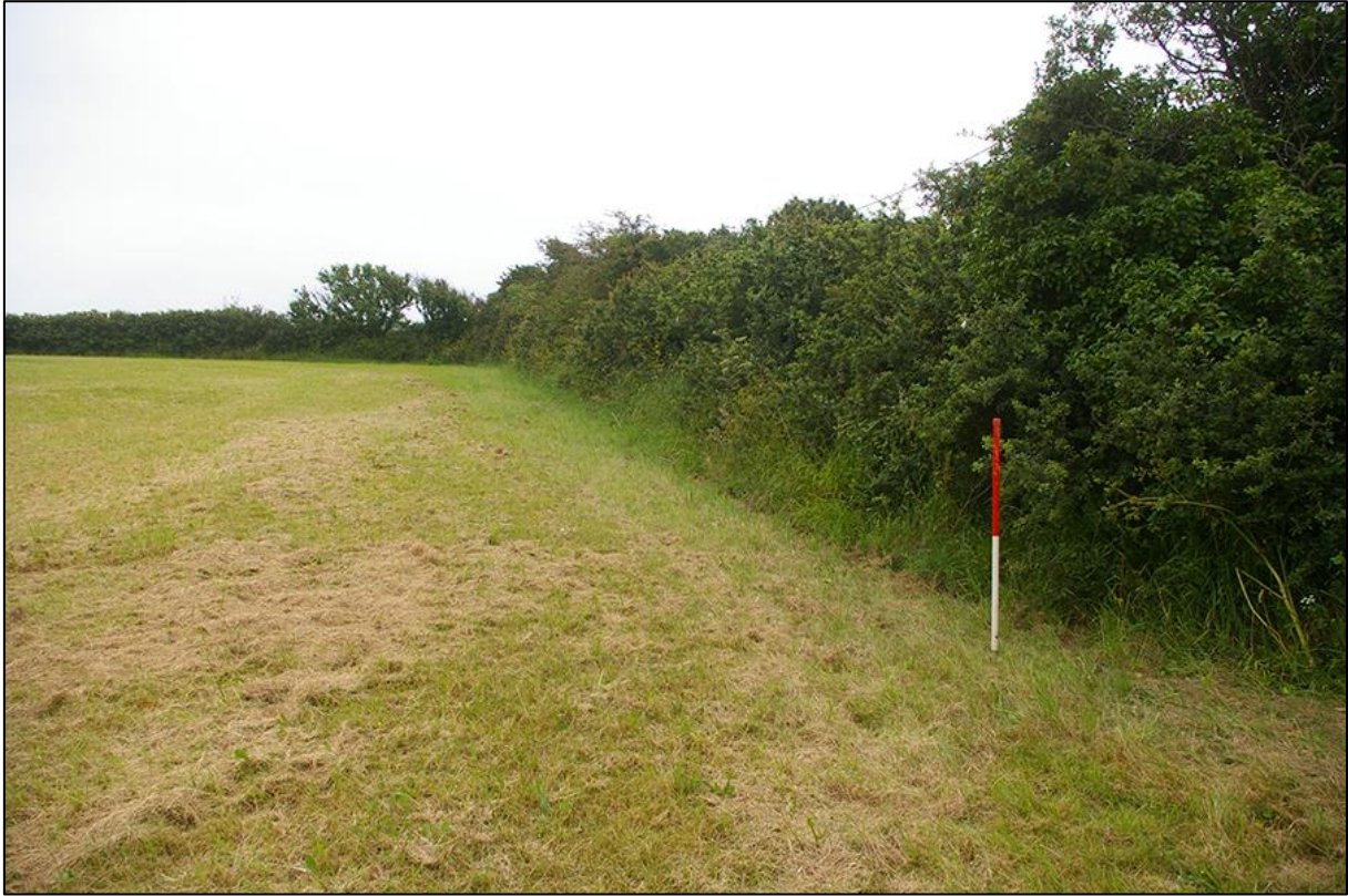
4. DETAIL OF THE NORTHERN ROADSIDE SITE BOUNDARY; VIEWED FROM THE EAST (1M SCALE).
