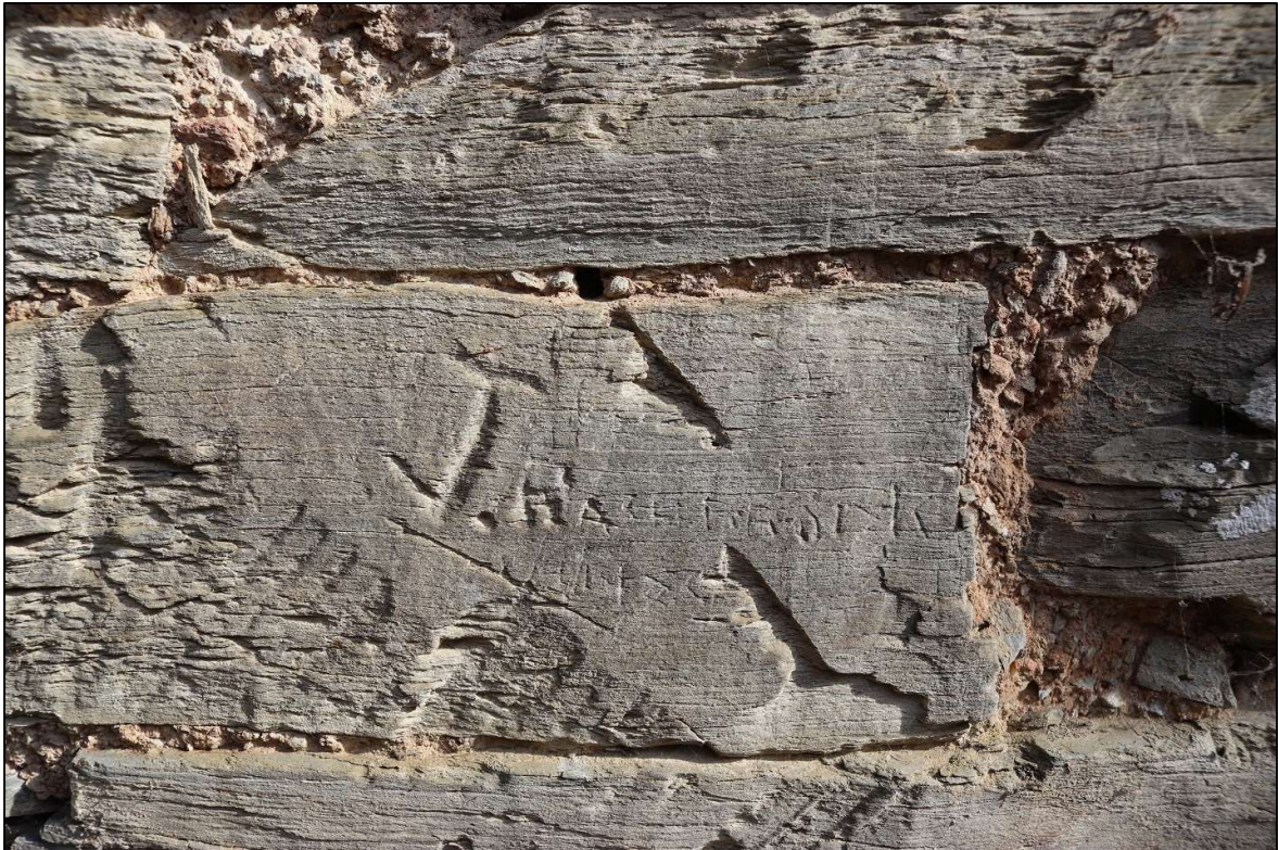
15. THE GRAFFITI SEEN ON SECTION OF WALL AGAINST WEST PIER; VIEWED FROM THE SOUTH.
