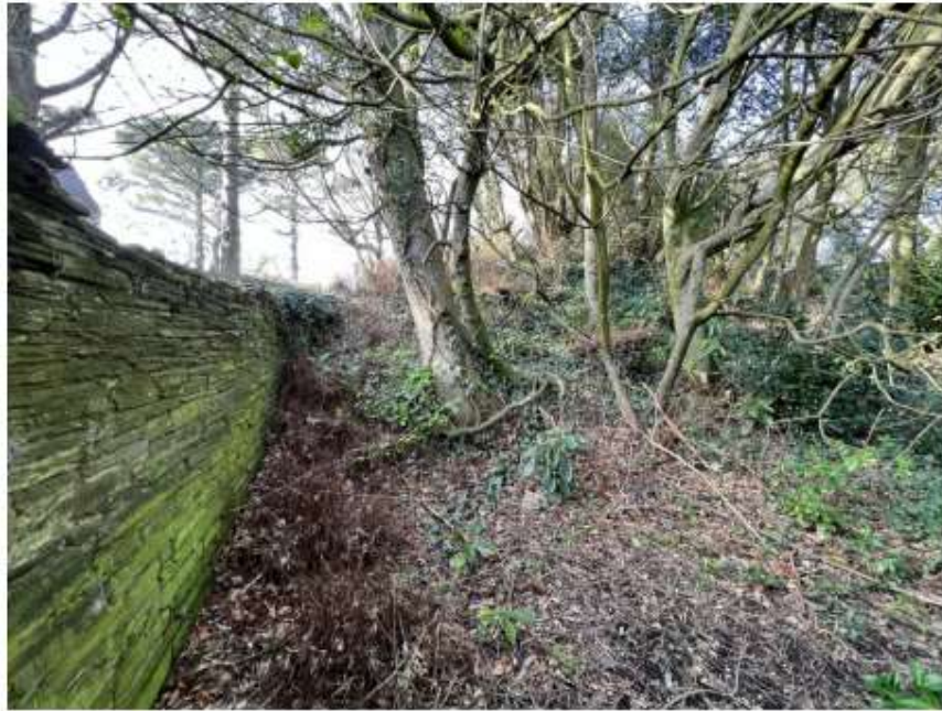
Figure 3 - Boundary wall following Westerly direction ("Rear").
