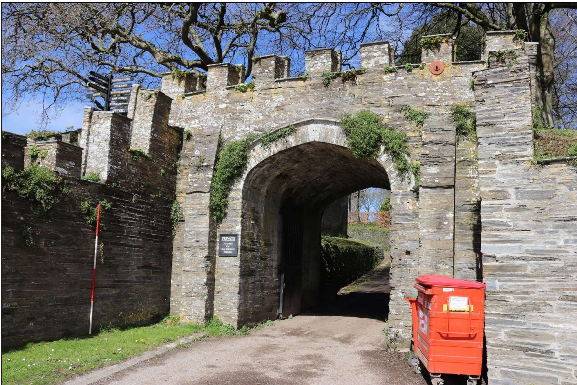
83. THE 19 TH CENTURY FOOTBRIDGE LEADING TO THE ESTATE STABLES; VIEWED FROM THE SOUTH (SCALE 2M).
