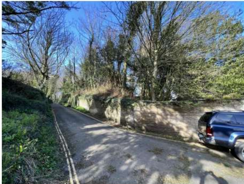
Figure 2 - Boundary wall following Westerly direction ("Front").
