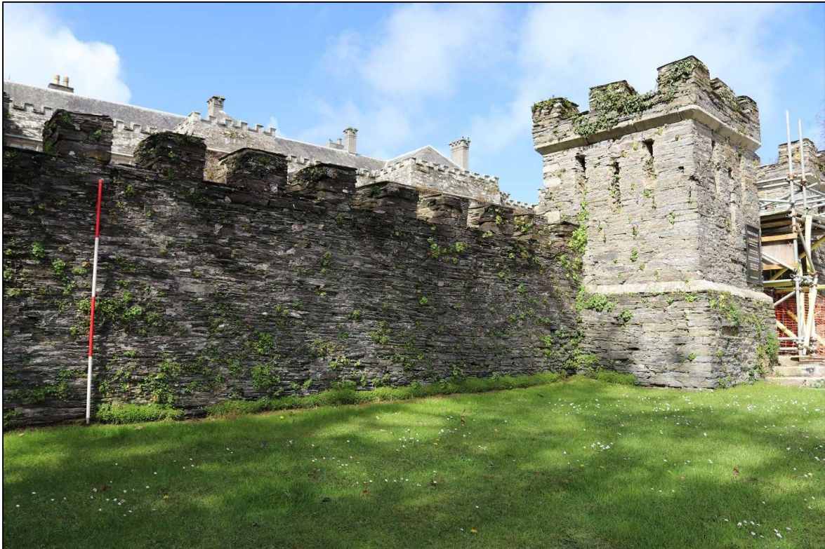
67. THE EXTERNAL FACE OF THE SOUTH WALL AGAINST SOUTH PIER; VIEWED FROM THE SOUTH-EAST (SCALE 2M).
