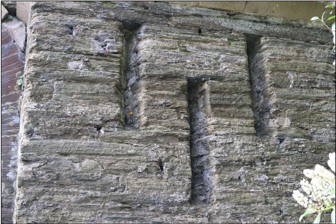
8. THE INSET AND RECESSED 'ARROW SLITS' TO THE WEST ELEVATION OF WEST PIER (SOUTH GATE).
