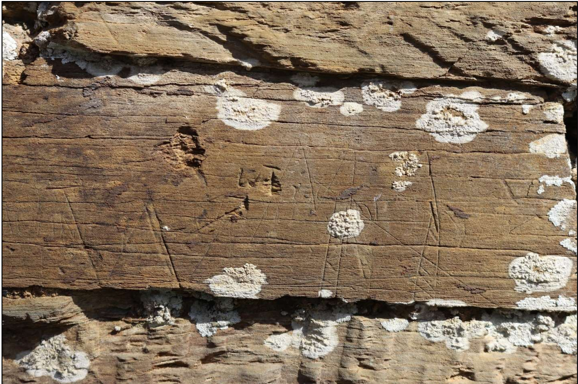
33. THE GRAFFITI SEEN ON SECTION OF WALL AGAINST EAST PIER; VIEWED FROM THE SOUTH.
