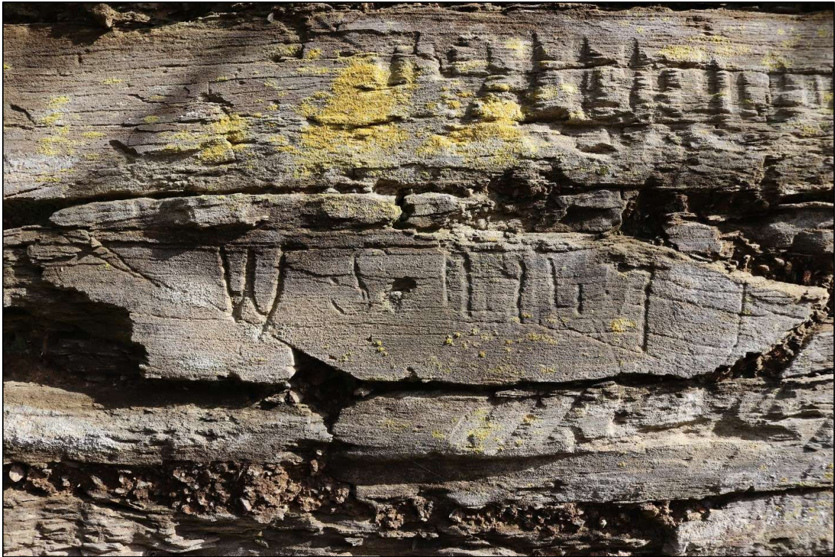
18. THE GRAFFITI SEEN ON SECTION OF WALL AGAINST WEST PIER; VIEWED FROM THE SOUTH.
