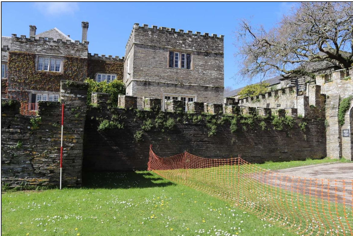
80. THE NORTH WALL WITH DEEP CHAMFER MEETING LATER WALL; VIEWED FROM THE EAST (SCALE 2M).
