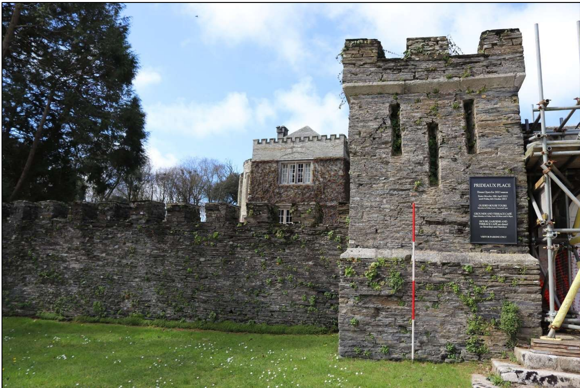
69. THE EXTERNAL FACE OF THE SOUTH WALL AGAINST SOUTH PIER; VIEWED FROM THE EAST (SCALE 2M).
