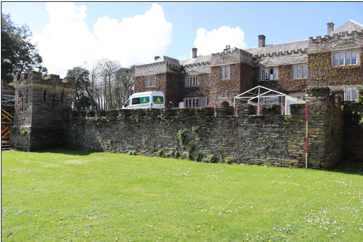
81. THE SECTION OF NORTH WALL FROM THE NORTH PIER LOOKING BACK AT THE HOUSE; VIEWED FROM THE NORTH-EAST (SCALE 2M).
