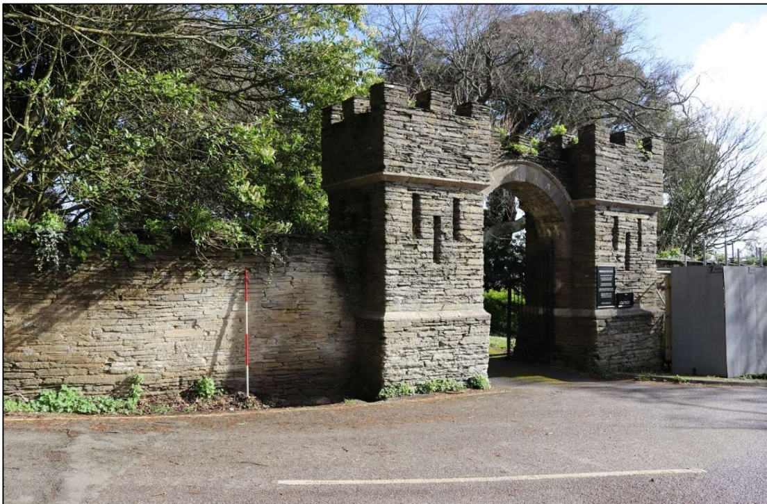
FIGURE 20: THE EXTERNAL ELEVATION OF THE SOUTH GATE; VIEWED FROM THE SOUTH-WEST (SCALE 2M).
