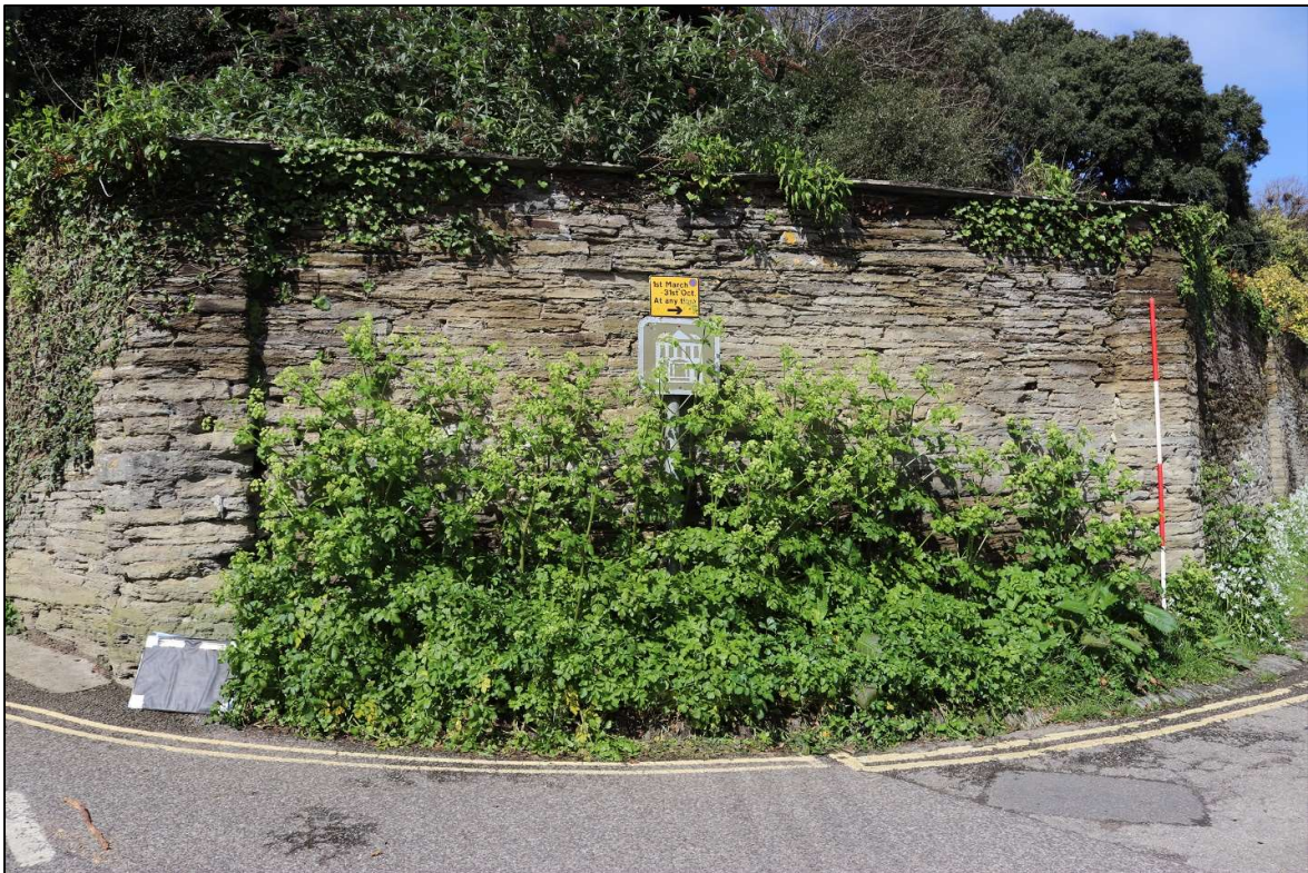
49. THE CORNER OF TREGIRLS LANE; VIEWED FROM THE NORTH-EAST (SCALE 2M).
