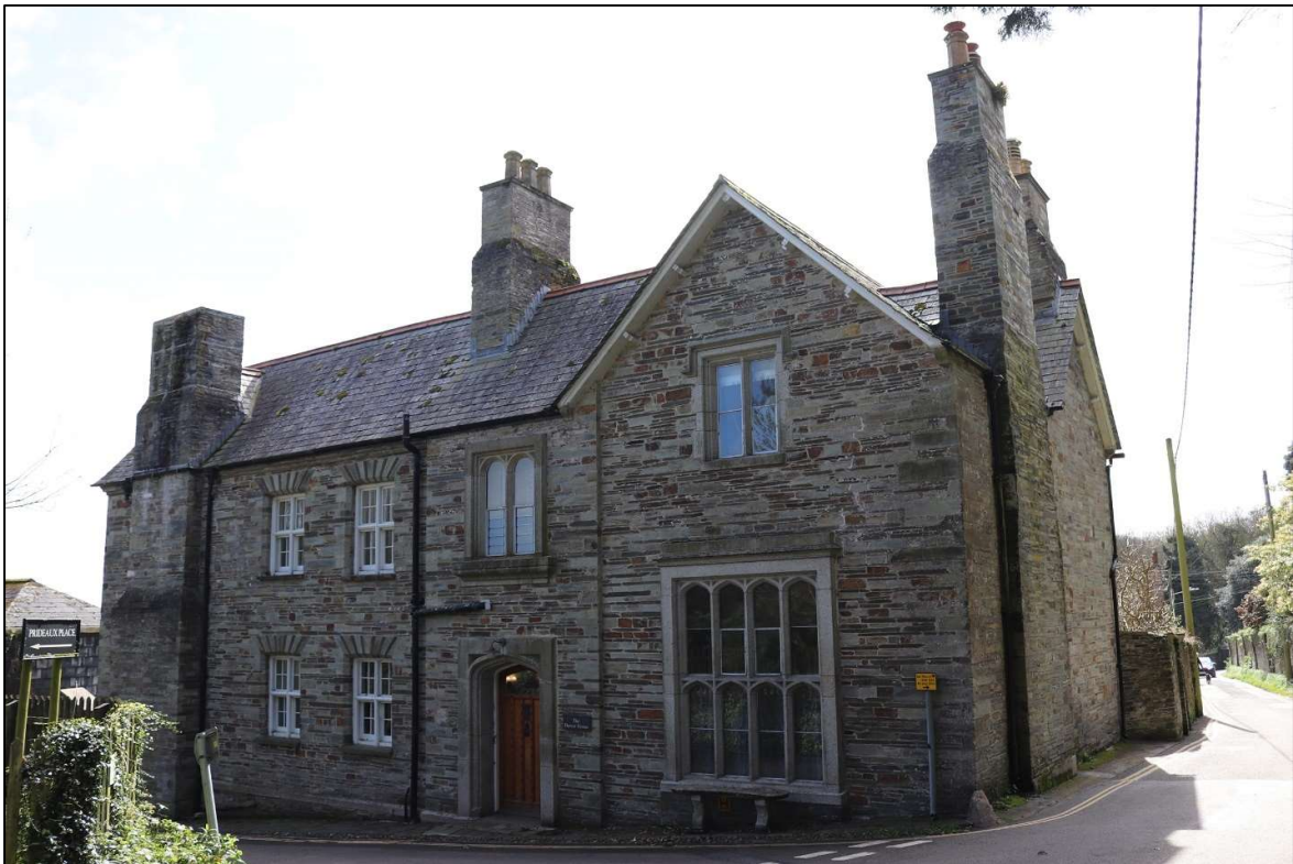
65. THE GRADE II LISTED DOWER HOUSE; VIEWED FROM THE NORTH.
