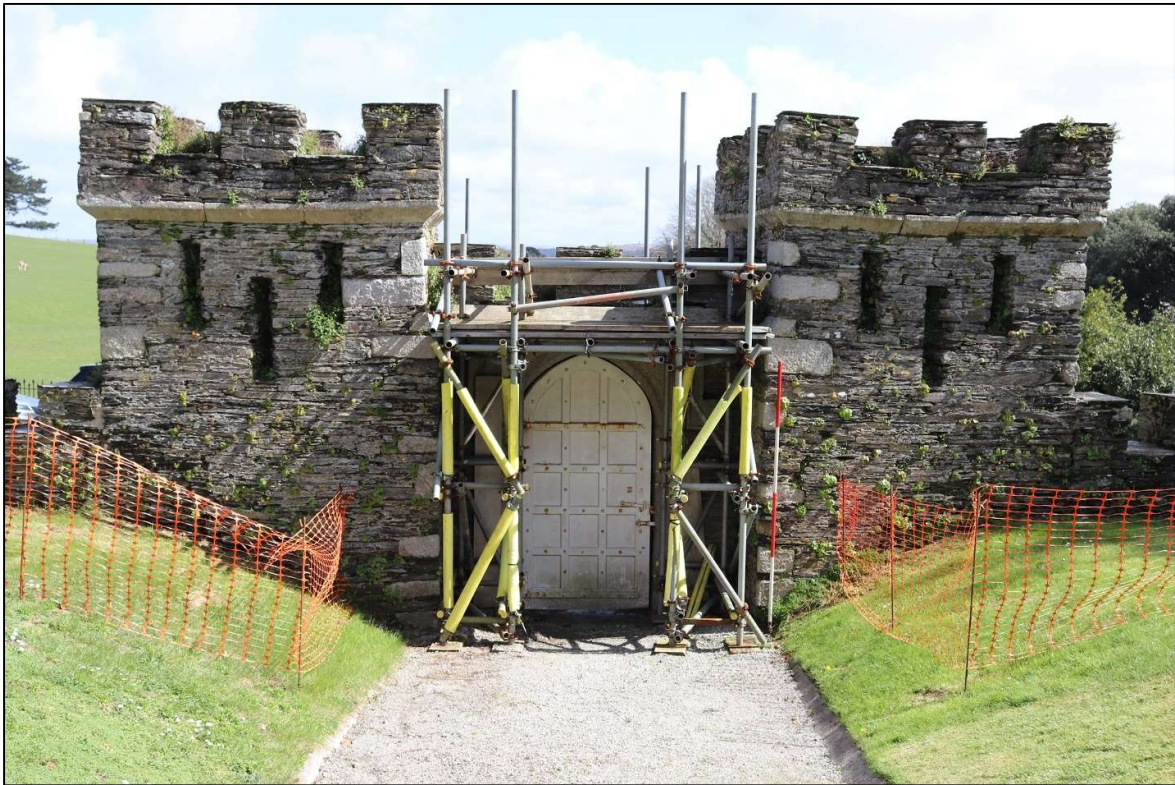
84. INTERNAL FACE OF EAST GATE; VIEWED FROM THE WEST (SCALE 2M).
