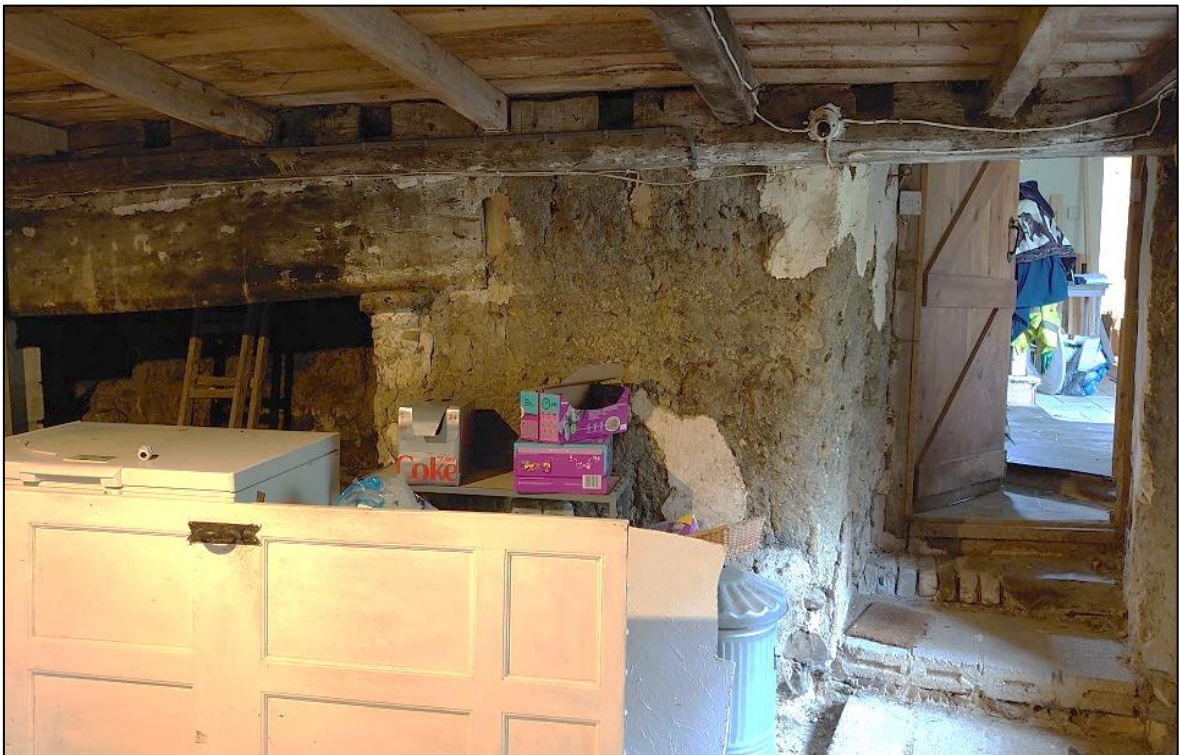
FIGURE 19: R13, THE SMOKE-BLACKENED 16 TH OR 17 TH CENTURY KITCHEN WITHIN THE BARN; VIEWED FROM THE SOUTH-EAST.
