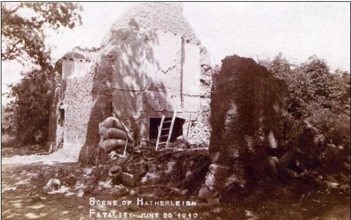
FIGURE 10: 1910 IMAGE OF THE PARTLY-COLLAPSED COB BUILDING RESPONSIBLE FOR THE DEATHS (NORTH DEVON RECORD OFFICE ARCHIVES AND ACCESSED VIA HATHERLEIGH HISTORY ARCHIVE WEBSITE 2022).
