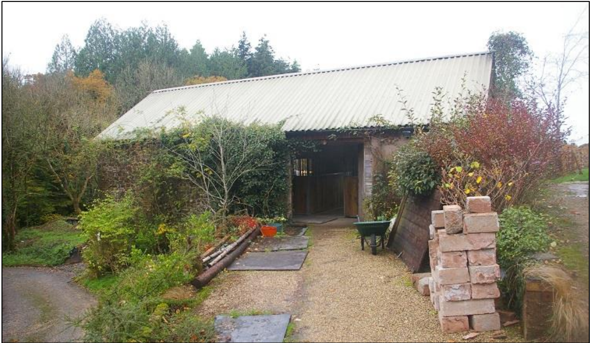
FIGURE 21: THE STABLES, FORMERLY THE THRESHING BARN; VIEWED FROM THE EAST.
