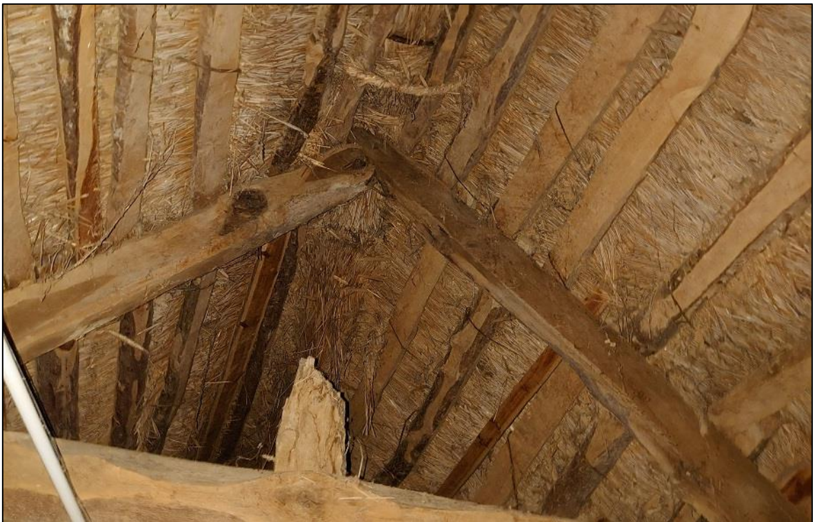
FIGURE 16: VIEW OF THE ROOF STRUCTURE OVER THE HOUSE.
