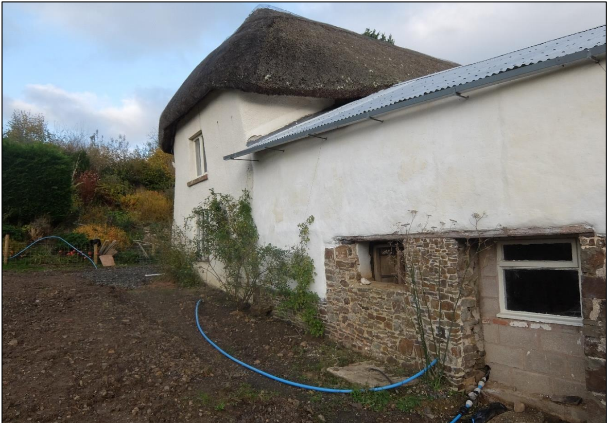
FIGURE 17: THE JUNCTION BETWEEN THE HOUSE (LEFT) AND THE BARN (RIGHT) SHOWING THE PHASES OF REBUILDING AND FORCED OPENINGS; VIEWED FROM THE SOUTH-WEST (CLIENT PHOTOGRAPH).
