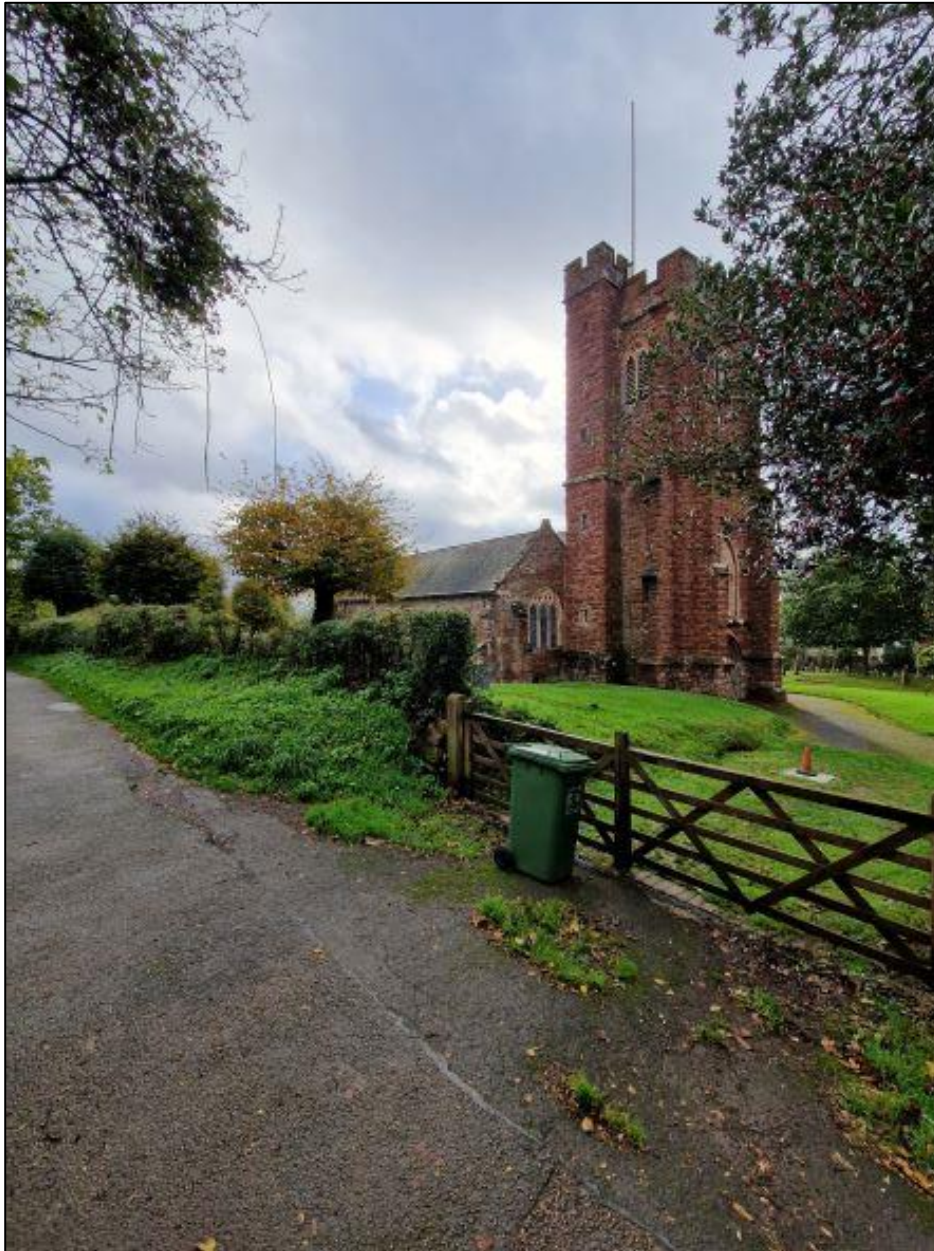
FIGURE 11: ST MICHAEL AND ALL ANGELS CHURCH VIEWED FROM THE NORTH-EAST.
