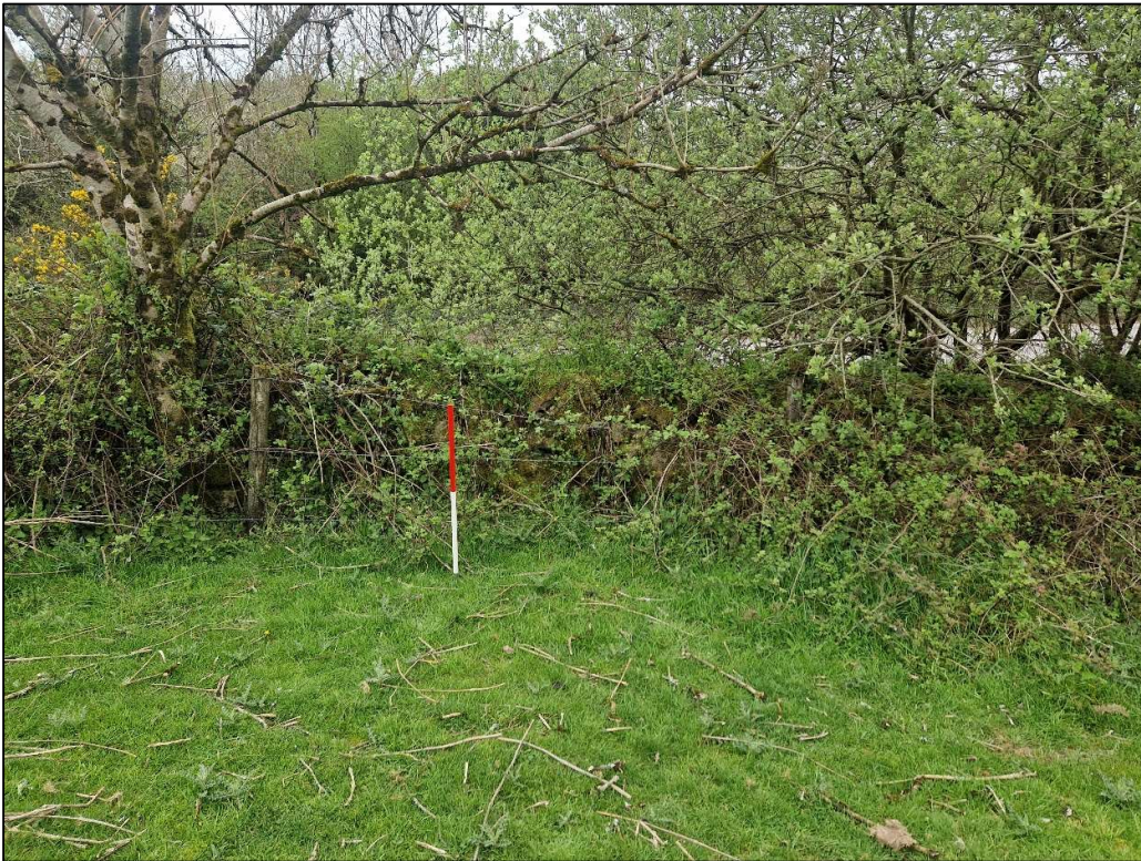
4. F1, DETAIL OF THE WESTERN BOUNDARY; VIEWED FROM THE SOUTH-EAST (1M SCALE).
