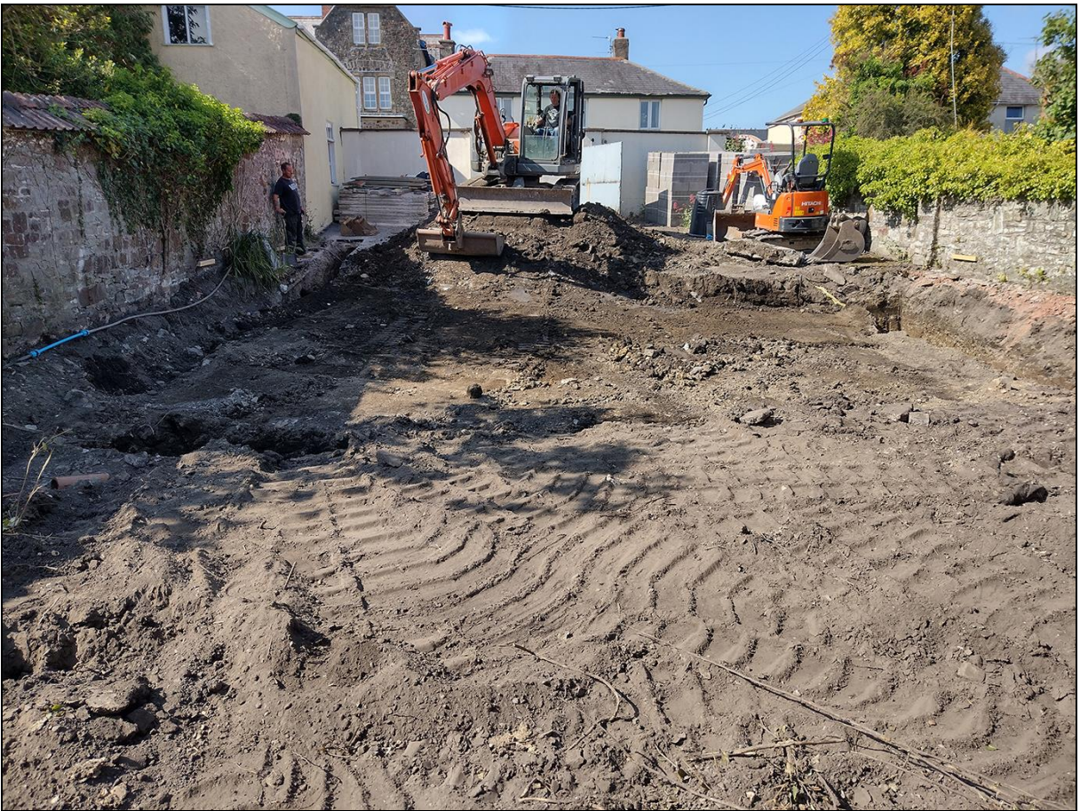
FIGURE 3: SITE SHOT, MID EXCAVATION; VIEWED FROM THE SOUTH (NO SCALE).
