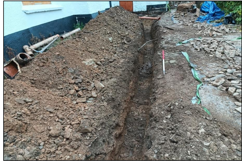
FIGURE 15: THE SERVICE TRENCH, AS VIEWED FROM THE NORTH (1M SCALE).
