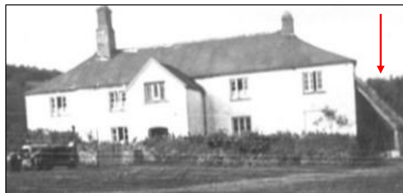
FIGURE 7: PHOTOGRAPH OF WOODLANDS, LIKELY 1900-1940, HELD IN GREAT TORRINGTON HERITAGE MUSEUM ARCHIVE, NOTED MR HUXTABLES HOUSE ON THE BACK.
