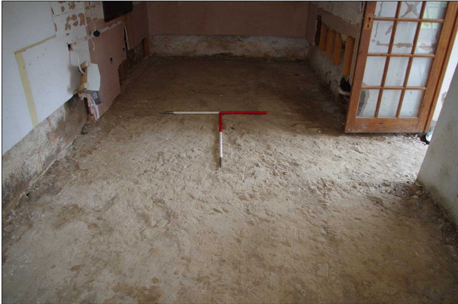
FIGURE 13: THE LIMECRETE FLOOR (101) BEFORE SECTIONING AND EVENTUAL EXCAVATION; FROM THE SOUTH (2 x 1M SCALES).
