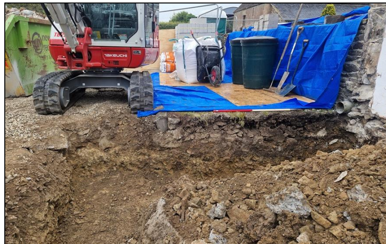
FIGURE 10: VIEW OF EXPOSED FOOTINGS (OF 19 TH CENTURY LEAN-TO?), FROM THE WEST (1M SCALE).
