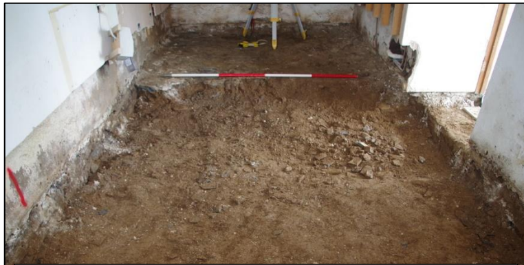
Plate 11: View of almost fully excavated and removed cobbled floor, showing depth of made ground packing beneath that and above the natural yellow-grey clay, 2m scale, from the east.
