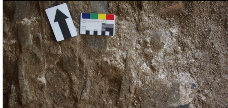
Plate 8: Detailed view of the lime and earth mixed fabric (105), with slates, which packs the sunken areas of the limecrete floor (107), with photocard scale.
