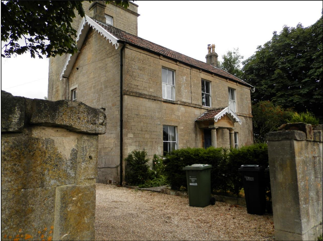
11. FRONT ELEVATION OF TOWER HOUSE FROM BLOOMFIELD ROAD (NO SCALE).
