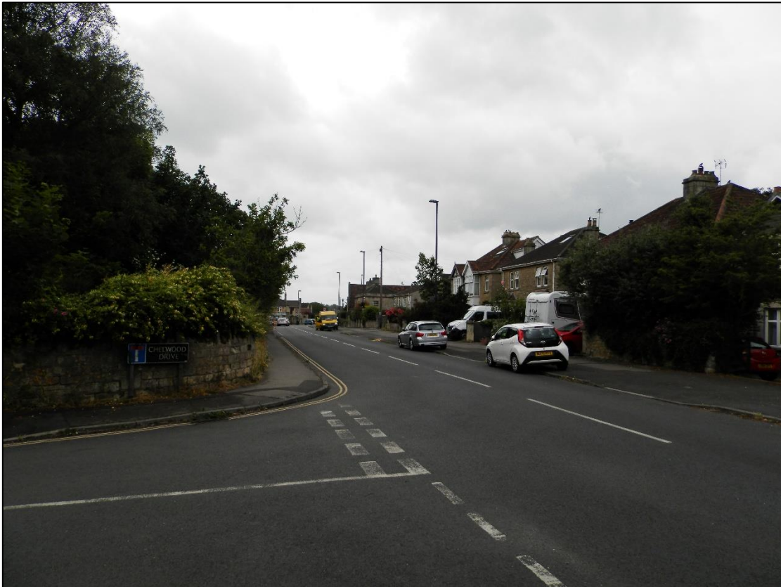
12. VIEW SOUTH ALONG BLOOMFIELD ROAD FROM ENTRANCE TO ODD DOWN COMPRISING SOUTHERN EXTENT OF CITY OF BATH CONSERVATION AREA (NO SCALE).
