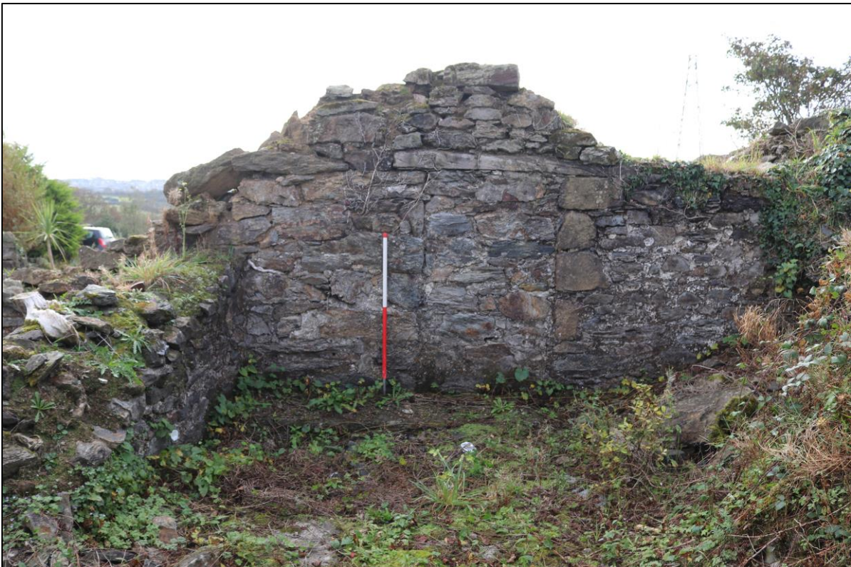
16. BLOCKED DOORWAY TO WEST BLOCK; FROM THE NORTH WITH 1M SCALE.
