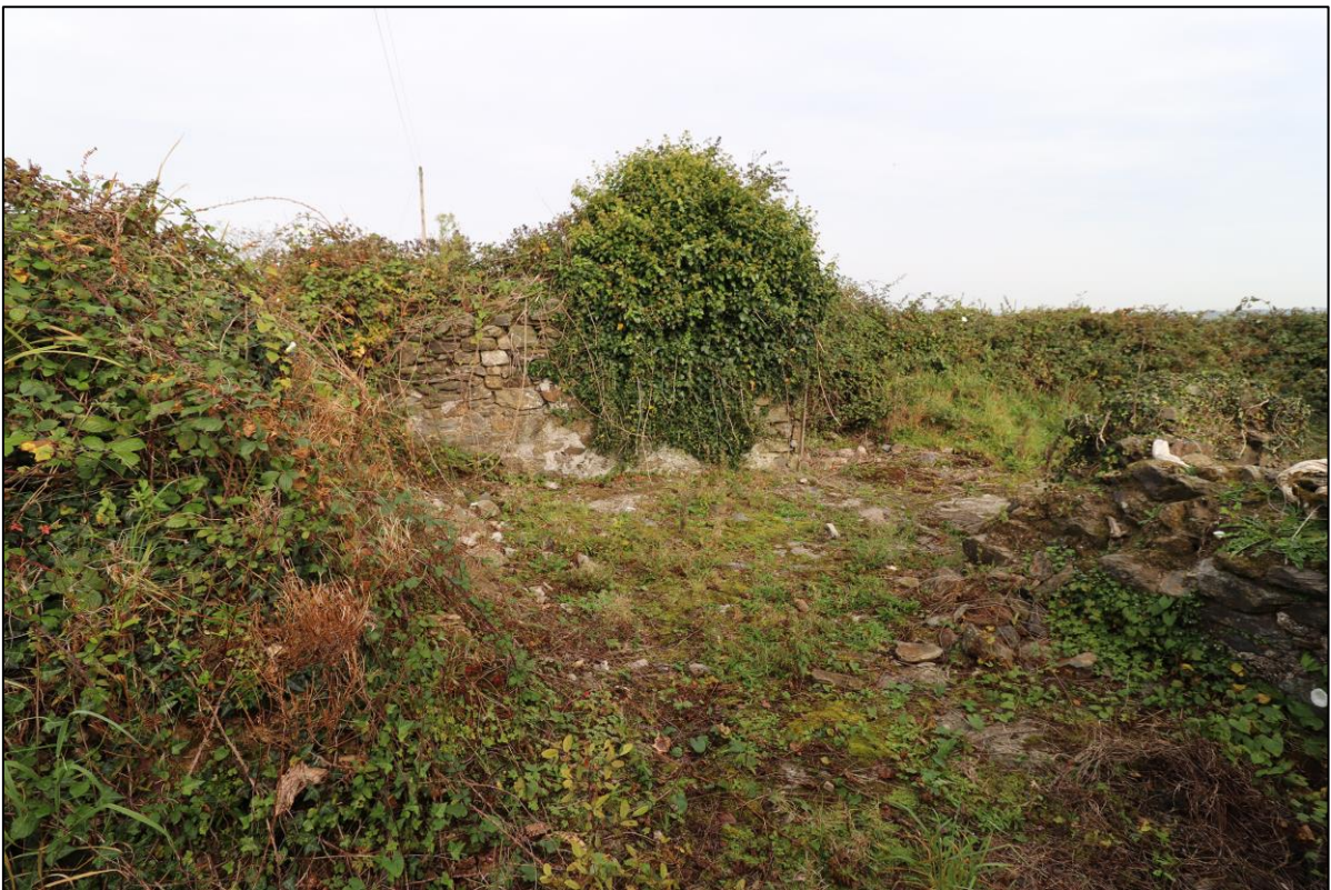
20. THE NORTH WALL OF NORTH WEST BLOCK; FROM THE SOUTH TAKEN WITH WIDE-ANGLED LENS.
