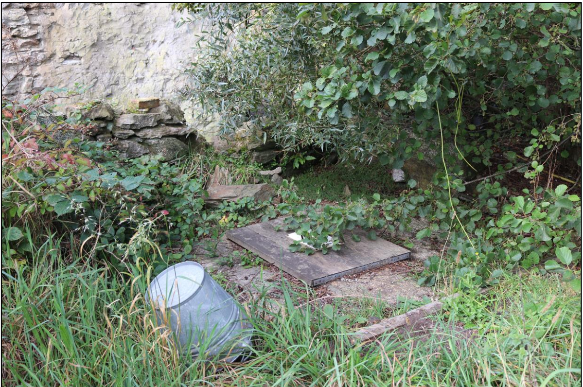
42. THE BOARDED UP WELL TO THE NORTH-WEST CORNER OF GARDEN; FROM THE SOUTH- EAST.
