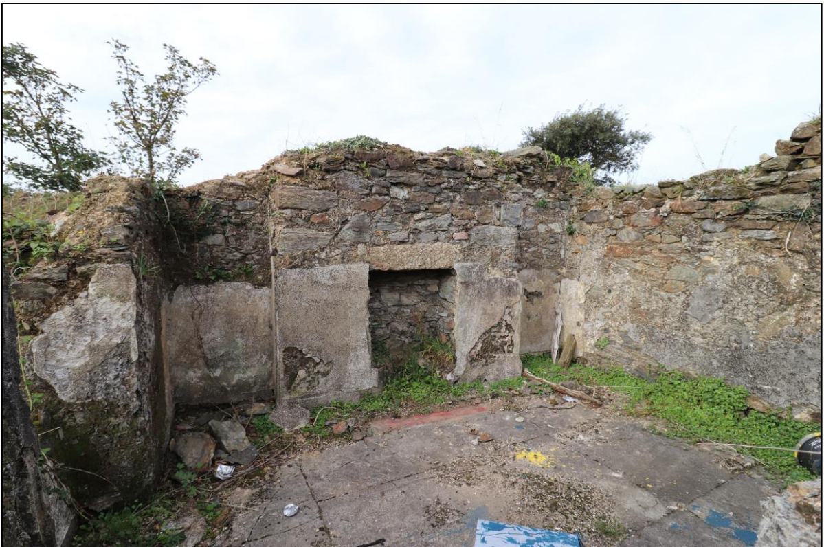
46. THE WEST BLOCK EXTENSION TAKEN WITH WIDE-ANGLED LENS FROM THE SOUTH-EAST.
