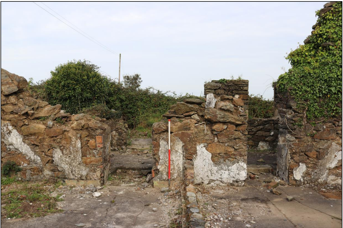
34. THE PAIR OF FORCED OPENING TO THE NORTH ELEVATION FOR REAR SERVICES; FROM THE SOUTH WITH 1M SCALE.
