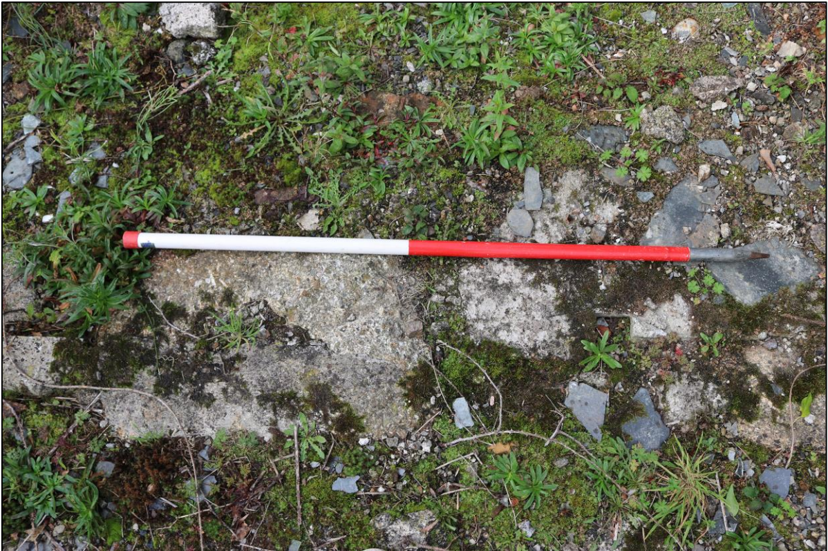
19. SCREED WRAPPING SOCKET TO THRESHOLD OF NORTH WEST EXTENSION.
