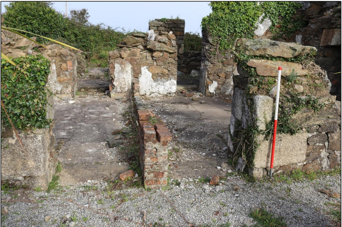
4. DETAIL OF THE SOUTH OPENINGS FOR BOTH COTTAGES, DIVIDED WHEN COTTAGE SPLIT TO TWO DWELLINGS C1843-1881. FROM THE SOUTH-WEST WITH 1M SCALE.
