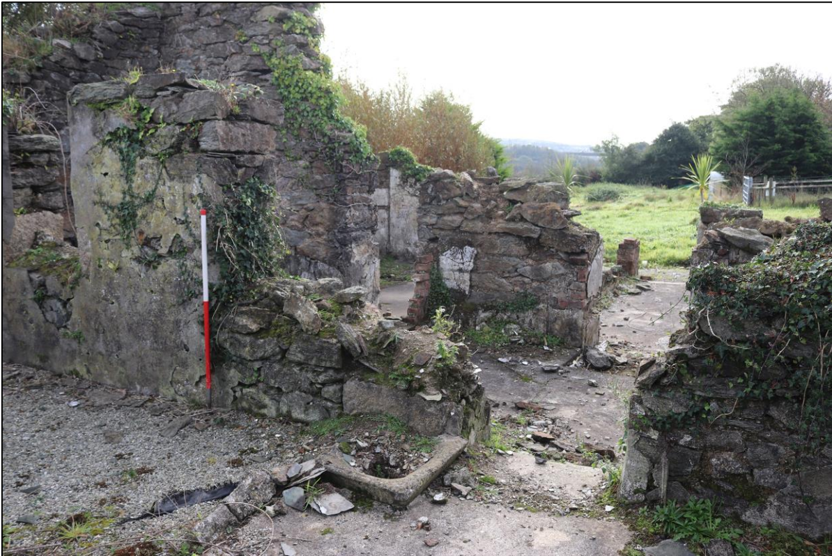
13. PAIR OF FORCED DOORWAYS TO NORTH INTERNAL ELEVATION AND OPENING TO C2 COURTYARD; FROM THE NORTH-WEST WITH 1M SCALE.
