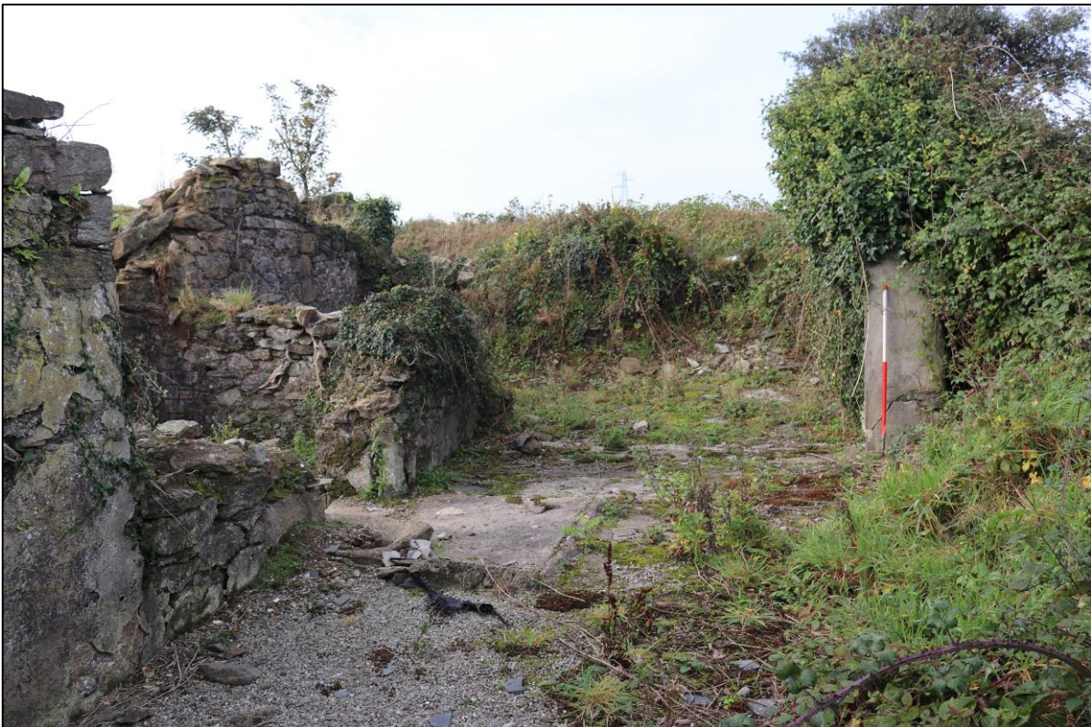
14. VIEW TO NORTH EXTENSION ON WEST BLOCK; FROM THE EAST WITH 1M SCALE.
