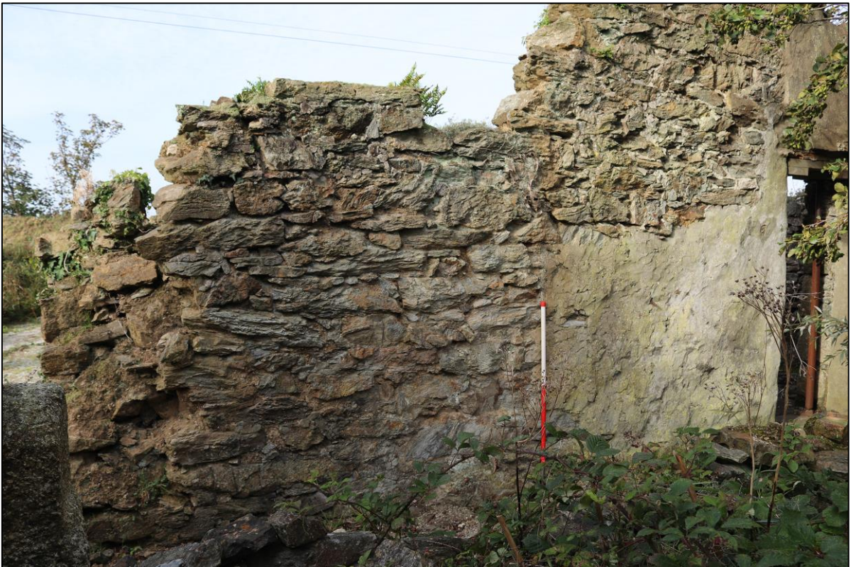
6. THE SOUTH-WEST CORNER, GRANITE QUOINS HAVE BEEN ROBBED OUT. TAKEN FROM THE EAST WITH 1M SCALE.
