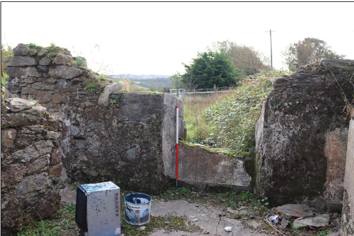
38. THE POSSIBLE BLOCKED DOOR NOW WINDOW TO SOUTH ELEVATION OF WEST BLOCK; FROM THE NORTH WITH 1M SCALE.
