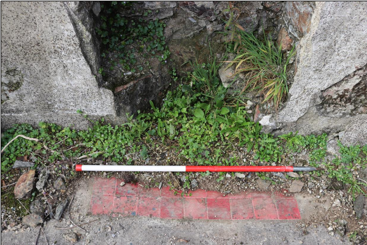
37. THE STACK HAD BEEN REWORKED IN MID-20 TH INCLUDING QUARRY TILE THRESHOLD.
