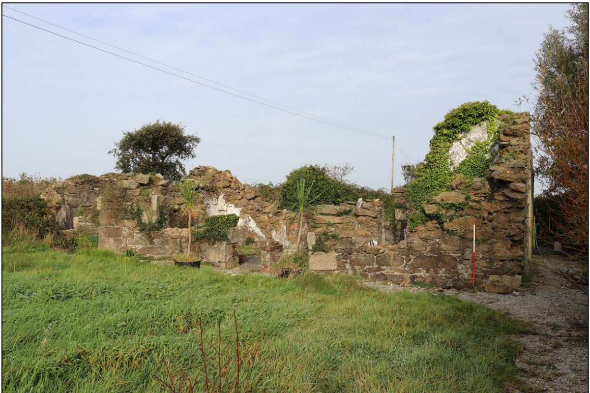
2. THE SOUTH FRONT; FROM THE SOUTH WITH 1M SCALE.
