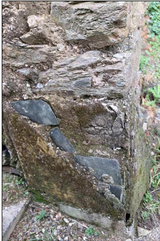
35. THE REUSED SLATES SEEN UNDER INTERNAL RENDERING.
