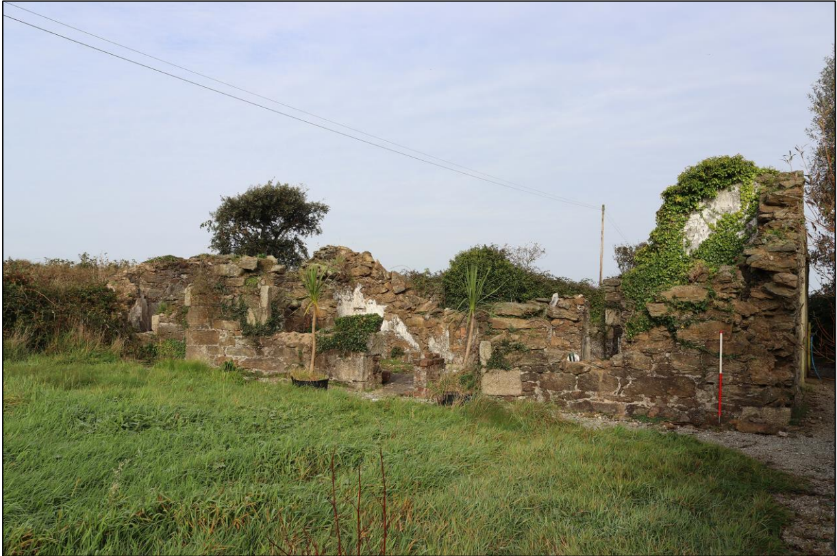
FIGURE 7: THE RUINOUS SOUTH FRONT, FROM THE SOUTH-EAST WITH 1M SCALE.
