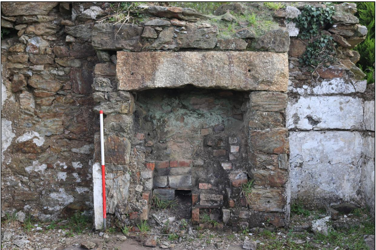
30. DETAIL OF THE STACK C1, FROM THE WEST 1M SCALE.
