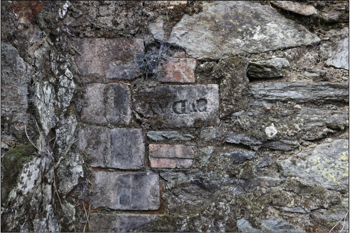
23. ST DAY BRICKWORKS CLOSED IN 1912.
