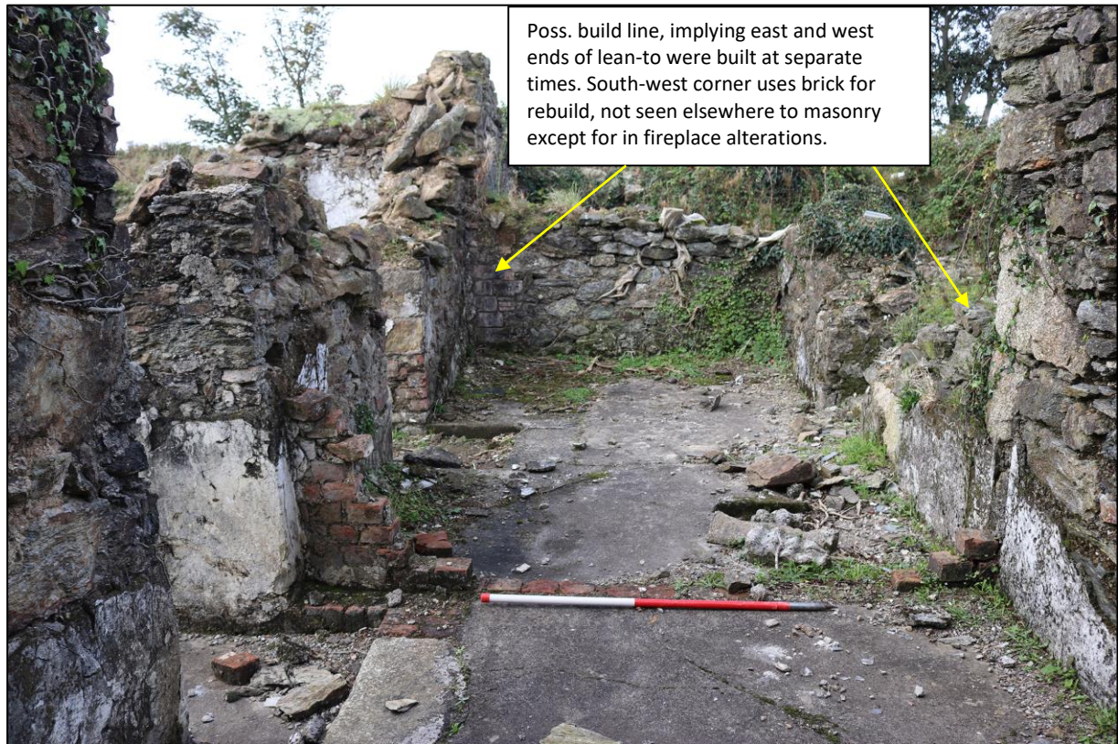
FIGURE 11: THE WEST END OF LEAN-TO, SHOWING POSSIBLE BUILD LINE TO NORTH. FROM THE EAST WITH 1M SCALE.
