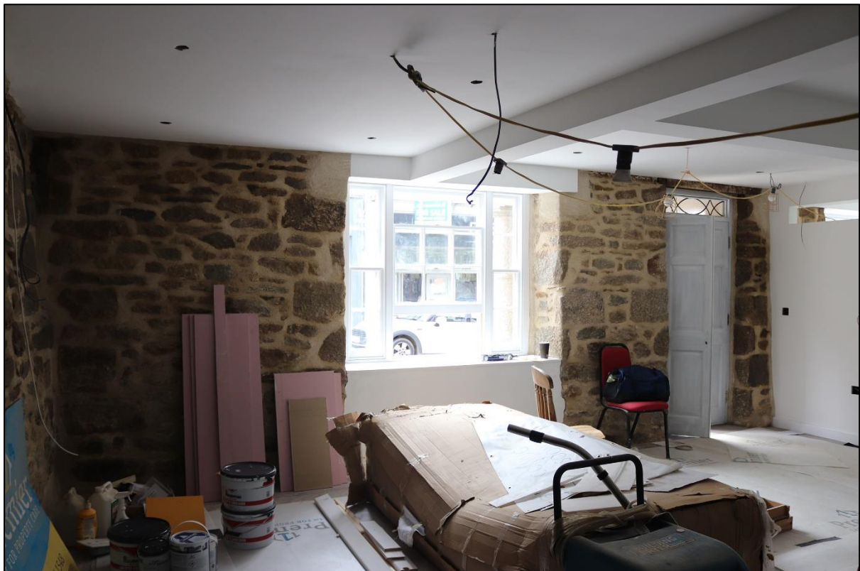
FIGURE 14: THE EXPOSED SOUTH WALL. TAKEN FROM THE NORTH-EAST.
