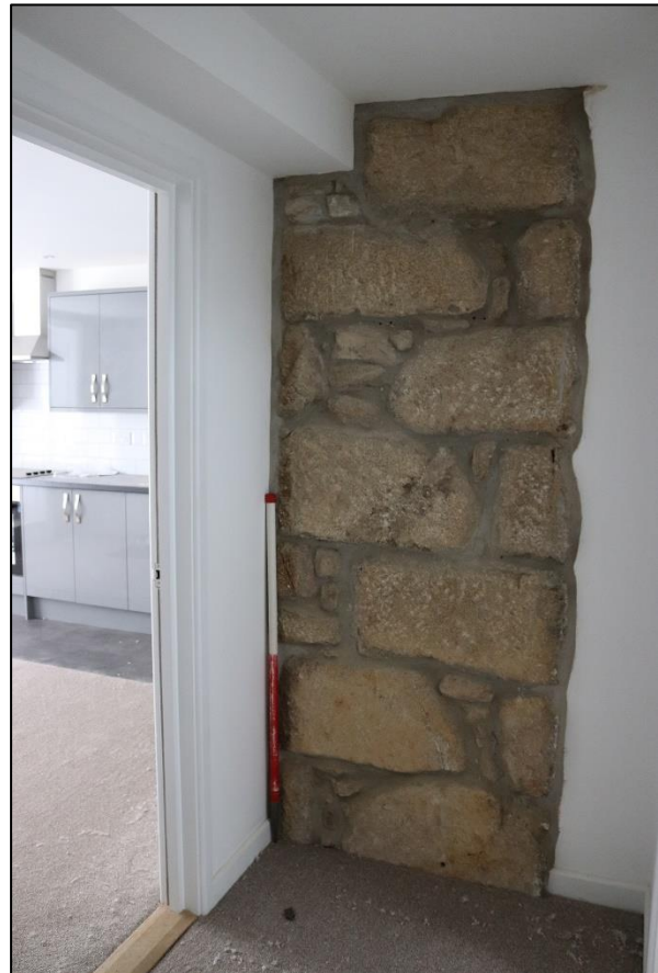
16. LEFT: SMALL BEDROOM TO REAR FF WEST FLAT SHOWING EXPOSED SECTION WITH QUOIN DRESSINGS. RIGHT: INCLUDING SIMILAR FABRIC SEEN ON ENTRANCE TO FLAT FROM THE WEST. BOTH WITH 1M SCALES.
