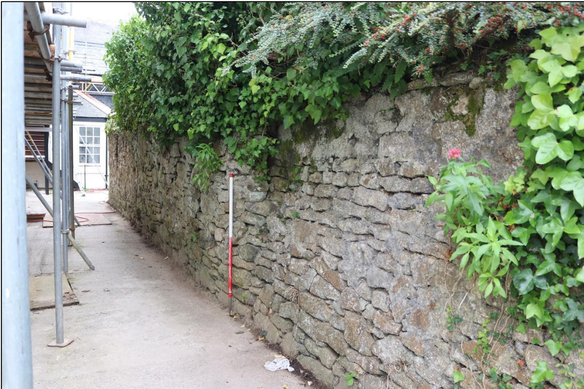
32. THE SURVIVING SECTION OF RUBBLE WALL TO THE EAST SIDE FROM THE NORTH WITH 1M SCALE.
