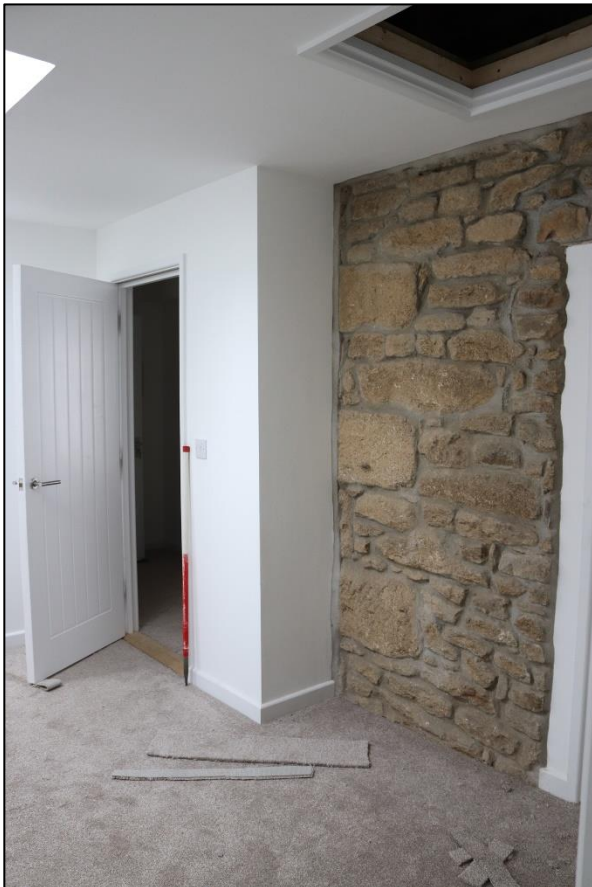
16. LEFT: SMALL BEDROOM TO REAR FF WEST FLAT SHOWING EXPOSED SECTION WITH QUOIN DRESSINGS. RIGHT: INCLUDING SIMILAR FABRIC SEEN ON ENTRANCE TO FLAT FROM THE WEST. BOTH WITH 1M SCALES.
