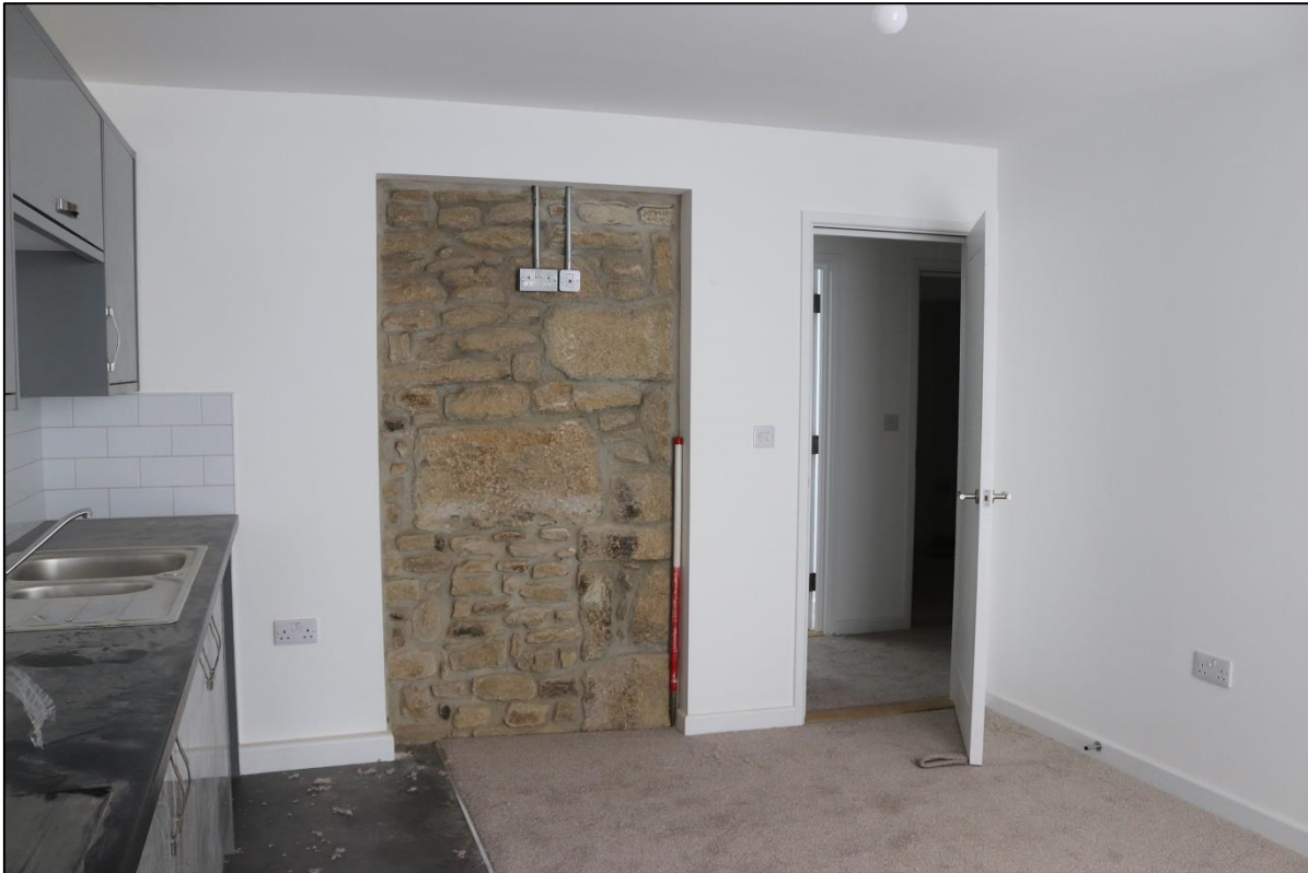
15. REFLECTING EXPOSED STONEMWORK IN THE FF WEST FLAT, WITH SMALL BLOCKED FIREPLACE; FROM THE SOUTH WITH 1M SCALE.
