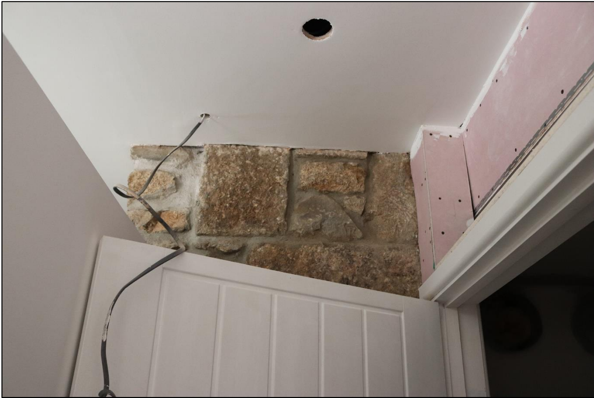
25. REUSED DRESSED GRANITE BLOCKS SEEN TO THE WEST WALL.
