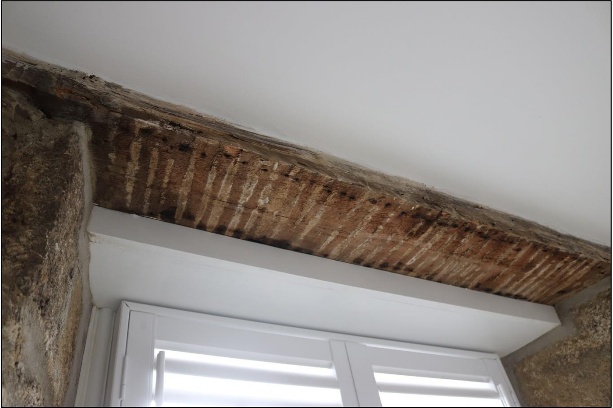
13. THE SURVIVING TIMBER LINTELS TO THE FF FRONTAGE SHOWING SCARRING FOR FORMER LATHE AND PLASTERWORK, WINDOWS REPLACED.
