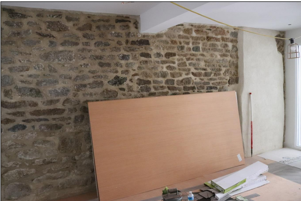
22. THE NOTABLY DIFFERENT MASONRY TO THE REAR GF COMMERCIAL SPACE, WHICH MAY REPRESENT EARLIER FABRIC, INCLUDING BLOCKED FIREPLACE NOW RENDERED; FROM THE WEST WITH 1M SCALES.
