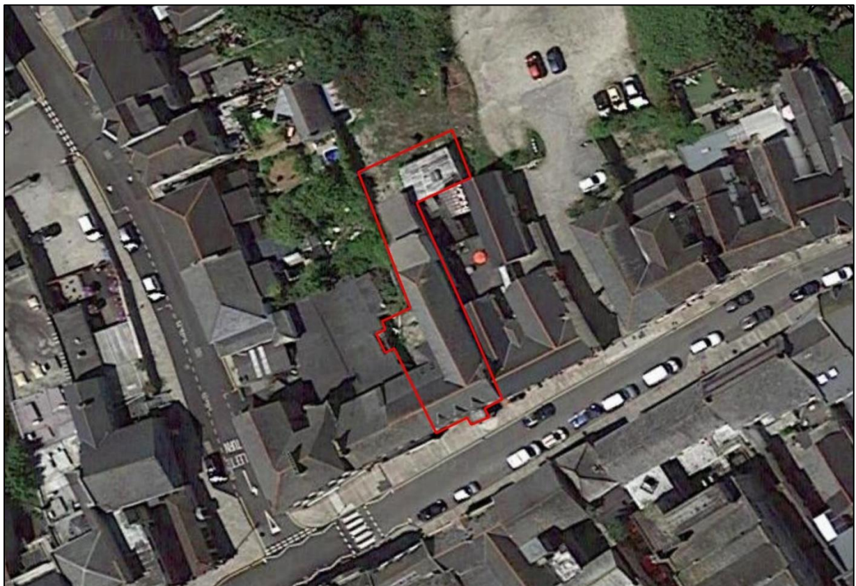
FIGURE 6: THE SITE AS IT STANDS TODAY (GOOGLE MAPS 2023©).
