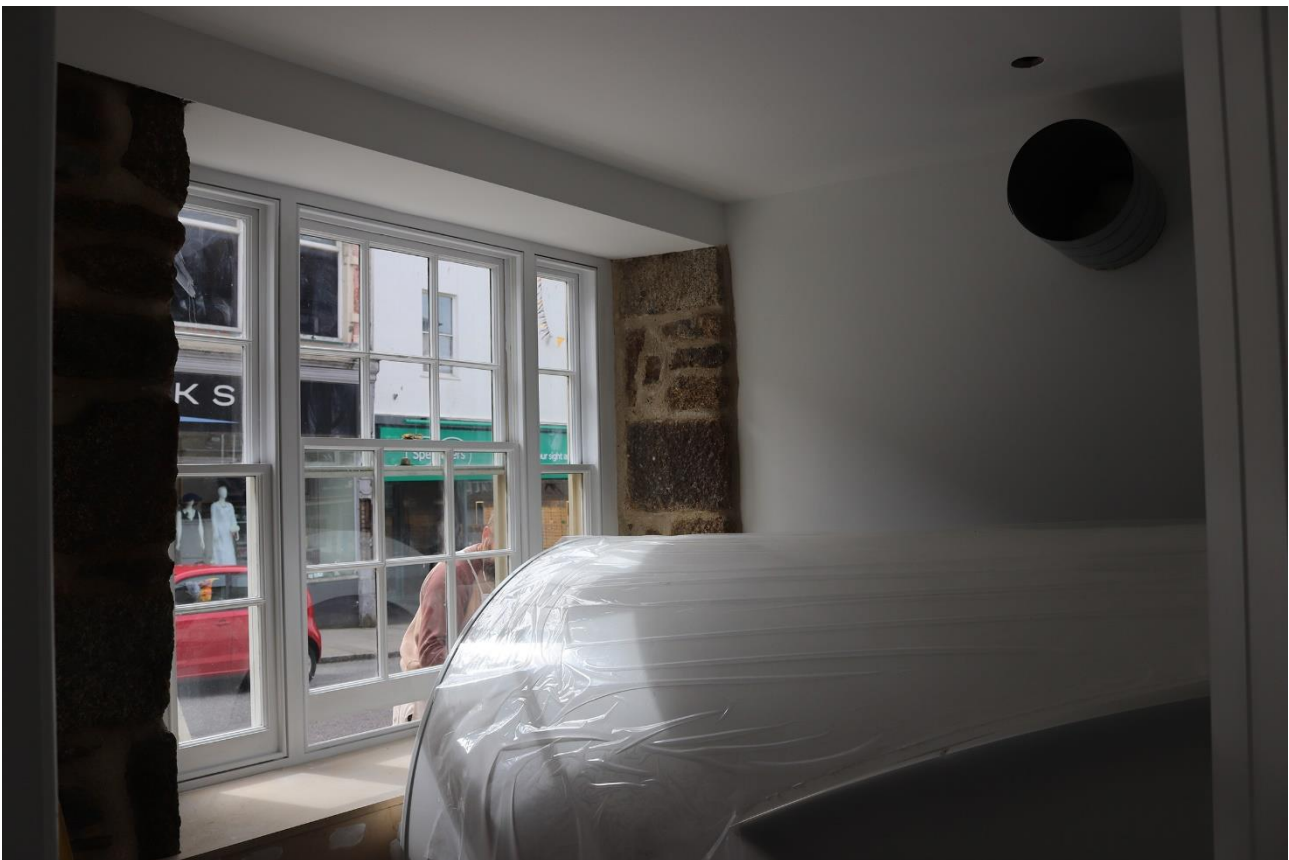
24. CUBICLE TO THE WEST SIDE OF GF SPACE SHOWING SOME EXPOSED STONEMWORK.
