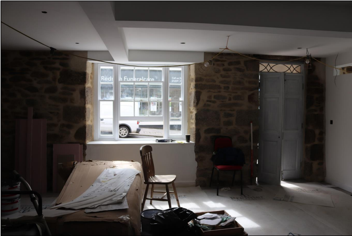
23. GF FRONT, REPLACEMENT TRI-PARTITE. FROM THE NORTH WITH 1M SCALES.
