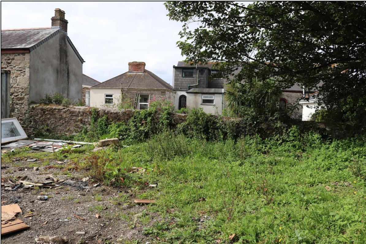
30. THE SURVIVING COMPOUND WALL TO THE EAST SIDE. FROM THE WEST.
