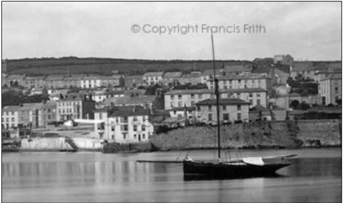
FIGURE 17: EXTRACT FROM A PHOTOGRAPH TAKEN FROM FLUSHING IN C.1876; THE HOTEL VIEWED FROM THE NORTH-EAST (© FRANCIS FRITH COLLECTION). IN THIS PHOTOGRAPH BLOCK C IS ONLY A SINGLE-STOREY STRUCTURE, AND BLOCK E HAS YET TO BE RAISED TO FOUR STOREYS. BLOCK D PRESENTS AS A CLASSIC LATE REGENCY GENTLEMAN'S RESIDENCE.
