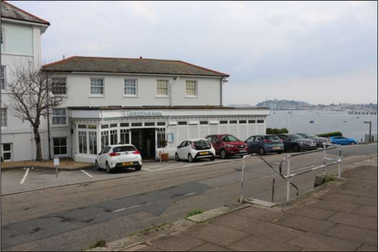
19. THE WEST ELEVATION OF BLOCK F; VIEWED FROM THE WEST.
