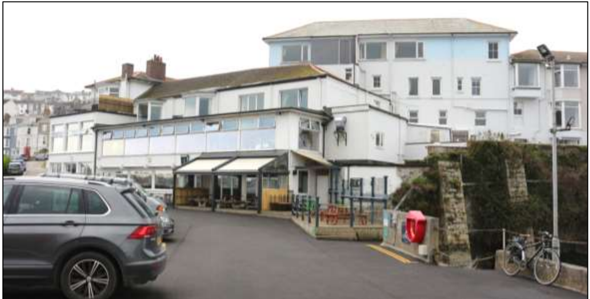
FIGURE 31: THE EAST ELEVATION OF THE SOUTHERN PART OF THE HOTEL; VIEWED FROM THE EAST.
