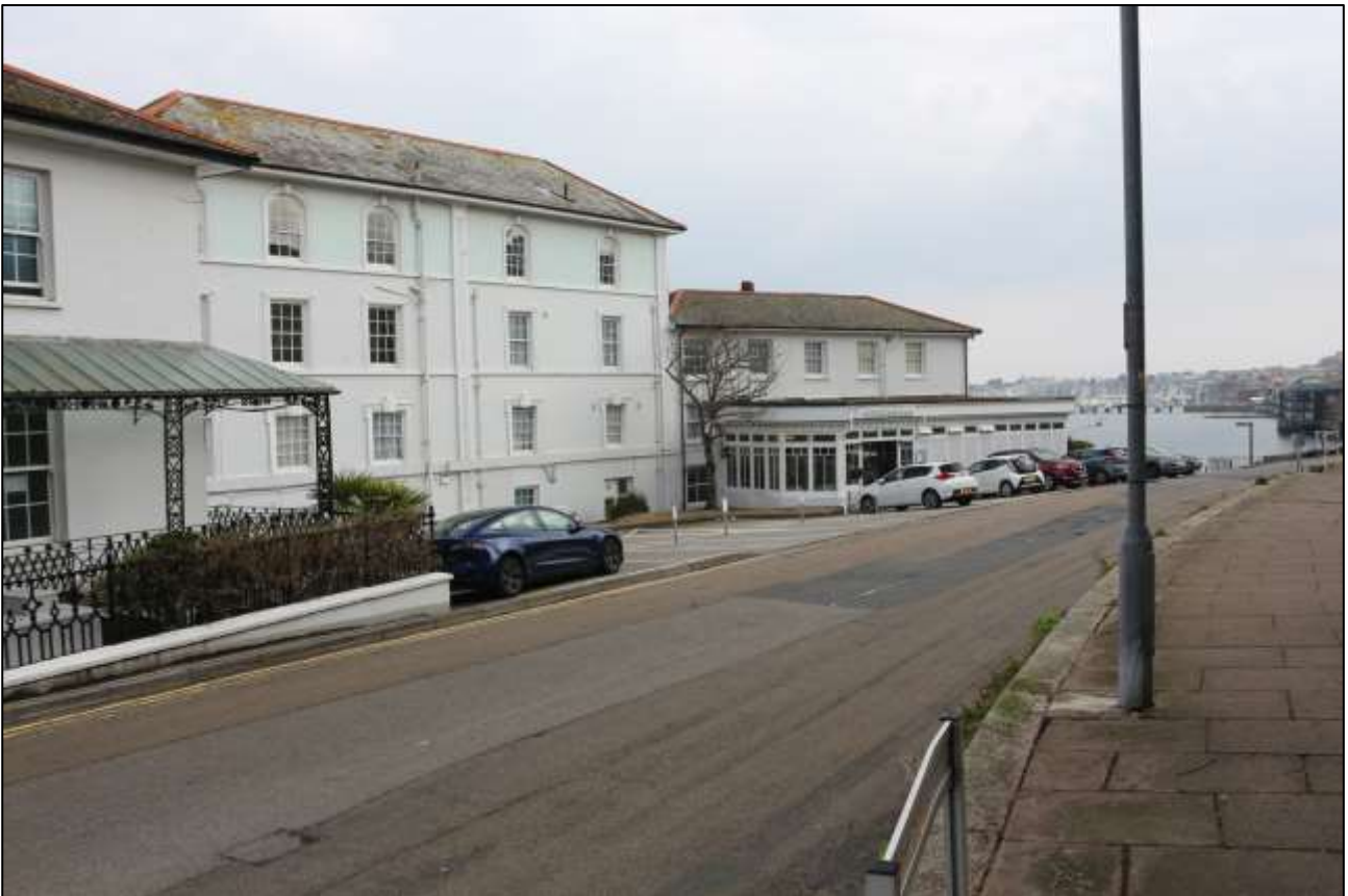
24. THE WEST ELEVATIONS OF BLOCKS D (LEFT), E (CENTRE-LEFT) AND F (RIGHT); VIEWED FROM THE NORTH-WEST.
