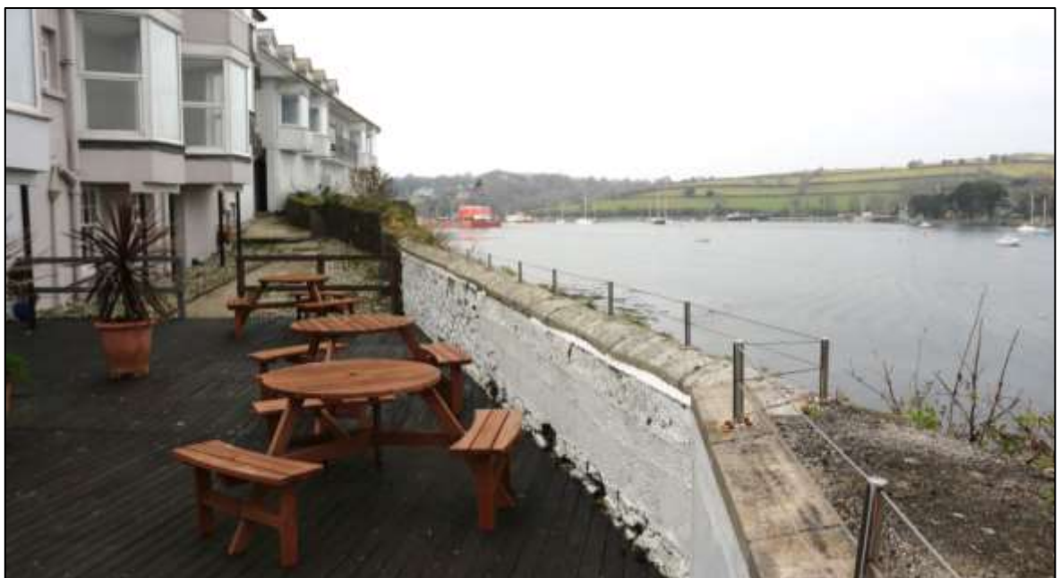
FIGURE 30: THE NARROW TERRACE BETWEEN THE HOTEL AND THE DROP TO THE FORESHORE; VIEWED FROM THE SOUTH-EAST.
