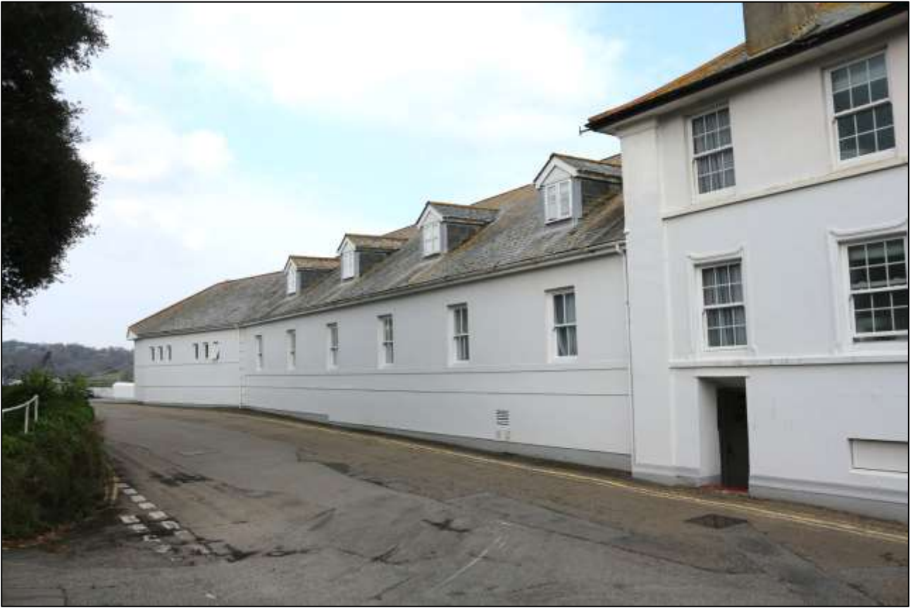
25. THE WEST ELEVATIONS OF BLOCKS A AND B (LEFT) AND BLOCK C (RIGHT); VIEWED FROM THE SOUTH-WEST.
