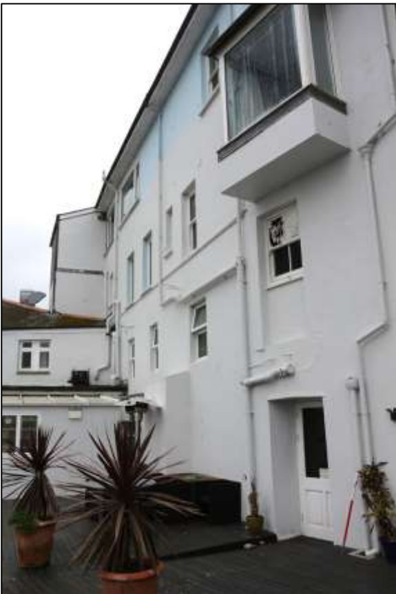
10. THE EAST ELEVATION OF BLOCK E; VIEWED FROM THE NORTH.
