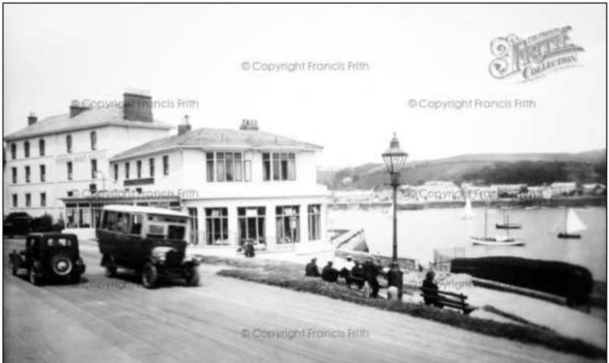
FIGURE 26: THE HOTEL IN 1933; VIEWED FROM THE SOUTH. THE NEW PORCH HAS BEEN EXTENDED ALONG THE WEST SIDE OF BLOCK F, AND THE SEMI-CIRCULAR EXTENSION ADDED TO THE SOUTH SIDE OF BLOCK F (© FRANCIS FRITH COLLECTION).
