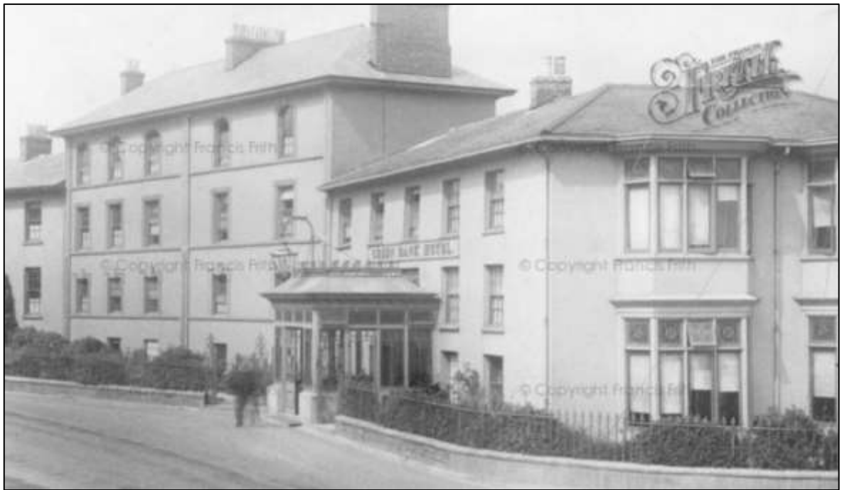
FIGURE 22: THE HOTEL IN 1904; VIEWED FROM THE SOUTH. THE PORCH ON THE WEST SIDE OF BLOCK F HAS GONE, REPLACED BY A LARGER EDWARDIAN TIMBER STRUCTURE WITH LANTERN (© FRANCIS FRITH COLLECTION).
