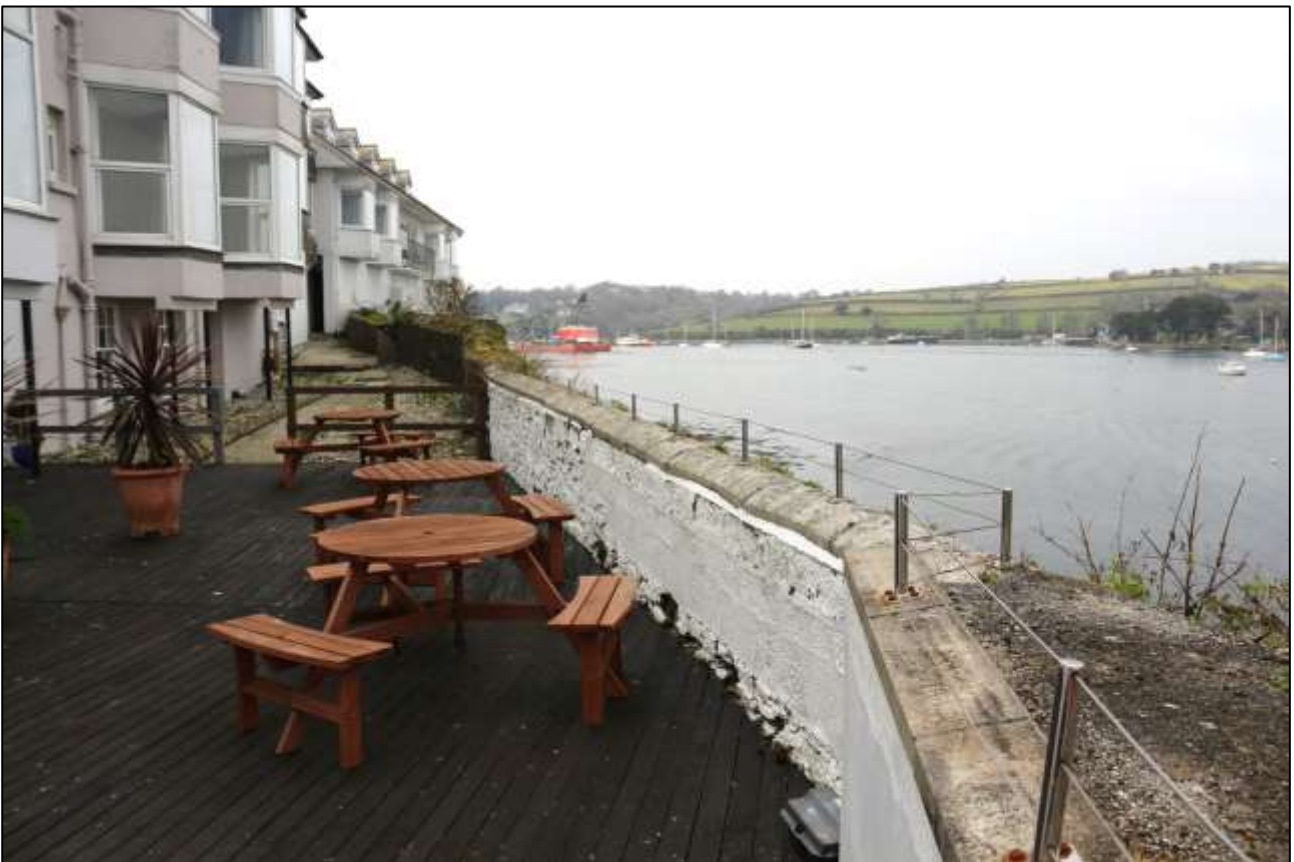
7. AREA 4, THE SOUTHERN TERRACE, SURFACE TREATMENTS AND WALL; VIEWED FROM THE SOUTH-EAST.
