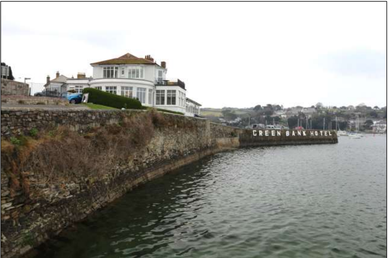
14. THE VIEW BACK TO THE QUAY FROM THE GREEN BANK GARDENS; VIEWED FROM THE SOUTH-WEST.
