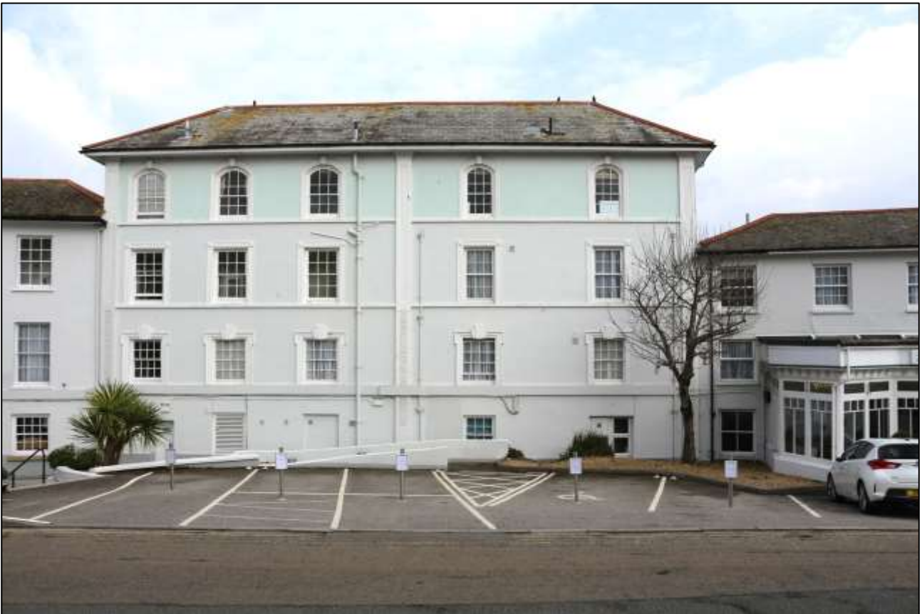
20. THE WEST ELEVATION OF BLOCK E; VIEWED FROM THE WEST.
