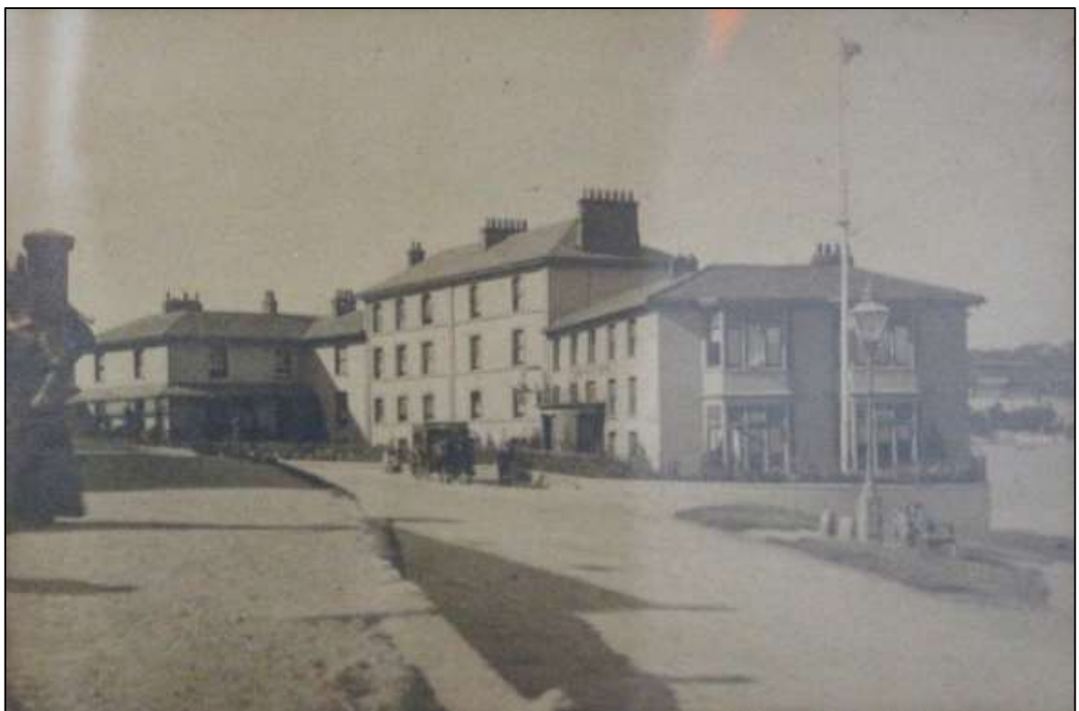
FIGURE 20: THE HOTEL IN 1897; VIEWED FROM THE SOUTH (IMAGE FROM THE HOTEL COLLECTION). THE SHALLOW BAYS WITH SASHES ON THE SOUTH SIDE OF BLOCK F HAVE GONE, REPLACED BY CHUNKY LATE VICTORIAN CANTED BAY WINDOWS.
