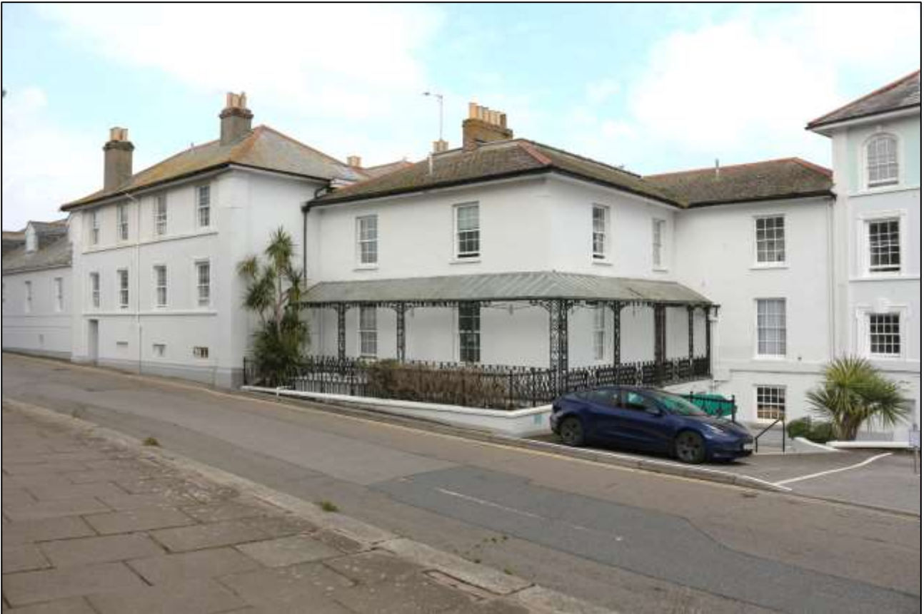
21. THE WEST AND SOUTH ELEVATION OF BLOCKS C (LEFT) AND D (CENTRE); VIEWED FROM THE SOUTH-WEST.
