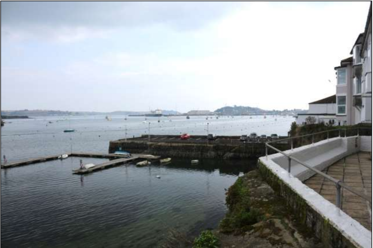
4. VIEW FROM THE AREA 1, NORTHERN TERRACE, TOWARDS PENDENNIS AND FALMOUTH DOCKS; VIEWED FROM THE NORTH-WEST.
