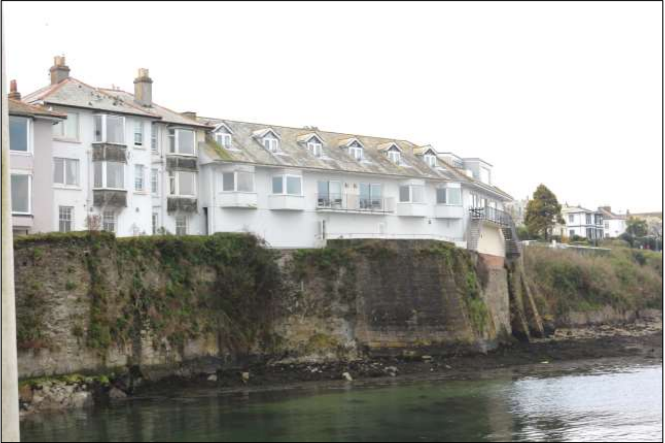
11. THE EAST ELEVATION OF BLOCKS A AND B (CENTRE) AND C (LEFT); VIEWED FROM THE ESE.
