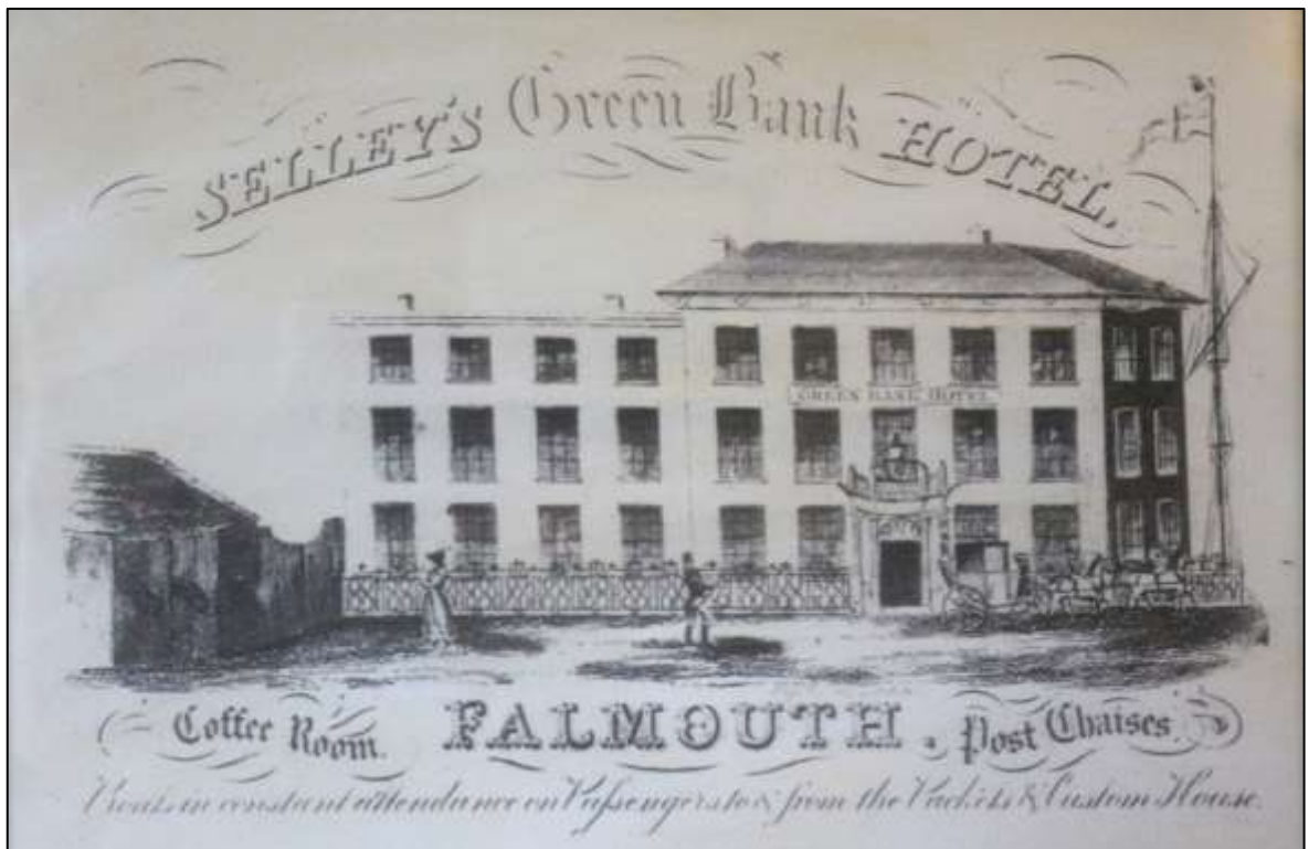
FIGURE 16: ANOTHER EARLY 19 TH CENTURY FLYER FOR SELLEY'S GREEN BANK HOTEL . THIS IMAGE MORE CLEARLY SHOWS THE RELATIVE HEIGHT OF BLOCKS E AND F. IT MUST PREDATE C.1830 AS BLOCK D AS A LOW BUILDING WITH GATES IS SHOWN INSTEAD (ON THE LEFT). AN ELABORATE PILLARED PORCH IS SHOWN ADORNING THE FRONT OF BLOCK; DETAIL OF THE PORCH WOULD SUGGEST A REGENCY DATE. THIS IMAGE SHOWS THREE WINDOWS IN THE SOUTH WALL, BUT THE PREVIOUS FLYER AND SUBSEQUENT PHOTOGRAPHS ONLY SHOW TWO (IMAGE FROM THE HOTEL COLLECTION).
