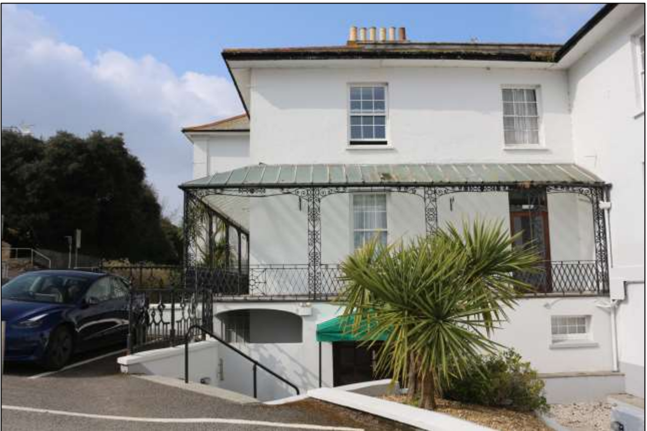
22. THE SOUTH ELEVATION OF BLOCK D; VIEWED FROM THE SOUTH.
