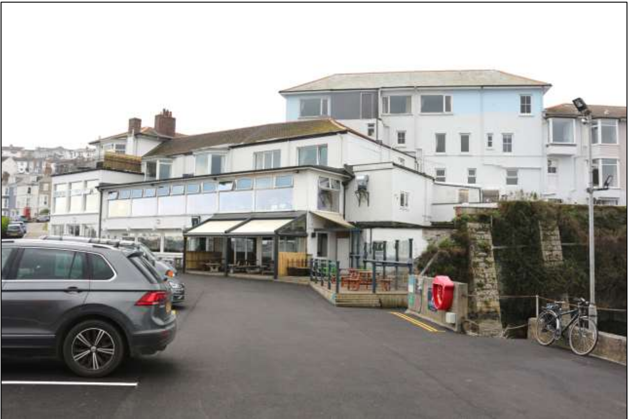
12. THE EAST ELEVATIONS OF BLOCKS E (RIGHT OF CENTRE), G, H, AND I; VIEWED FROM THE NORTH-EAST.
