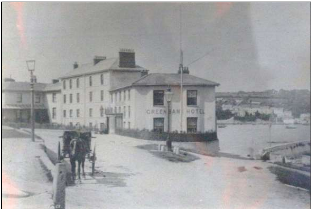
FIGURE 18: THE HOTEL IN 1885; VIEWED FROM THE SOUTH (IMAGE FROM THE HOTEL COLLECTION). BLOCK E HAS NOW BEEN RAISED TO FOUR STOREYS, AND THE SOUTH END OF BLOCK F SPORTS TWO SHALLOW BAYS WITH SINGLE SASH WINDOWS. THE WEST PORCH SHOWN ON THE EARLIER DRAWN FLYERS (CONTRAST THIS IMAGE WITH FIGURE 20, BELOW).
