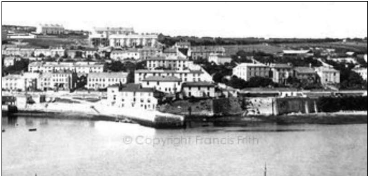
FIGURE 21: EXTRACT FROM A PHOTOGRAPH TAKEN FROM FLUSHING IN C.1895; THE HOTEL VIEWED FROM THE NORTH-EAST (© FRANCIS FRITH COLLECTION). IN THIS PHOTOGRAPH BLOCK C IS STILL SHOWN AS A SINGLE-STOREY STRUCTURE, BUT BLOCK E HAS BEEN RAISED TO FOUR STOREYS AND NOW DOMINATES BLOCK D.
