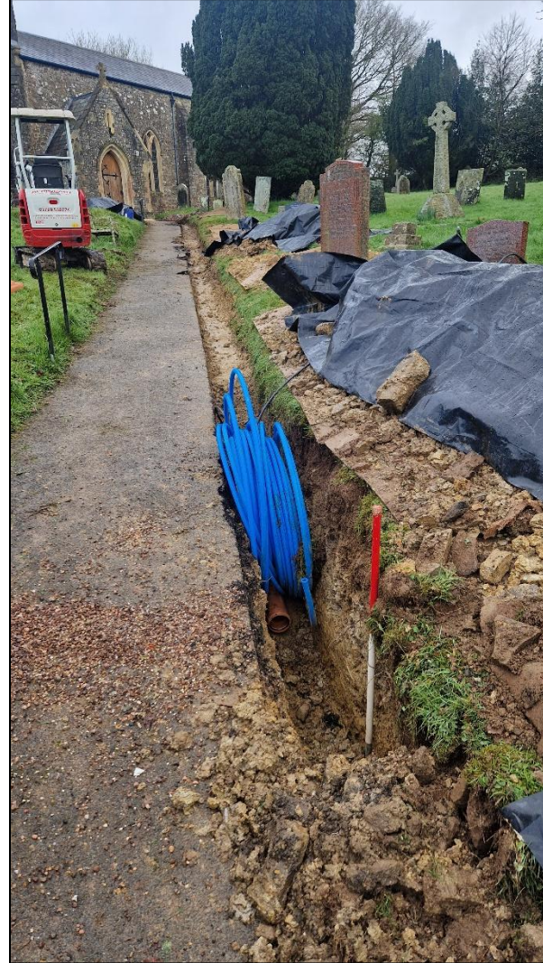
FIGURE 10: SOUTHERN END OF SERVICE TRENCH ALONG CHURCH PATH (SCALE 1M).
