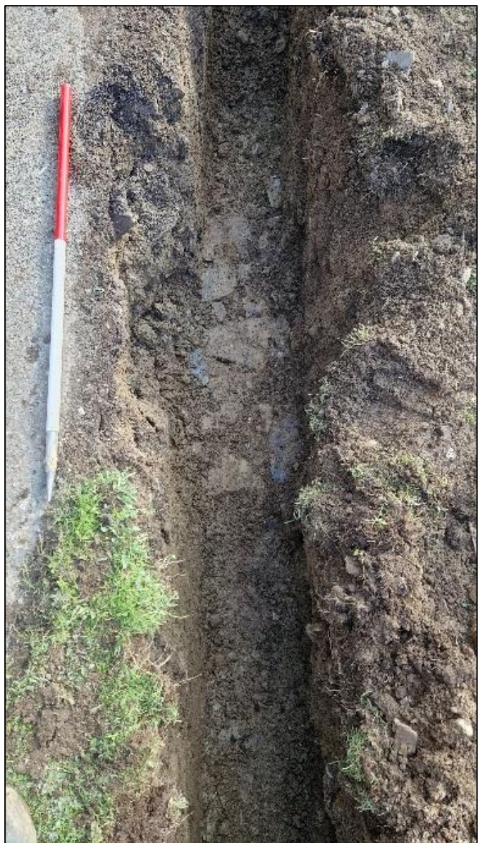
FIGURE 7: (LEFT) SHOT OF WALL FOOTINGS {103} VIEWED FROM NORTH (SCALE 1M).
